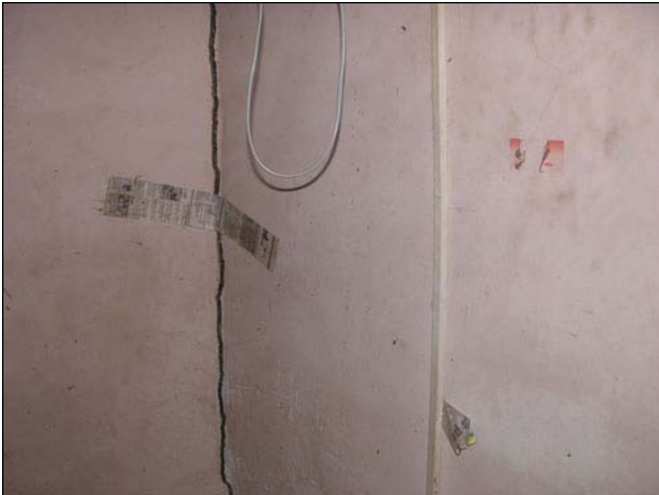
Figure 38 Masonry load bearing wall (S5-category)
