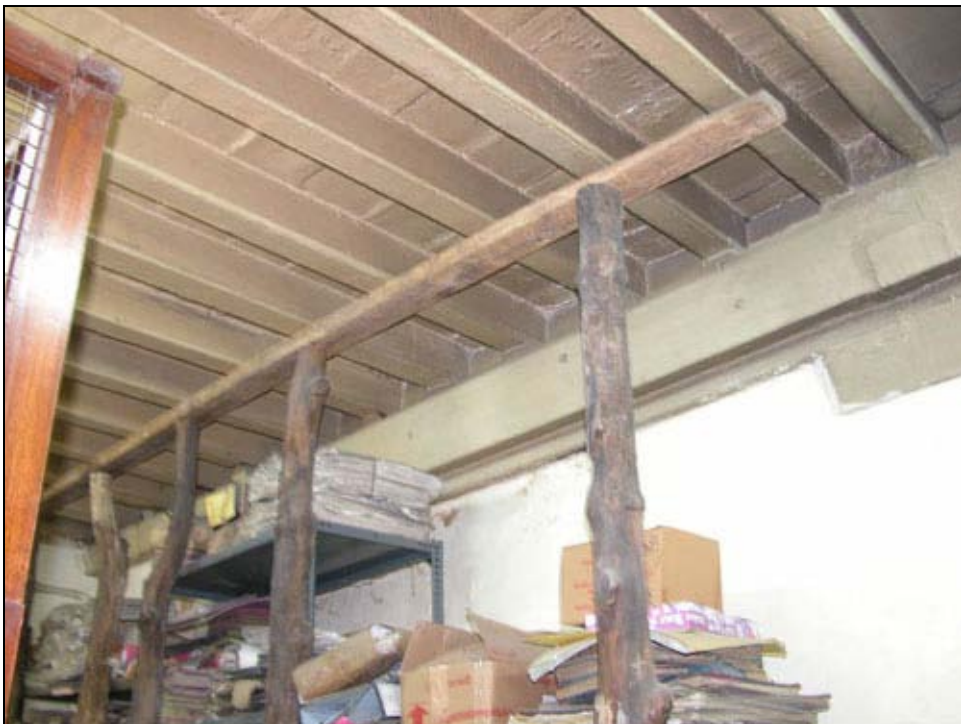
Figure 92 Timber joists (S3-category)
