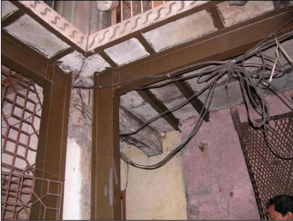
Figure 49 Steel column (S0-category)
