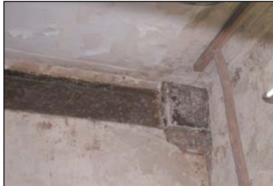
Figure 10 Steel beam on timber column
