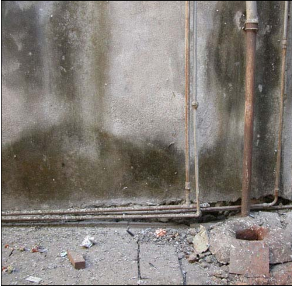
Figure 33 Masonry load bearing wall (S3-category)
