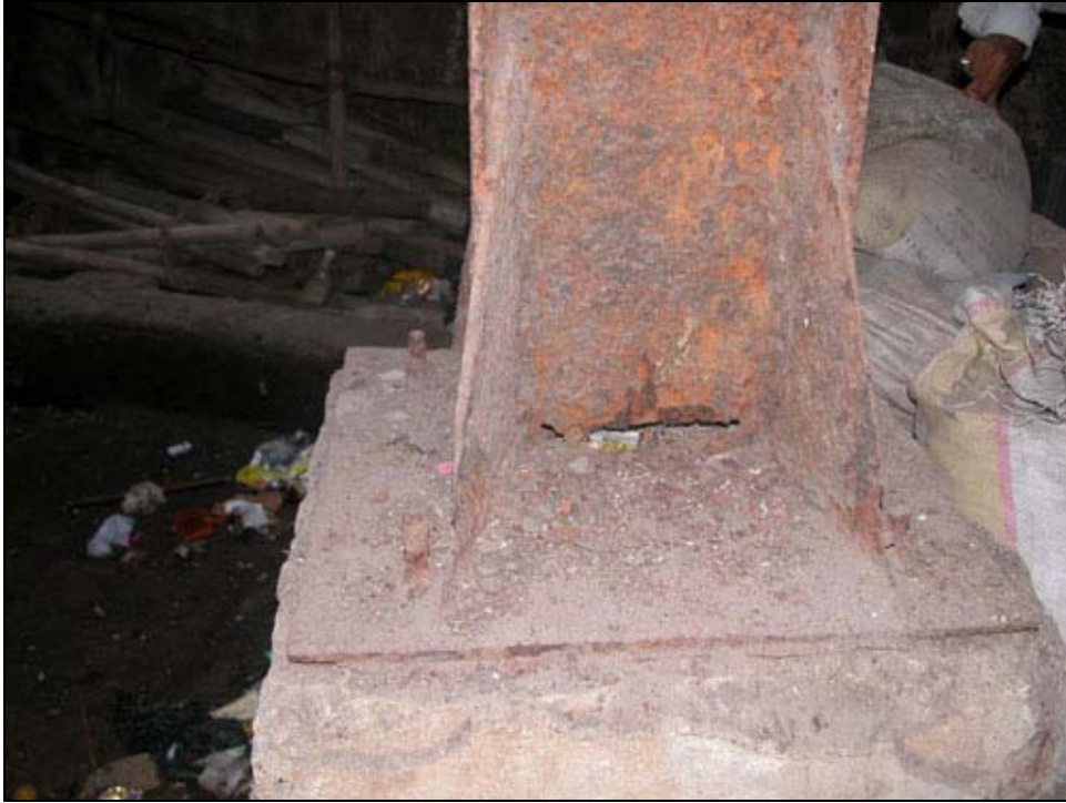
Figure 56 Steel column (S5-category)
