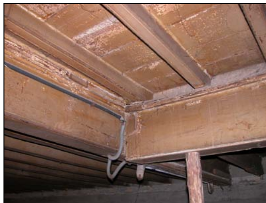
Figure 1 Timber flooring on timber joists
