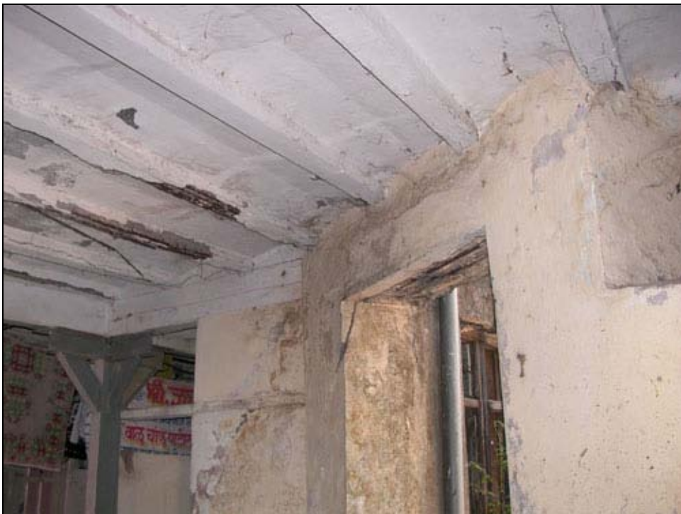
Figure 96 Cast stone slab (S1-category)
