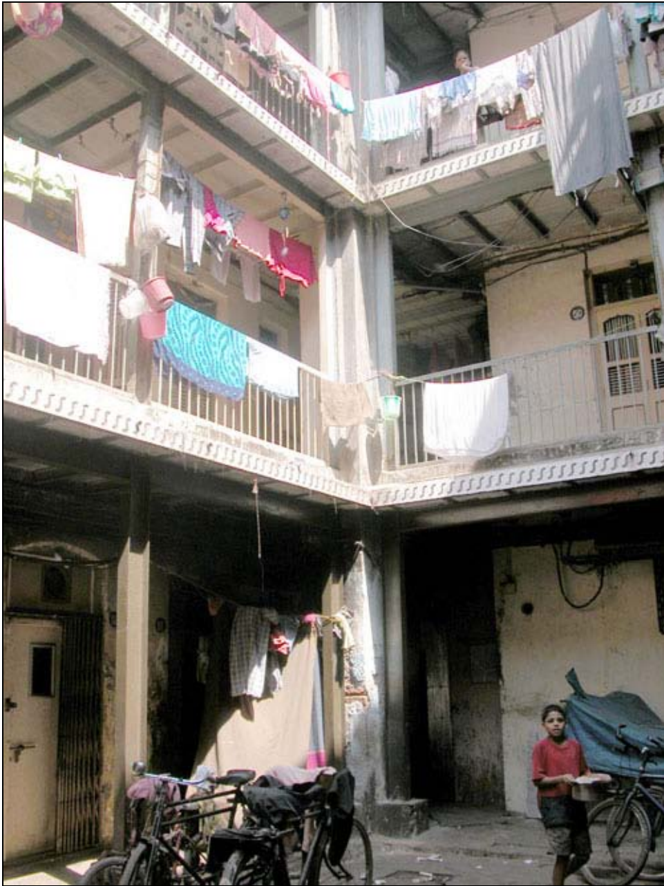
Figure 48 Steel column (S0-category)
