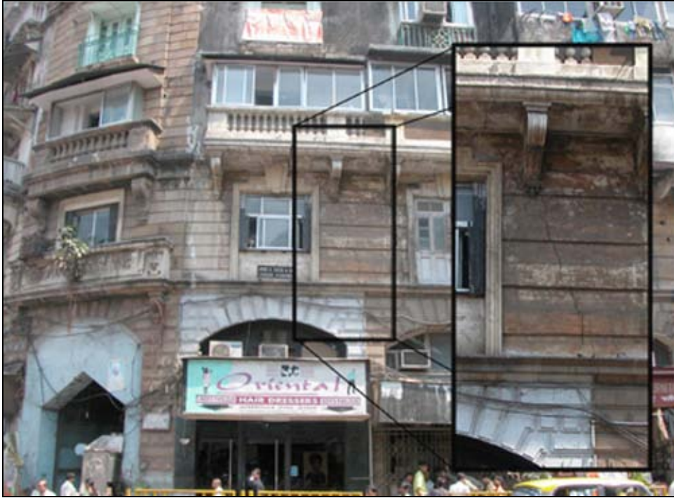
Figure 37 Masonry load bearing wall (S4-category)
