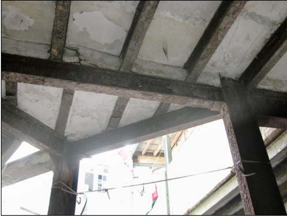
Figure 78 Steel beam (S3-category)
