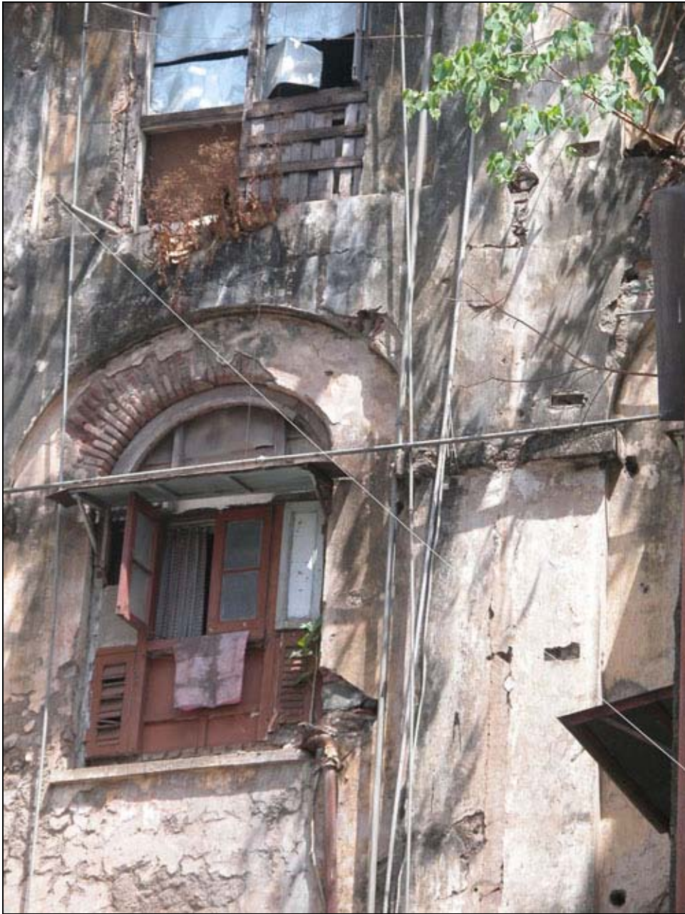
Figure 31 Masonry load bearing wall (S2-category)
