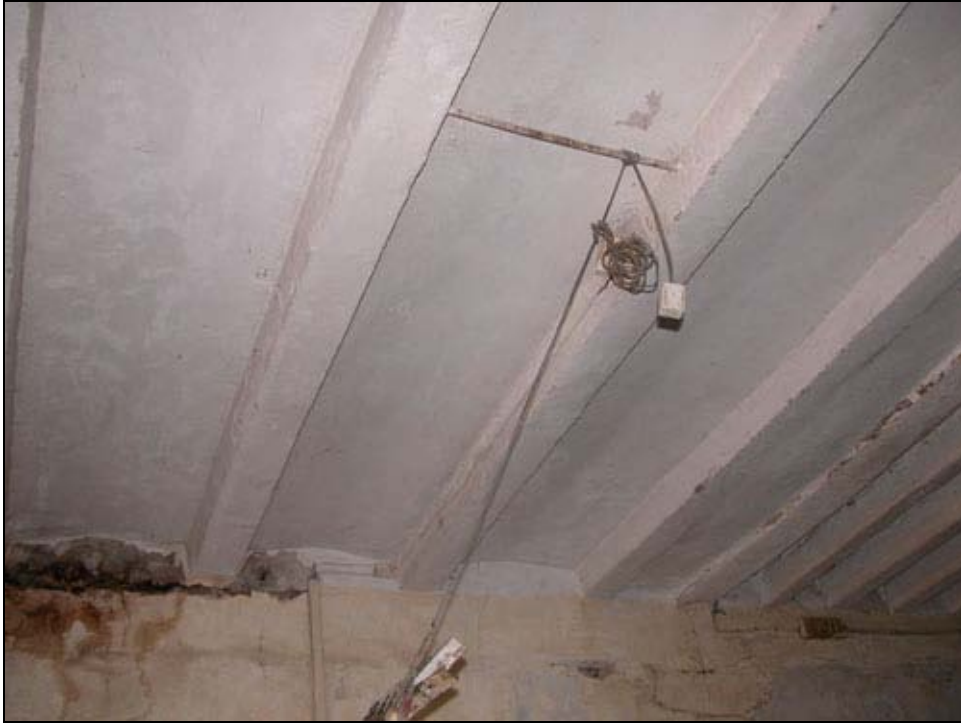
Figure 94 Cast stone slab (S0-category)
