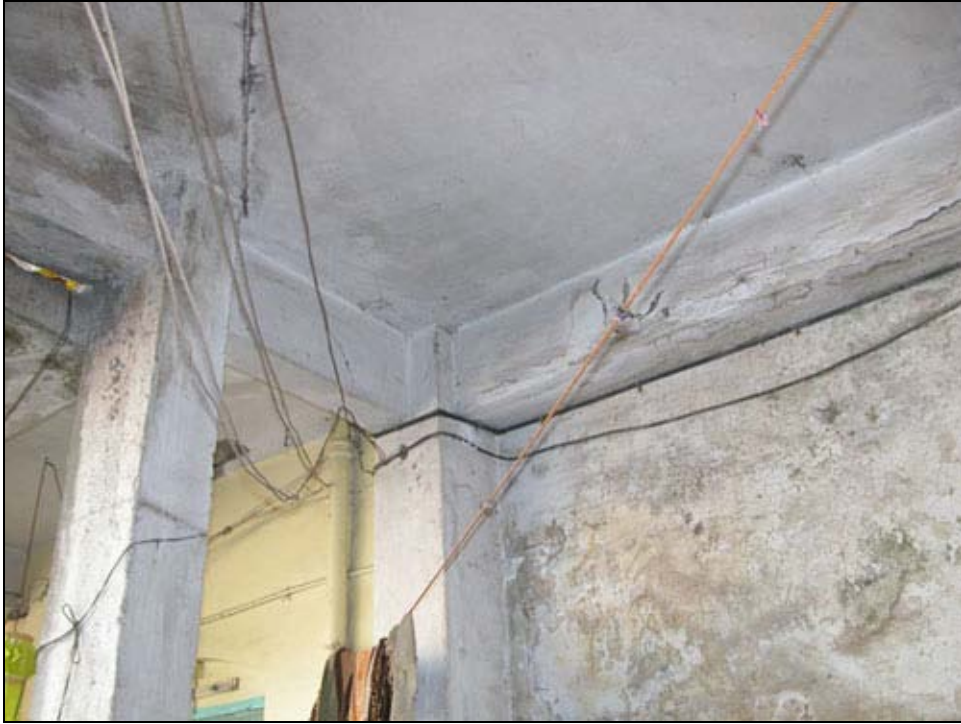
Figure 42 RCC column (S0-category)
