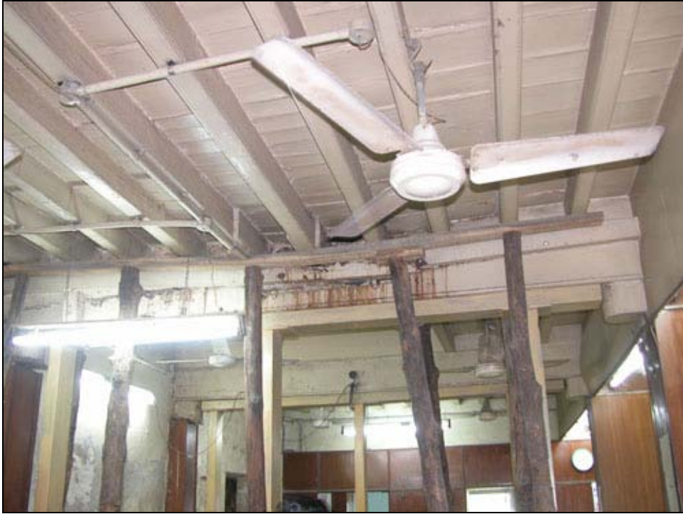
Figure 92 Timber joists (S3-category)
