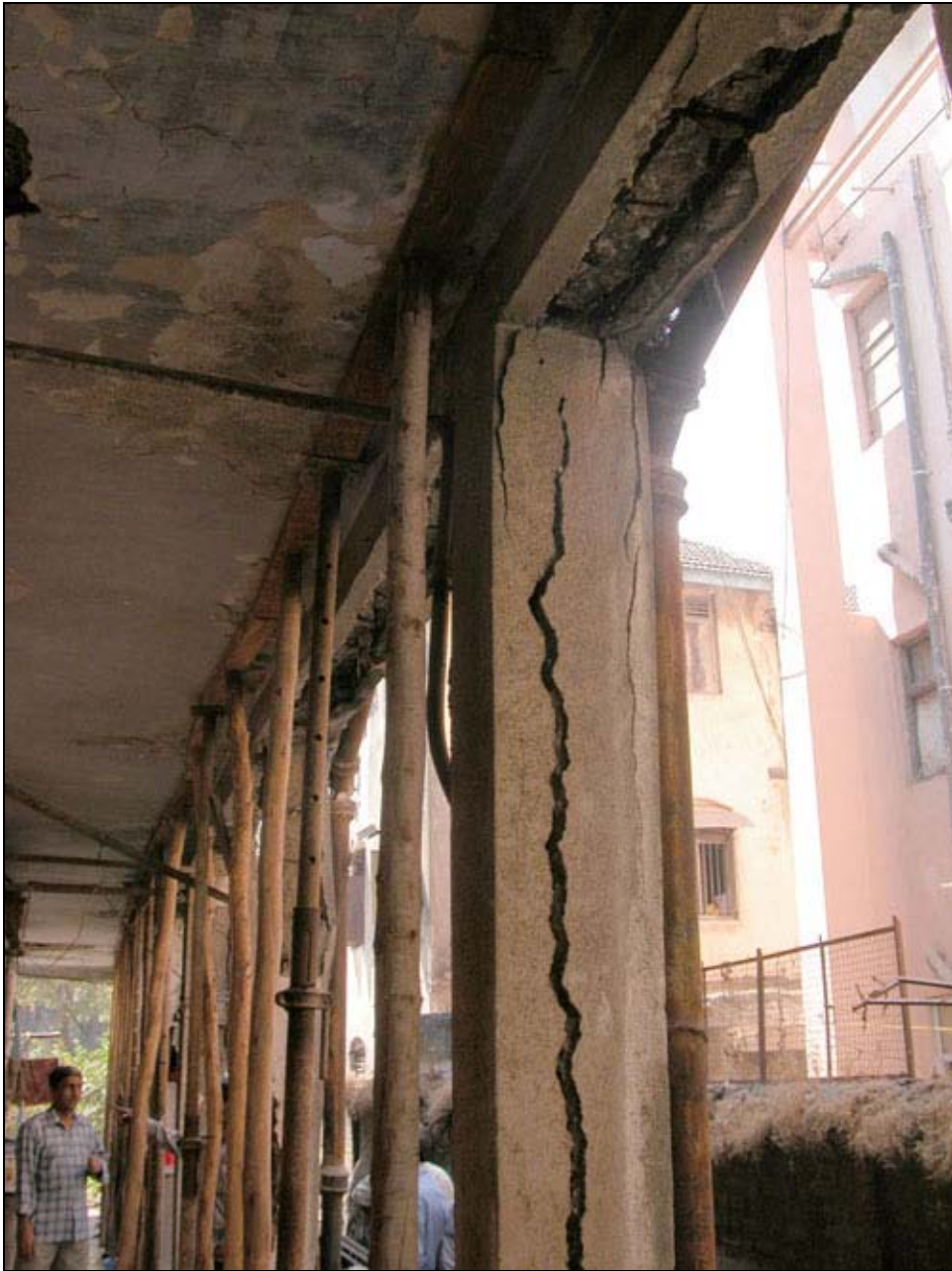
Figure 47 RCC column (S5-category)
