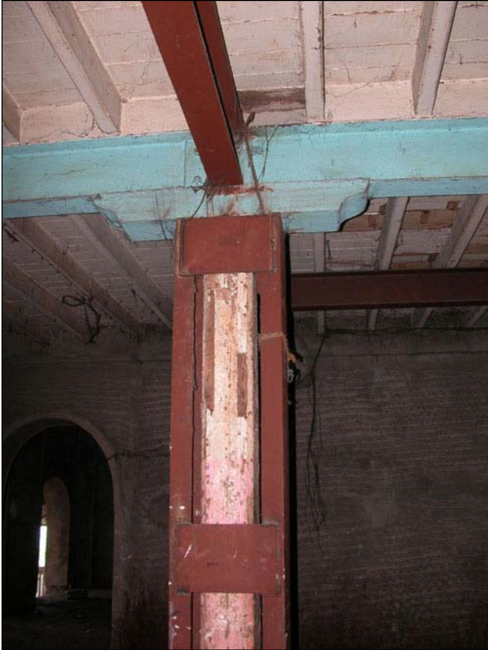
Figure 52 Steel column (S1-category)
