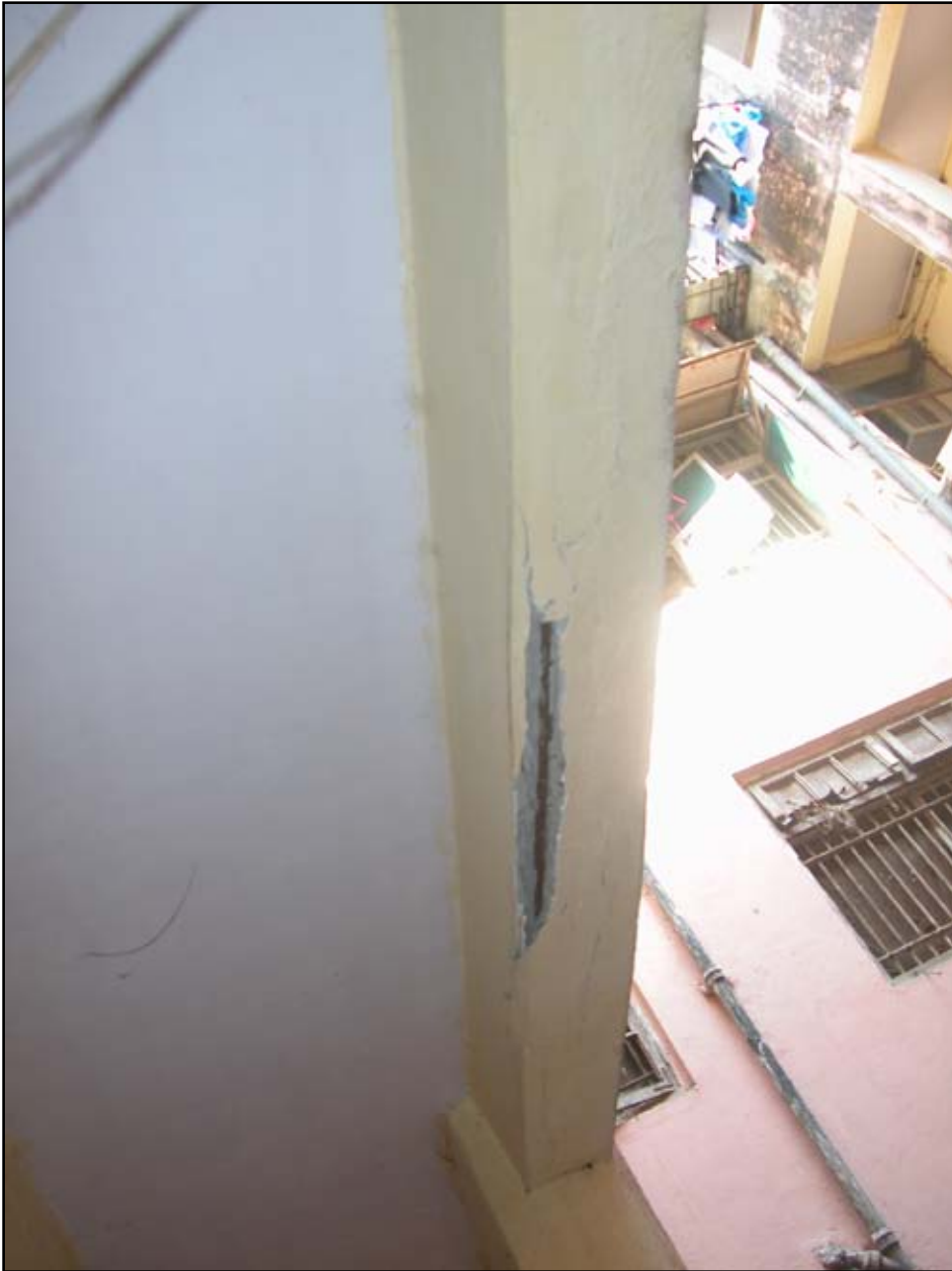
Figure 74 RCC beam (S3-category)
