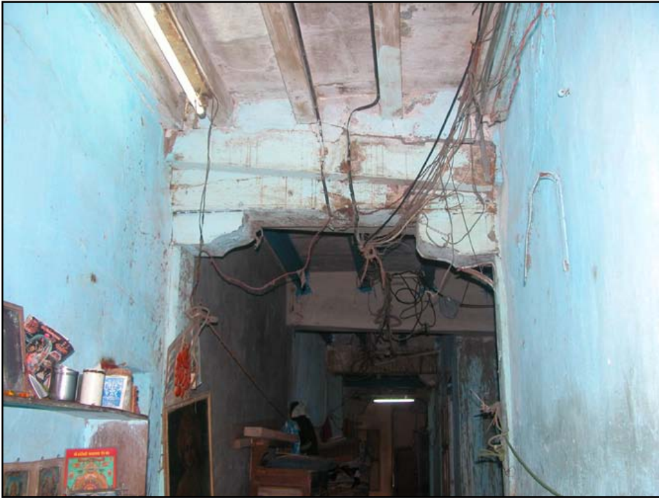
Figure 88 Timber beam (S4-category)
