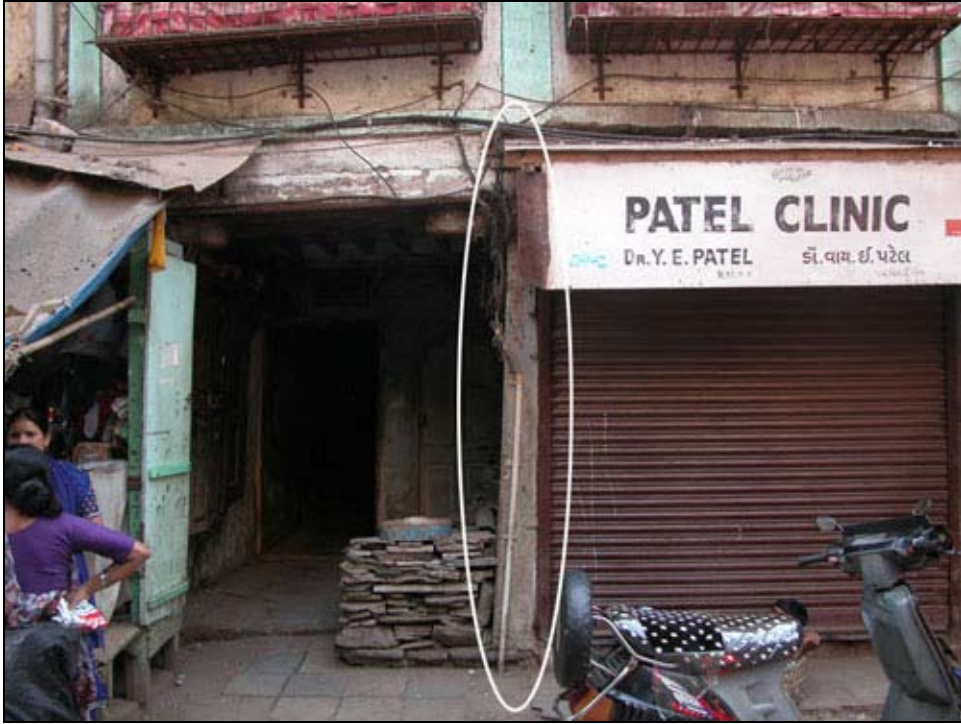
Figure 67 Timber column (S5-category)
