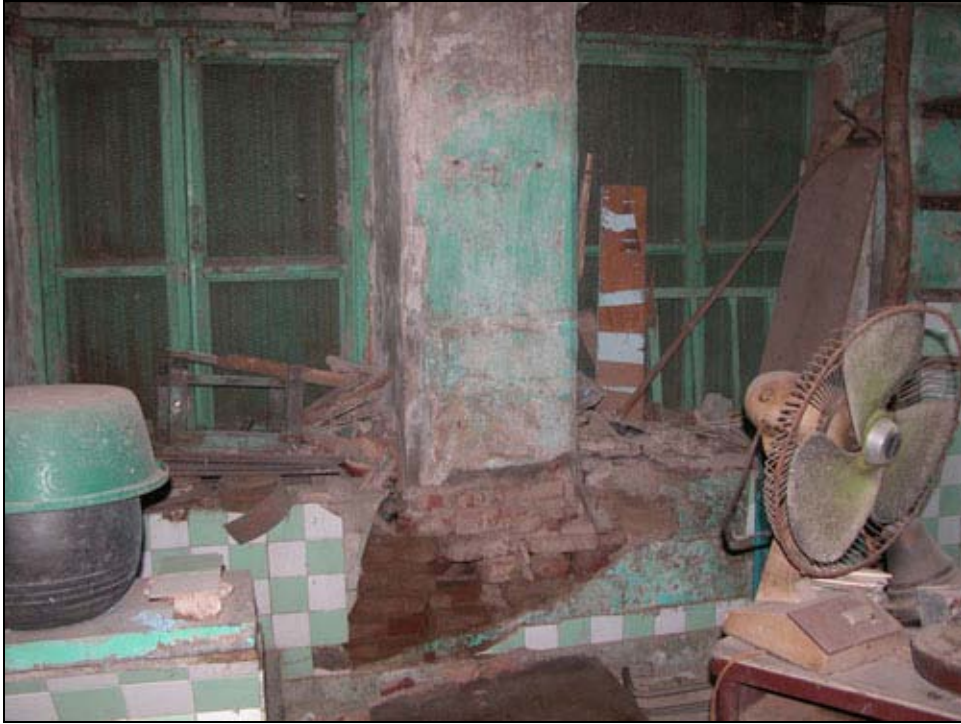
Figure 39 Masonry load bearing wall (S5-category)
