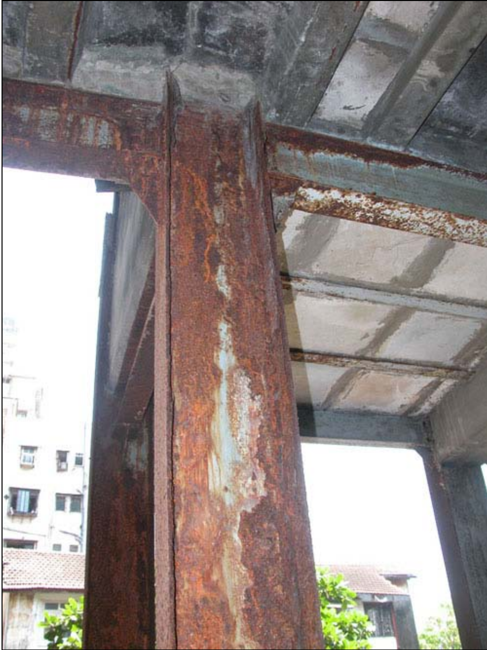
Figure 55 Steel column (S2-category)
