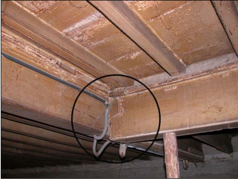
Figure 85 Timber beam (S3-category)
