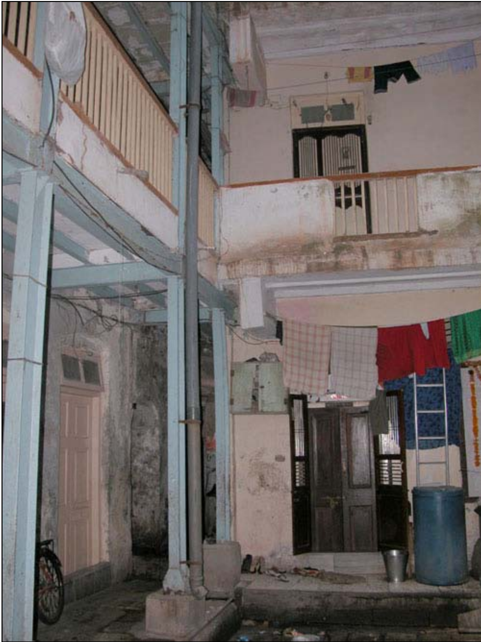
Figure 50 Steel column (S0-category)
