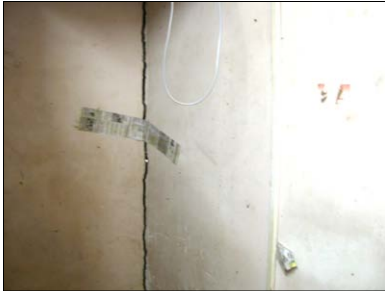
Figure 15 Separation of walls
