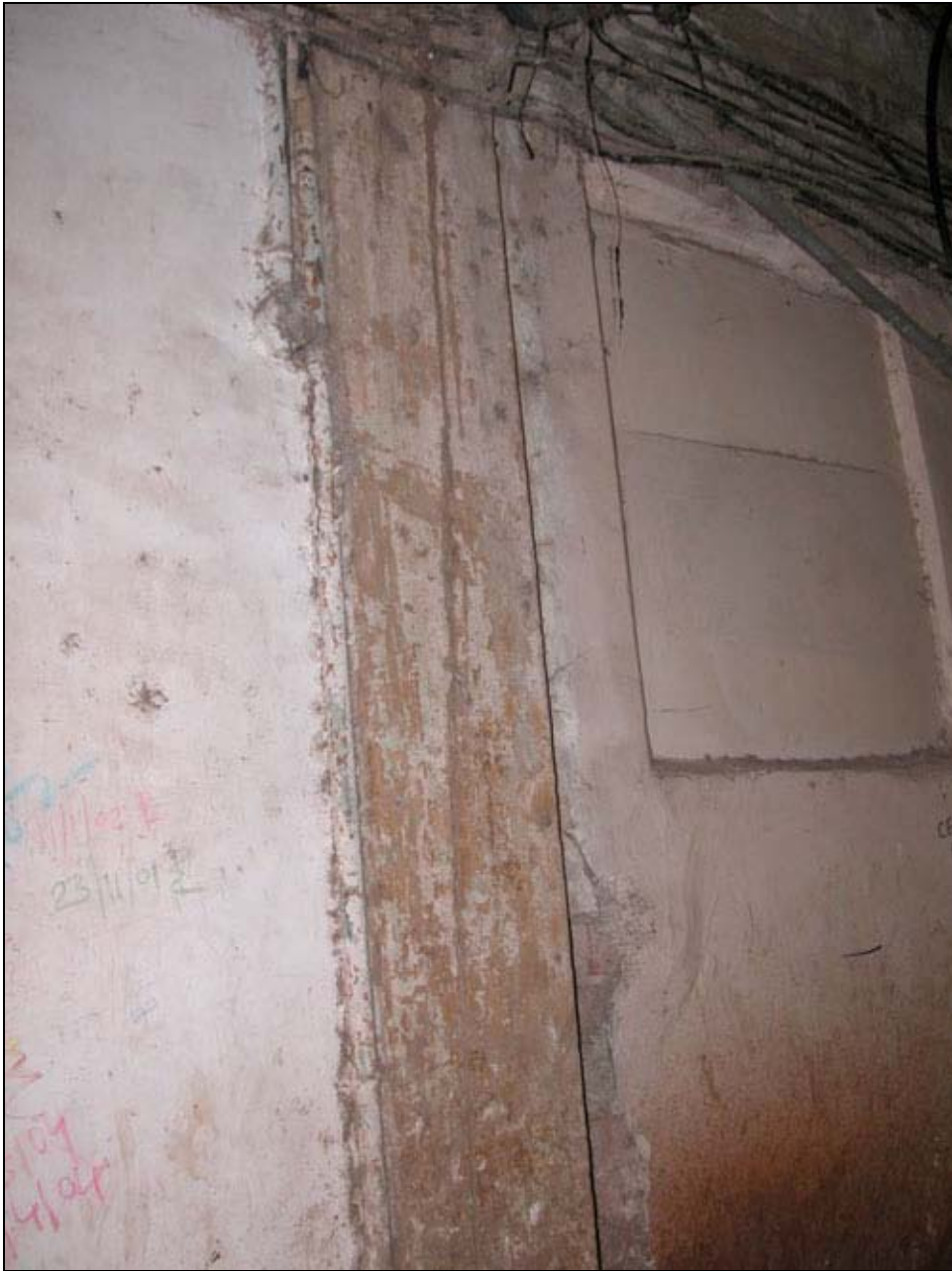
Figure 59 Timber column (S3-category)
