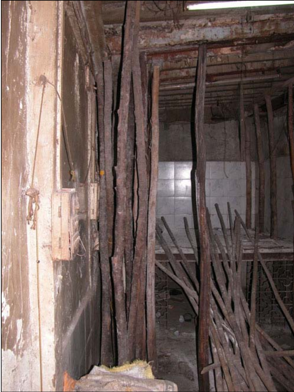
Figure 87 Timber beam (S4-category)
