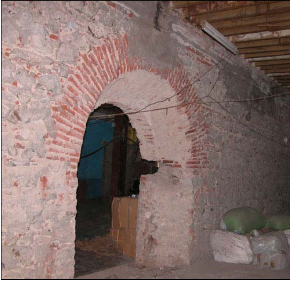
Figure 34 Masonry load bearing wall (S3-category)
