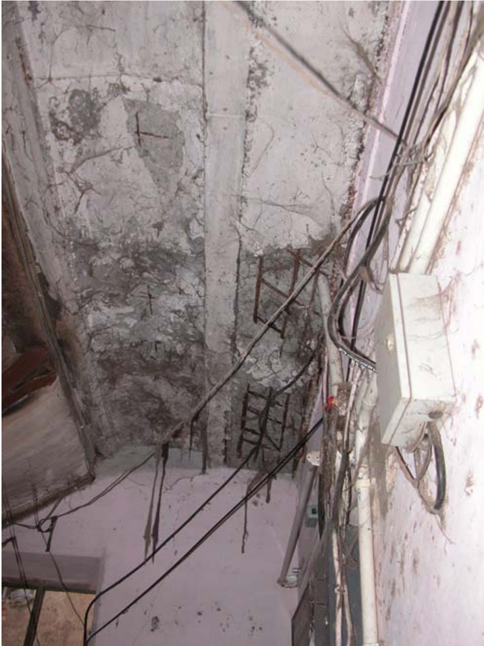
Figure 98 Cast stone slab (S3-category)
