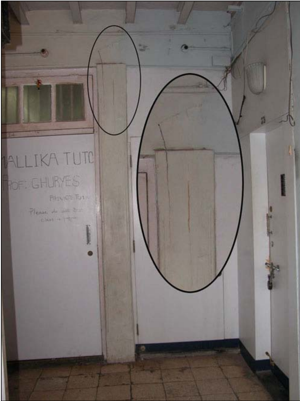
Figure 60 Timber column (S3-category)
