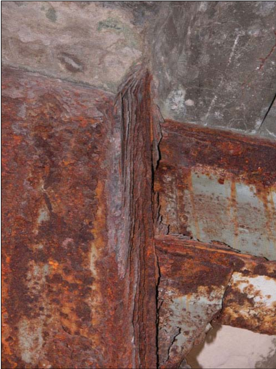
Figure 77 Steel beam-column junction (S3-category)
