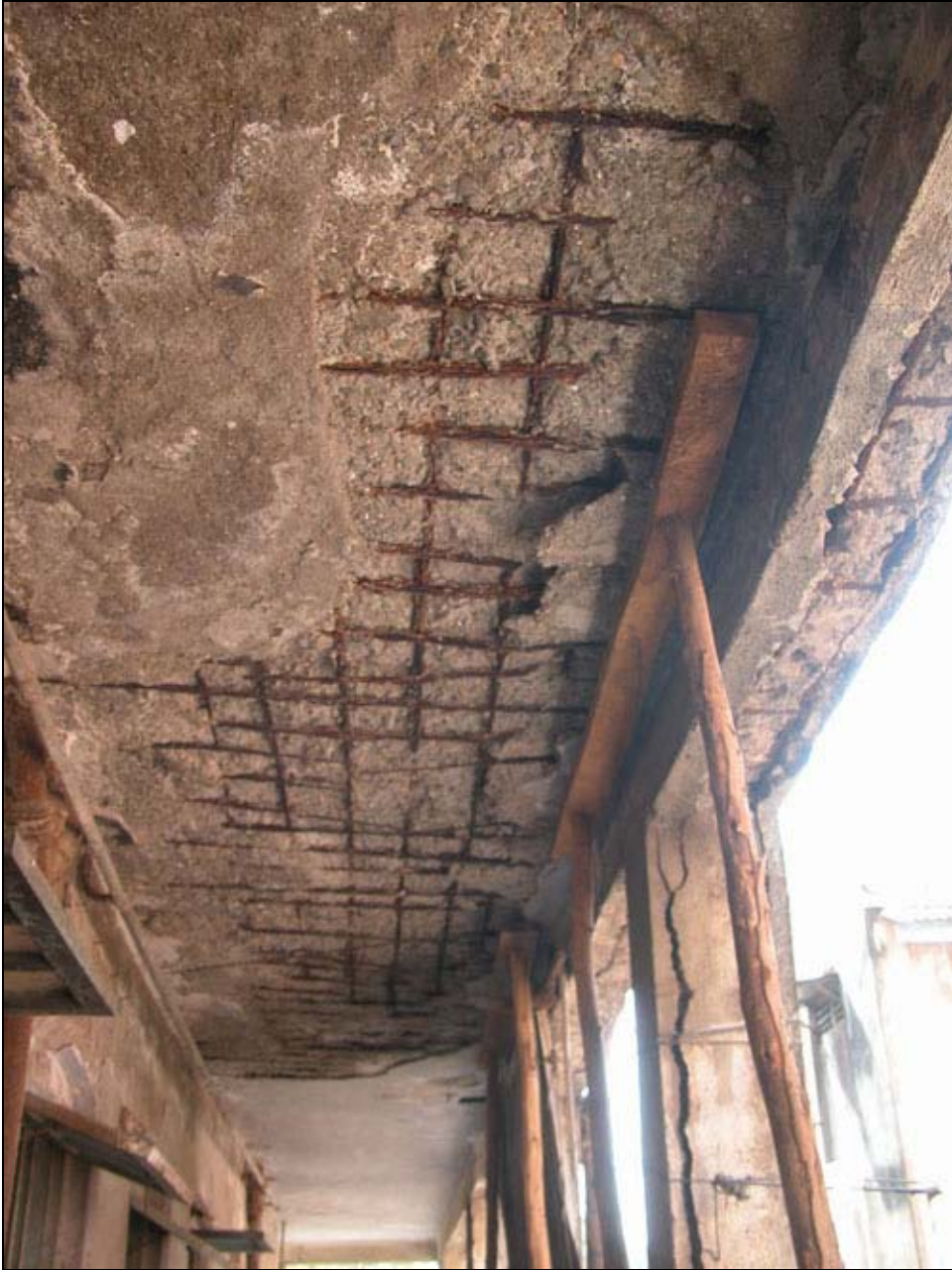
Figure 103 RCC slab (S4-category)
