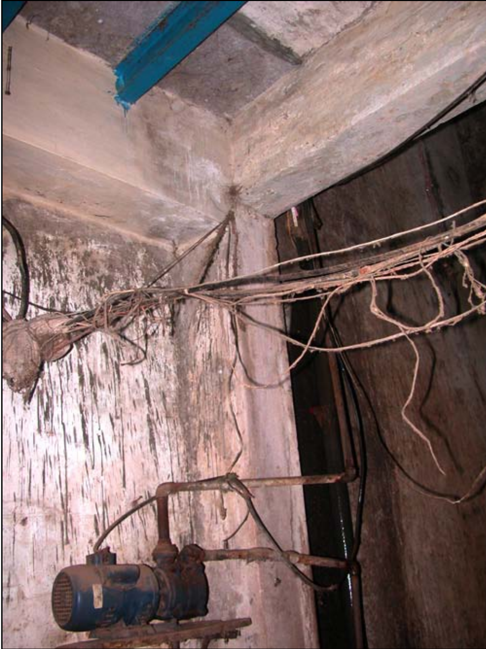
Figure 68 RCC beam (S1-category)
