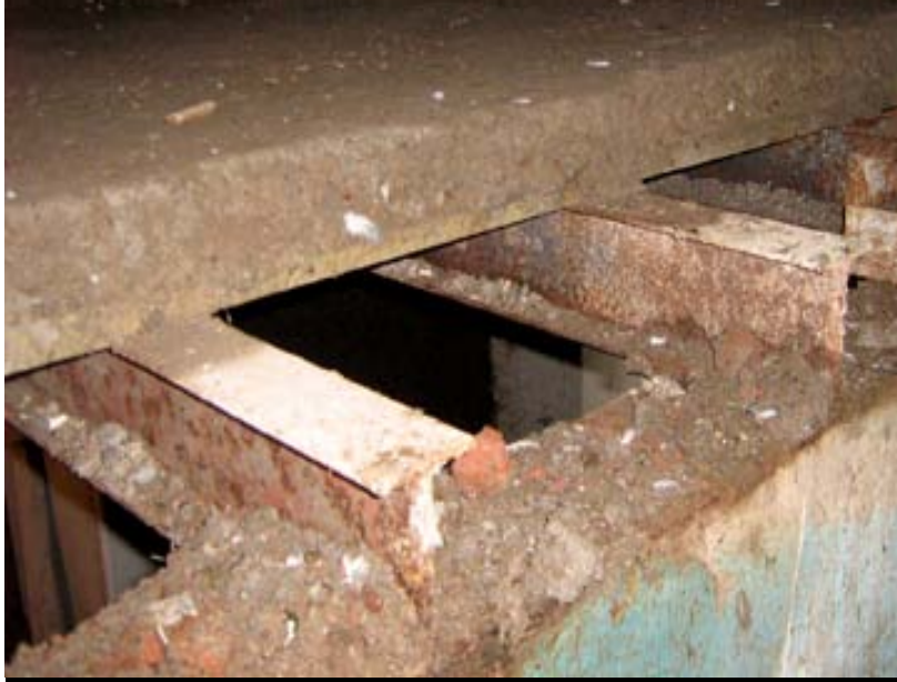
Figure 2 Ladi-Coba slab components
