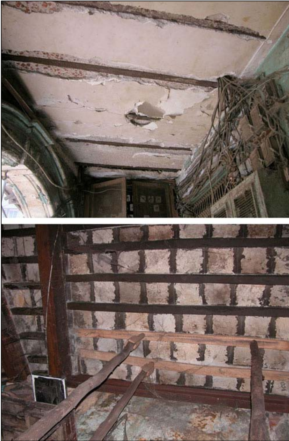
Figure 100 Ladicoba slab (S2-category)
