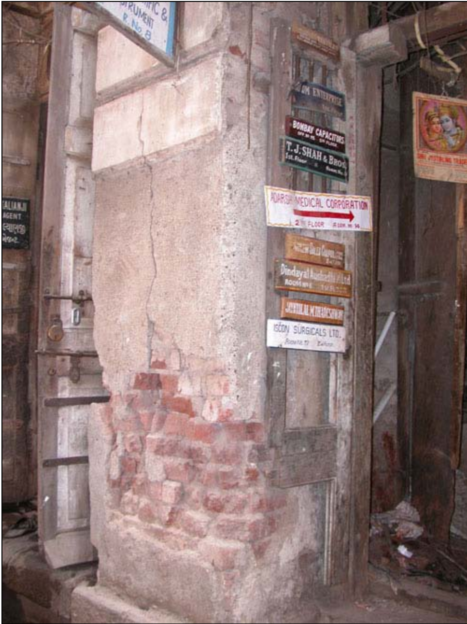
Figure 36 Masonry pier (S3-category)
