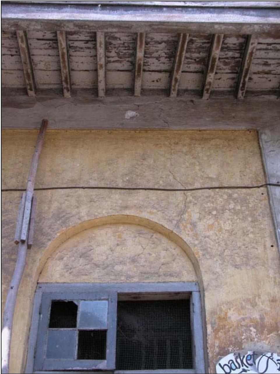
Figure 27 Masonry load bearing wall (S1-category)
