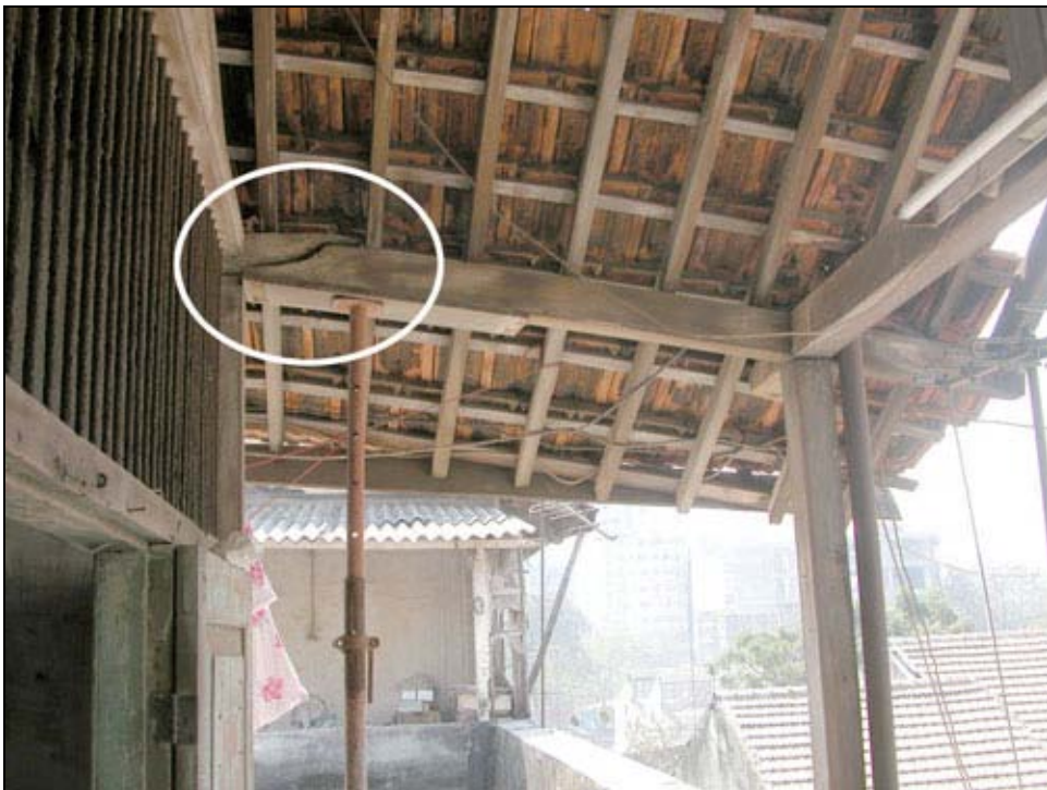
Figure 88 Timber beam (S4-category)
