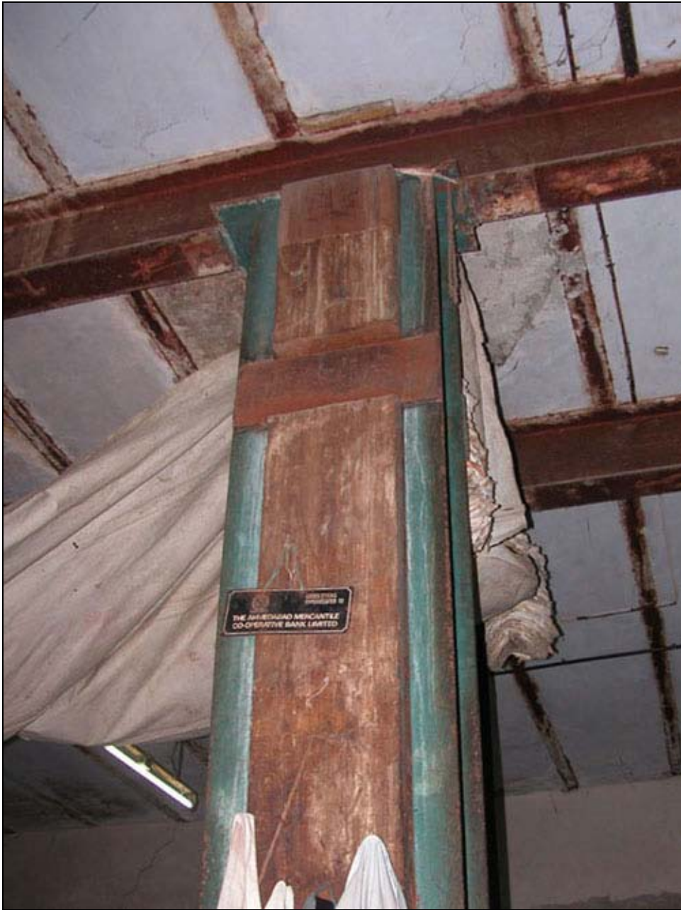
Figure 51 Steel column (S1-category)
