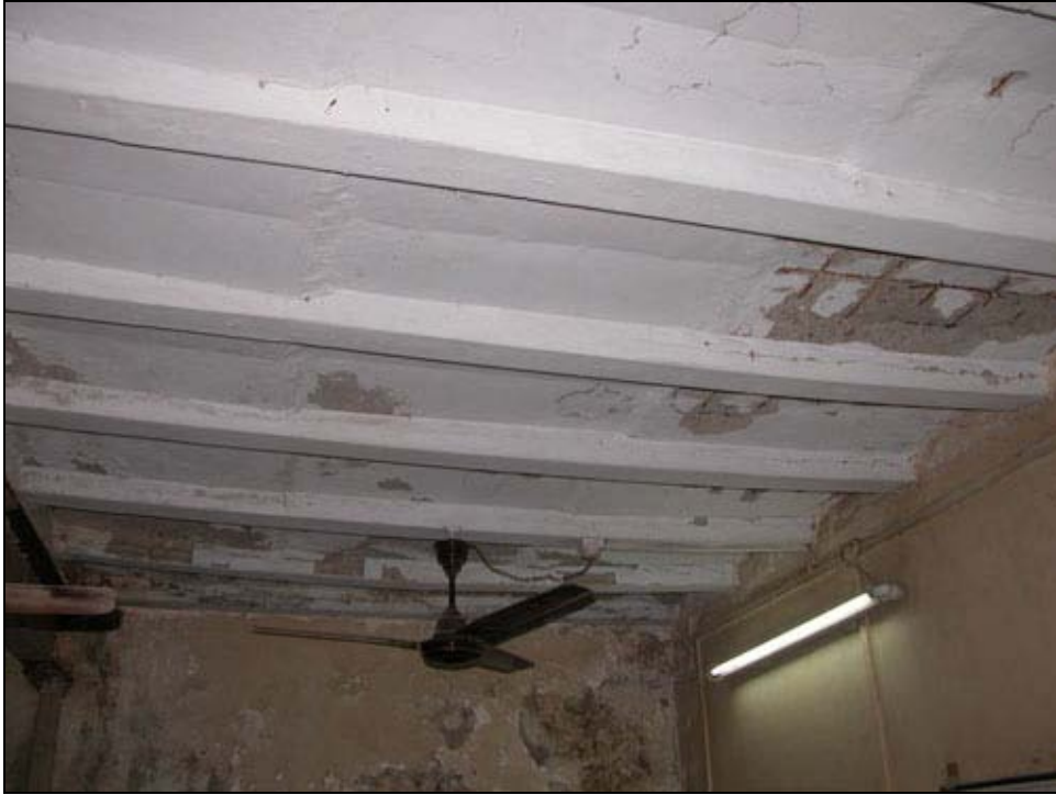
Figure 96 Cast stone slab (S1-category)
