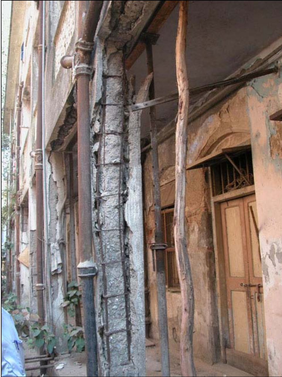
Figure 46 RCC column (S5-category)
