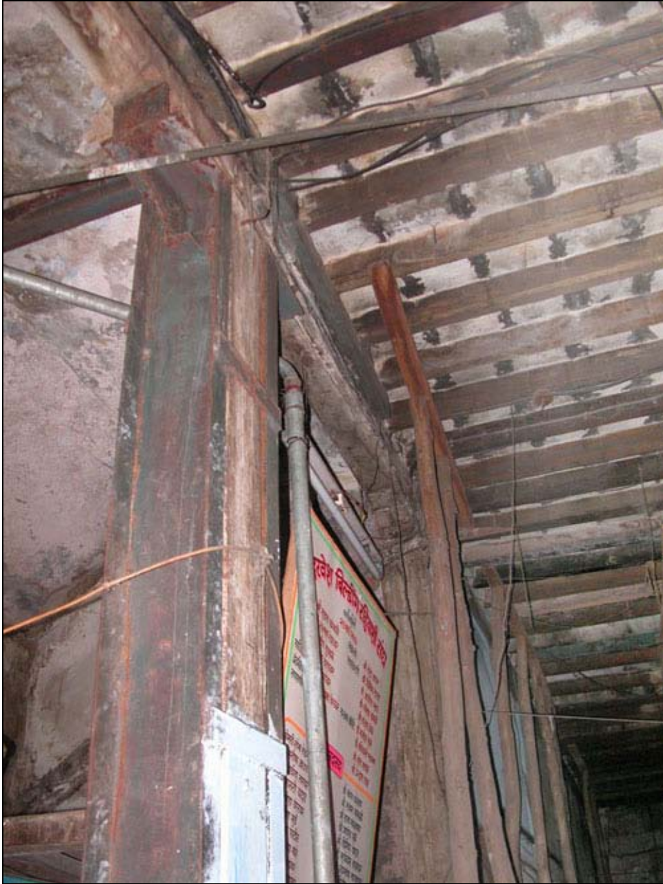
Figure 101 Ladikoba slab (S3-category)
