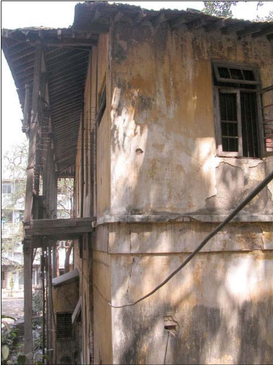
Figure 62 Timber column (S4-category)
