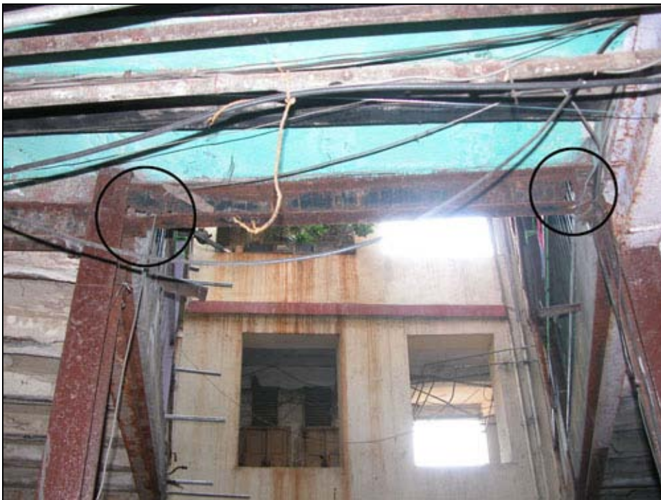
Figure 78 Steel beam (S3-category)
