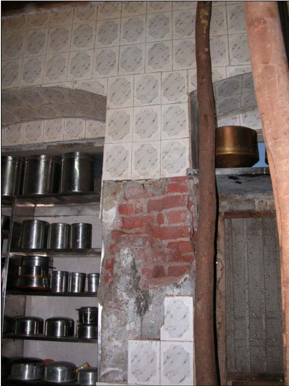
Figure 41 Masonry load bearing wall (S5-category)
