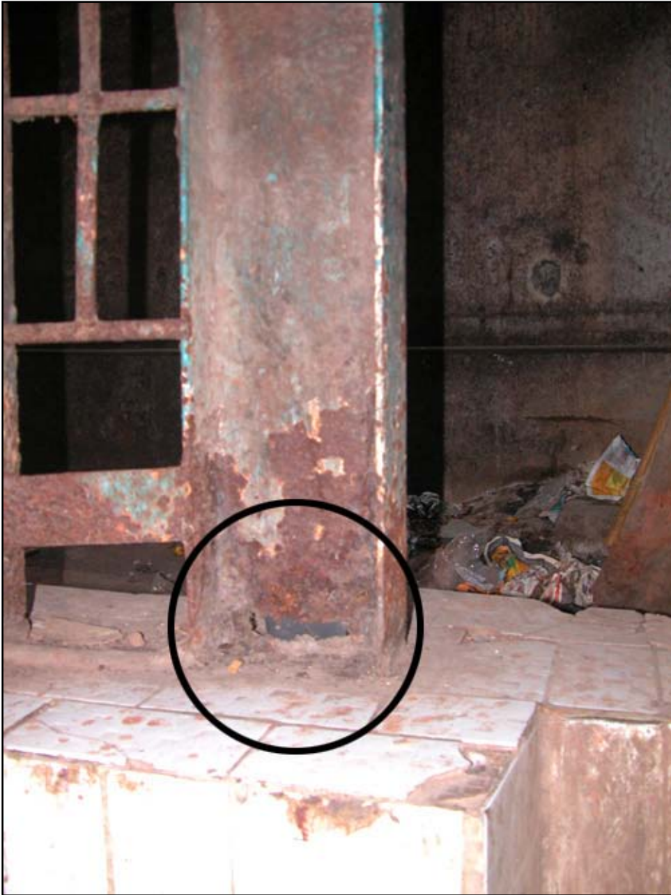
Figure 57 Steel column (S5-category)
