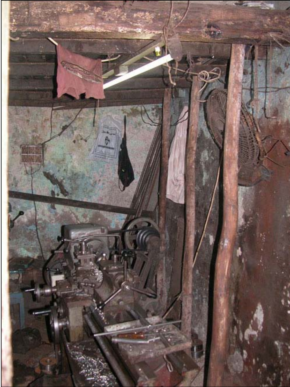
Figure 84 Timber beam (S3-category)
