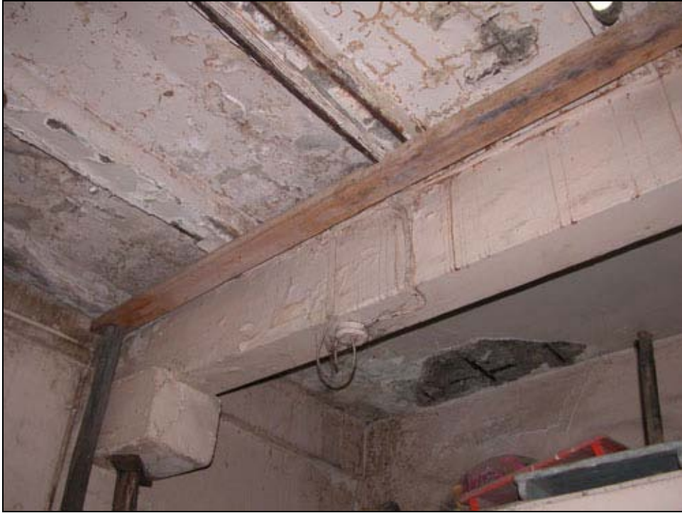
Figure 82 Timber beam (S3-category)
