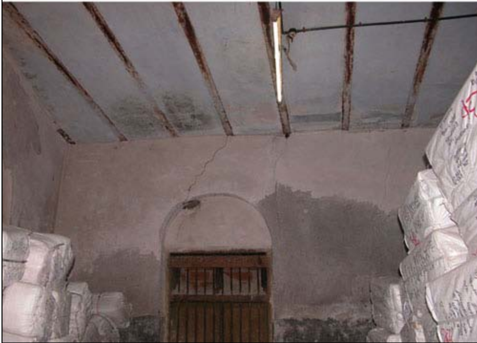
Figure 28 Masonry load bearing wall (S2-category)
