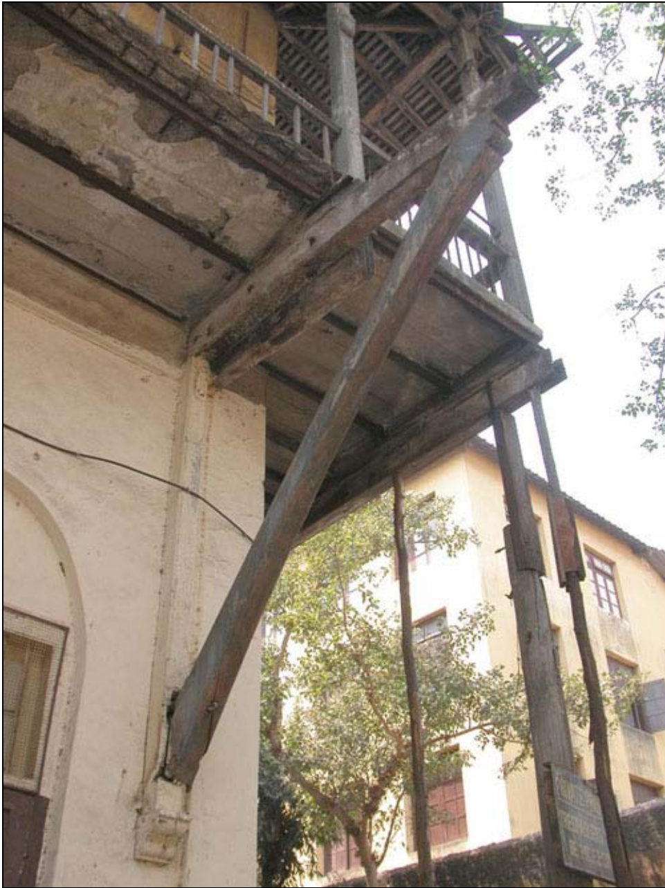
Figure 81 Timber beam (S3-category)
