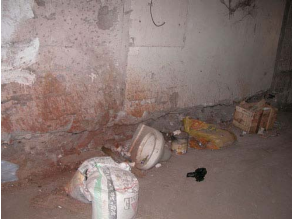
Figure 32 Masonry load bearing wall (S3-category)
