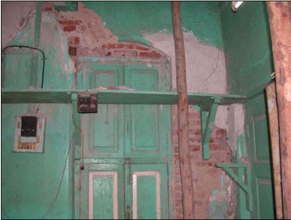
Figure 24 Masonry load bearing wall (S1-category)
