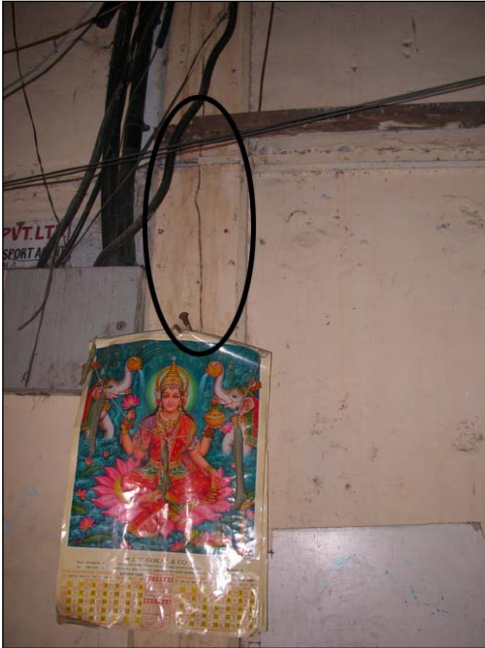
Figure 63 Timber column (S4-category)
