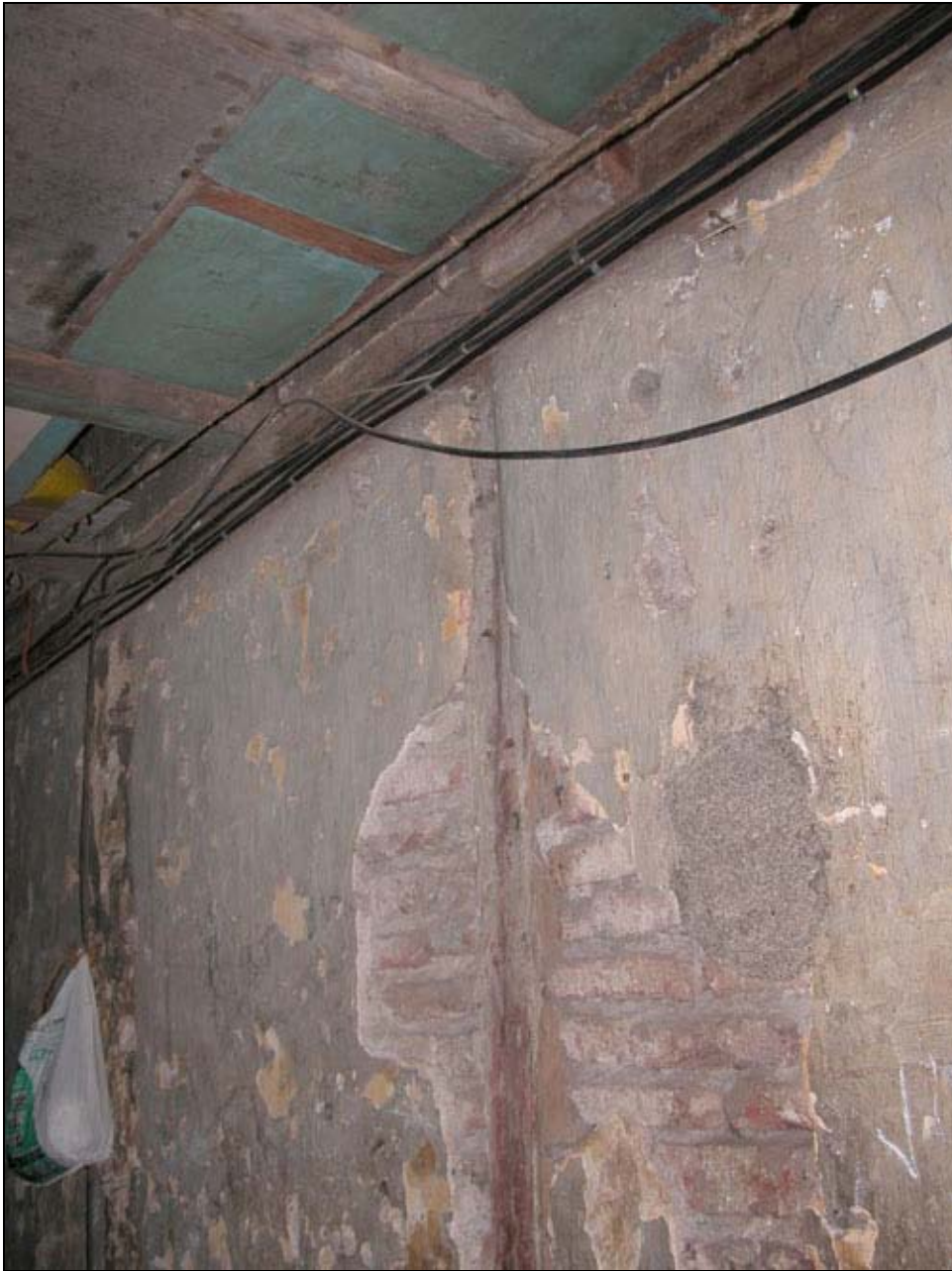
Figure 25 Masonry load bearing wall (S1-category)
