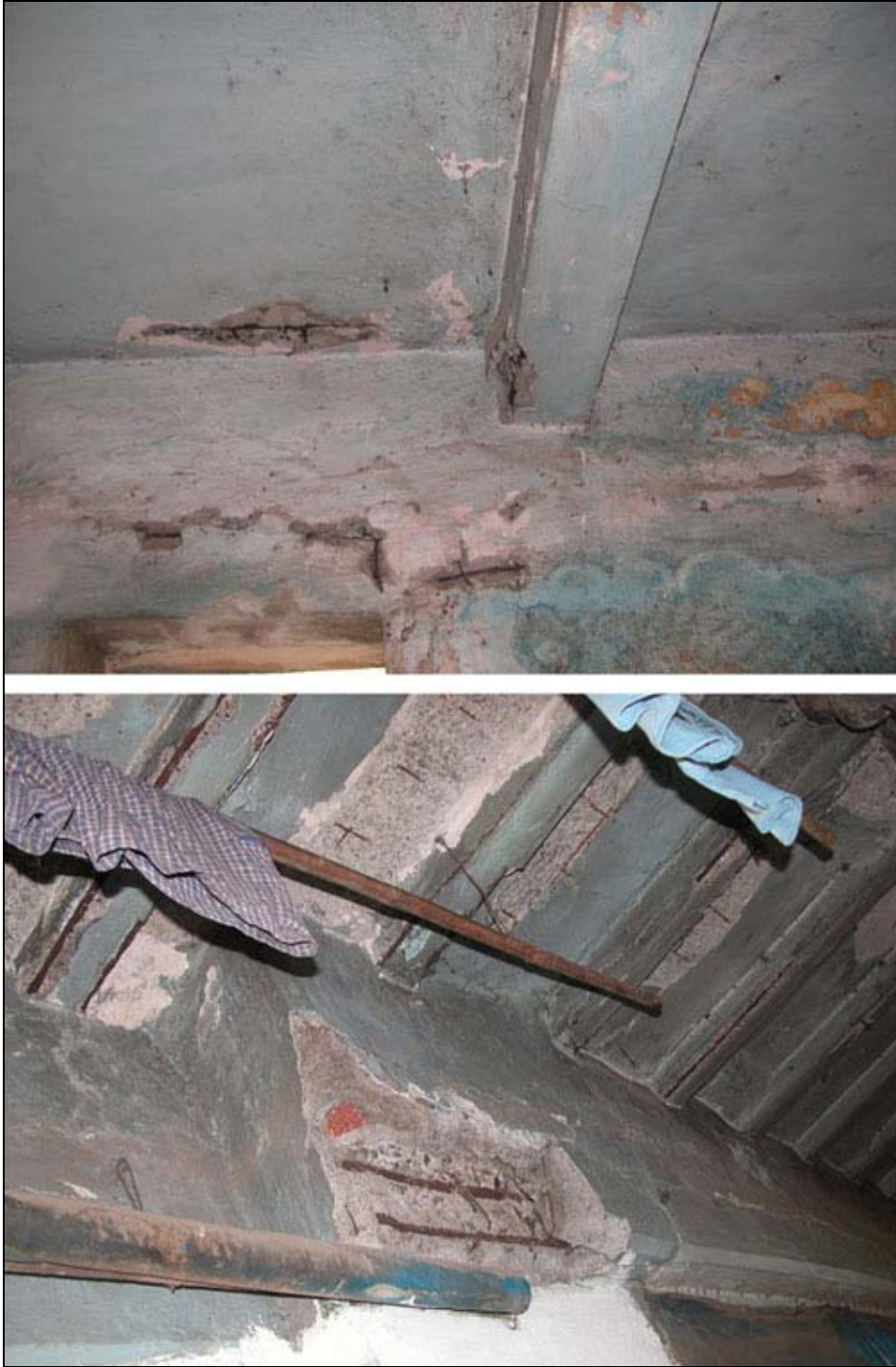
Figure 69 RCC beam (S2-category)
