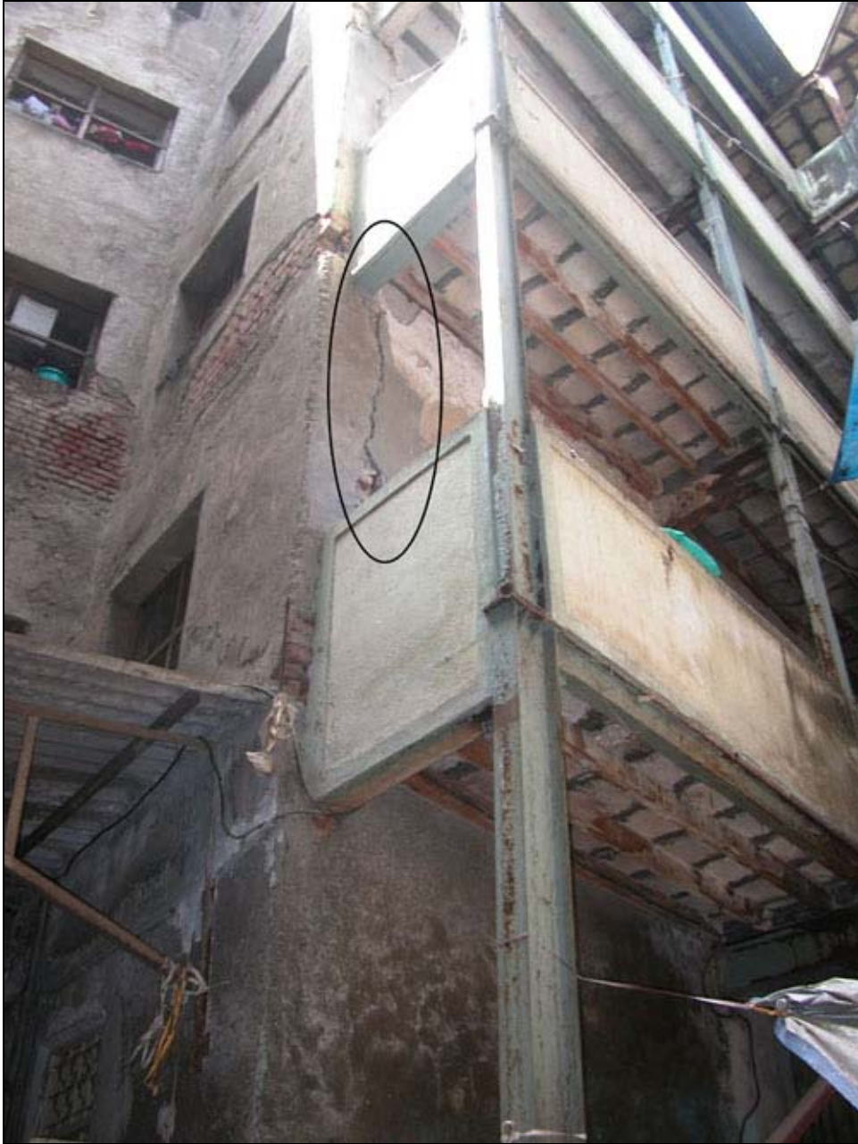
Figure 35 Masonry load bearing wall (S3-category)
