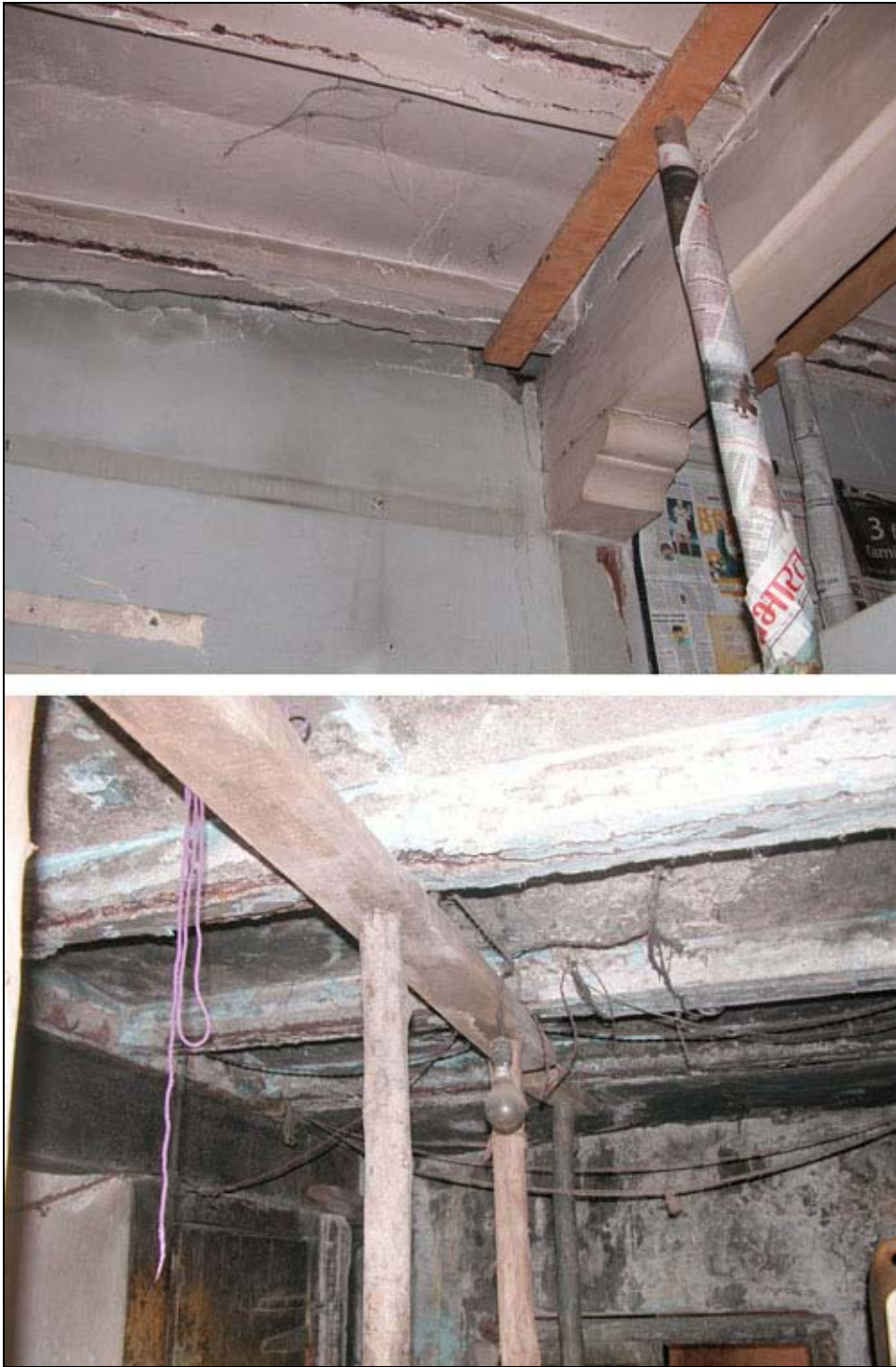
Figure 99 Cast stone slab (S3-category)
