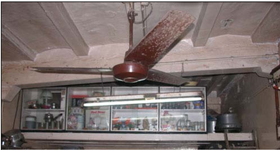
Figure 82 Timber beam (S3-category)
