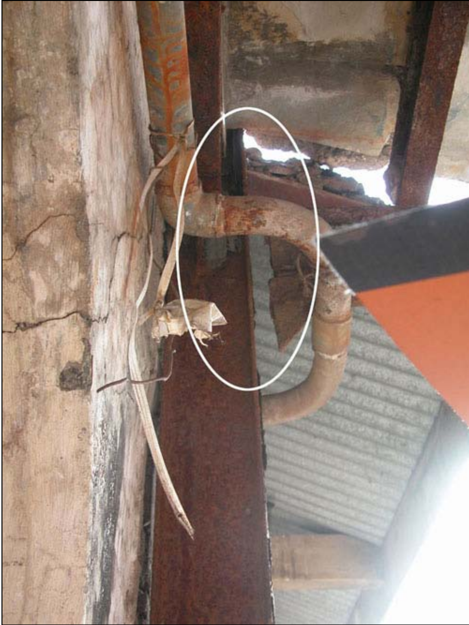
Figure 80 Steel beam-column junction (S5-category)
