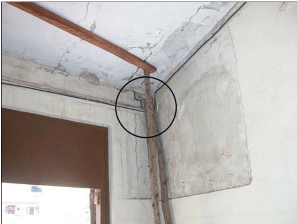
Figure 85 Timber beam (S3-category)
