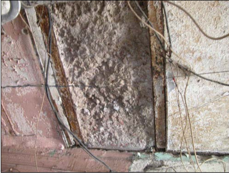
Figure 102 Ladicoba slab (S4-category)
