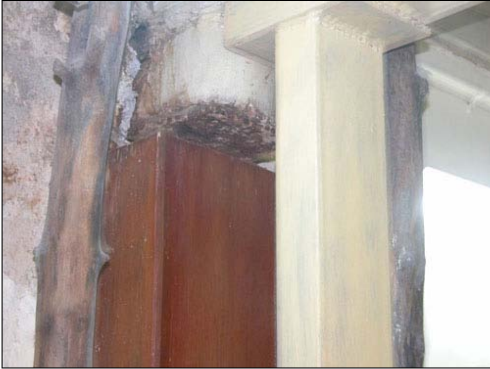
Figure 58 Timber column (S3-category)
