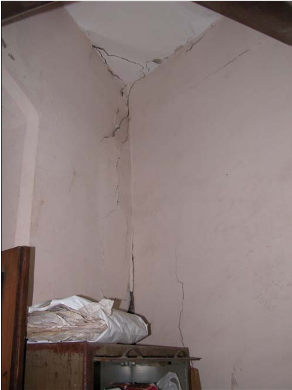
Figure 26 Masonry load bearing wall (S1-category)
