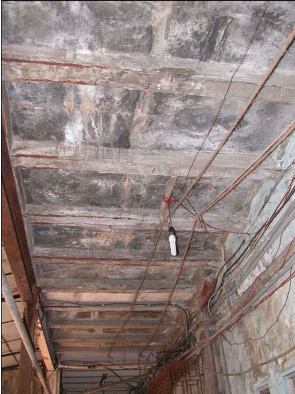
Figure 91 RCC joists (S2-category)
