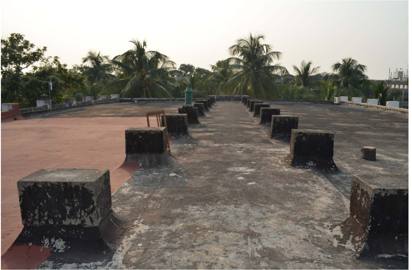
Roof view showing the column positions
