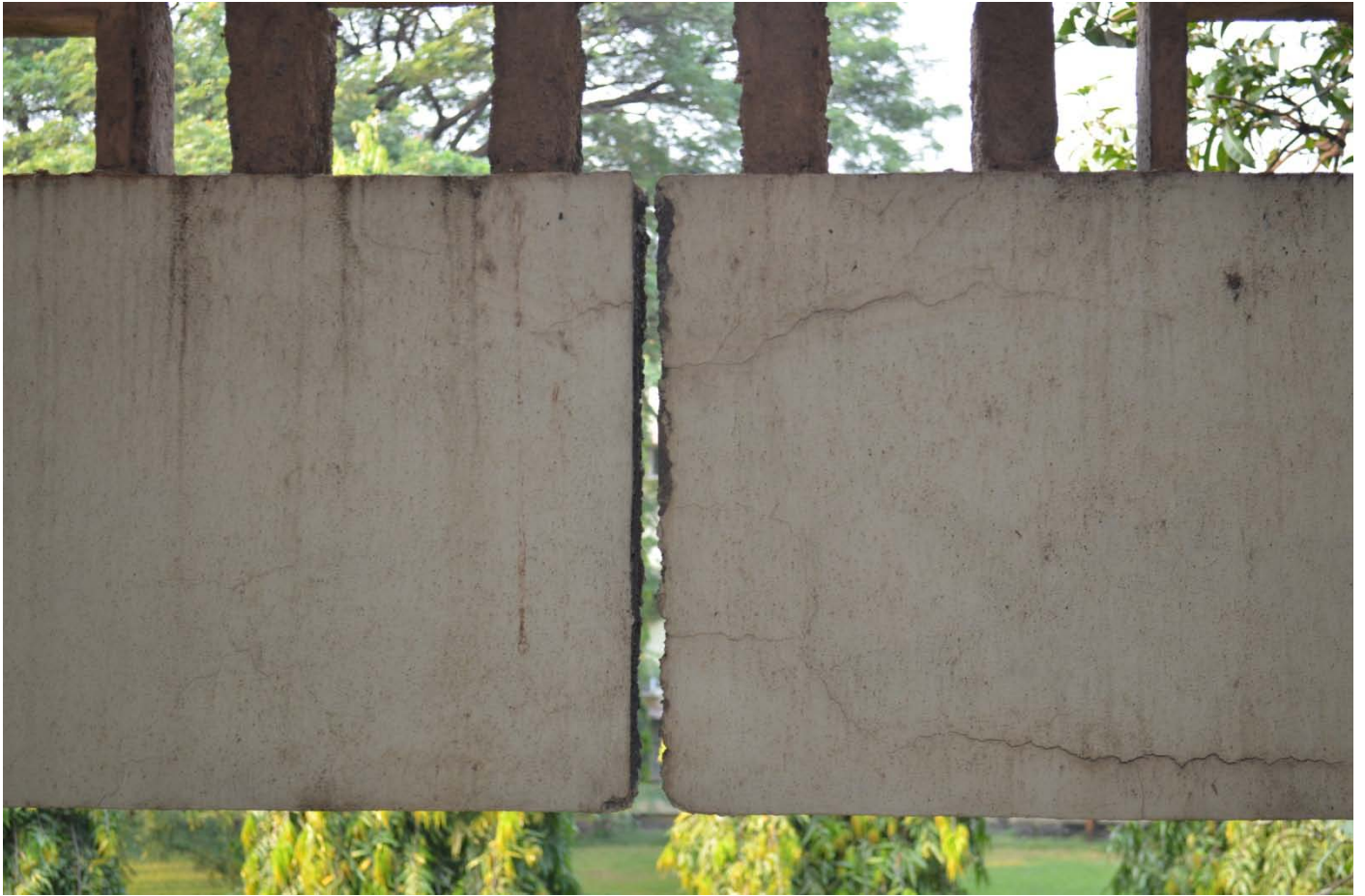
Expansion joint splitting the structure into two buildings
