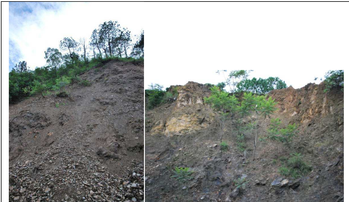
Figure 35.1. a. Soil c/s near site 1, b. soil c/s near site 4, c. Shear wave profiles of all the test sites in Solan
