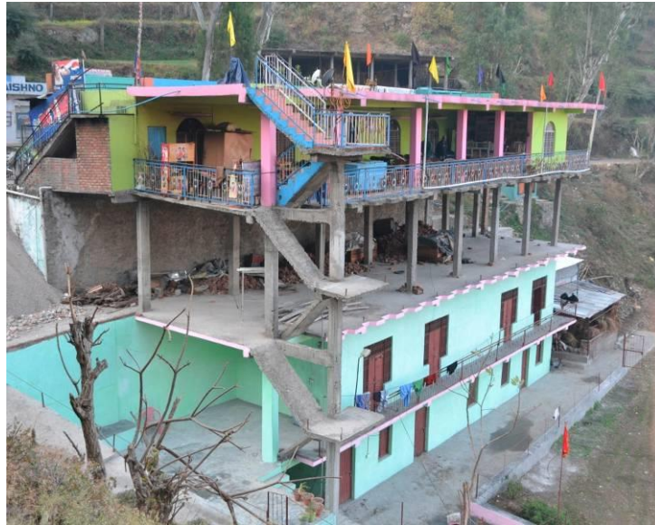
Figure 38: Structural irregularities are present in the building at Kangra district
