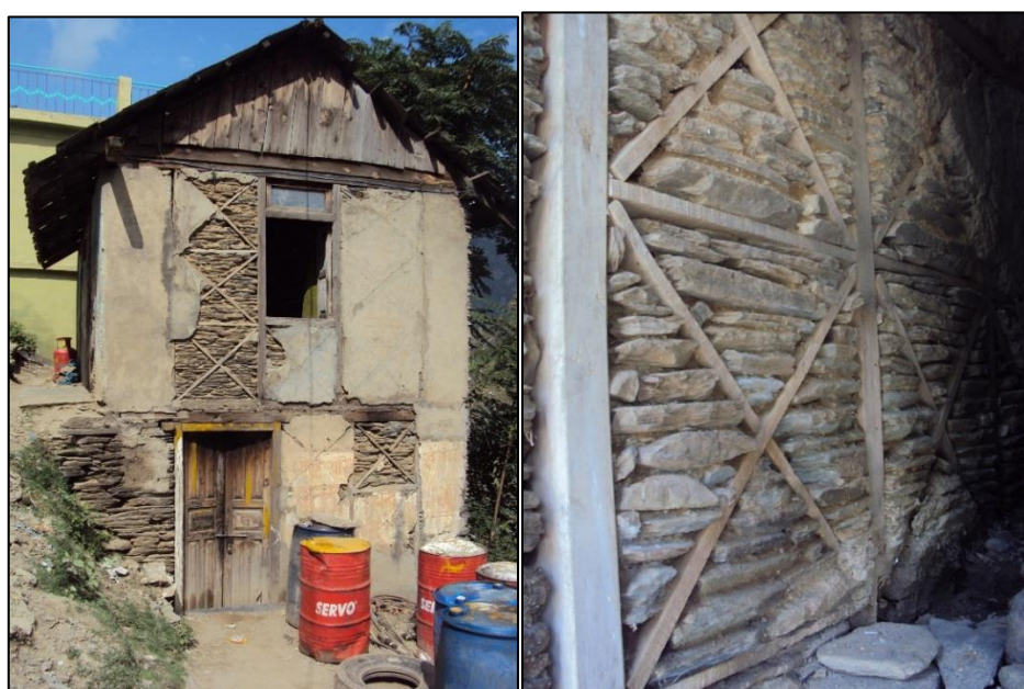
Figure 19: Dhajji Dewari Type House (Shimla, 13 th November 2013)
