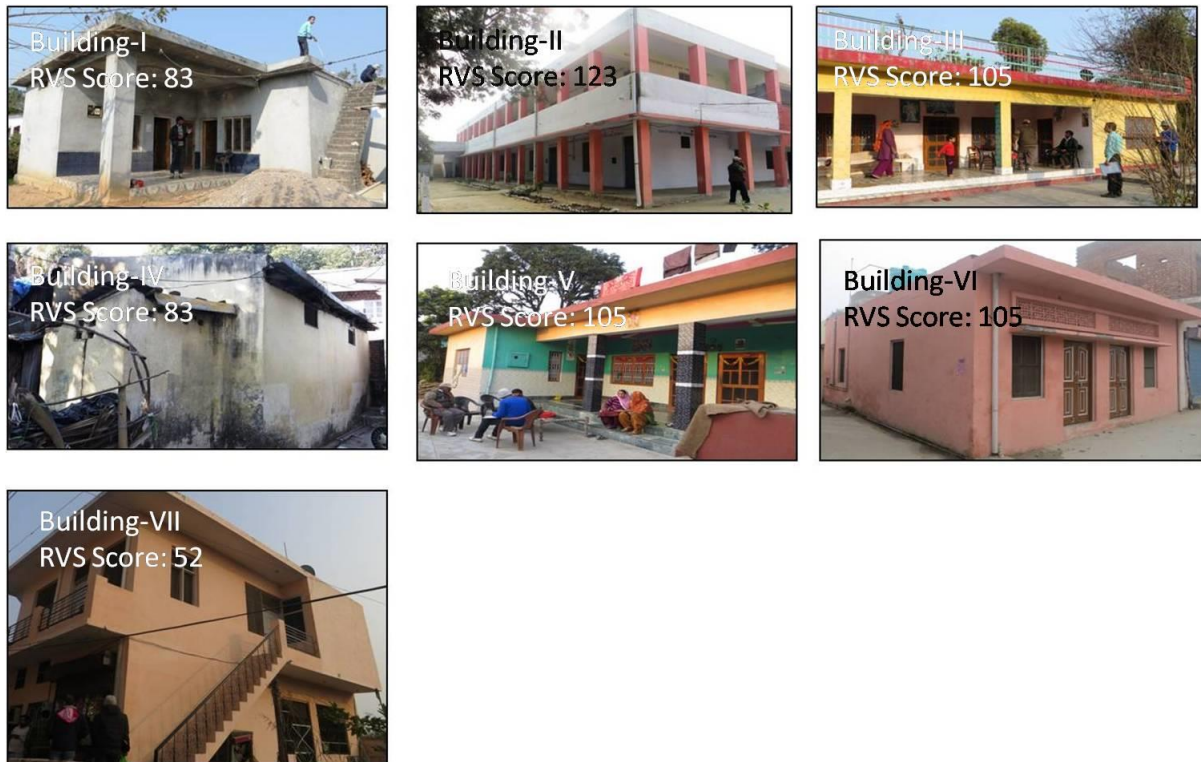
Figure 87: General View of brick masonry Buildings
