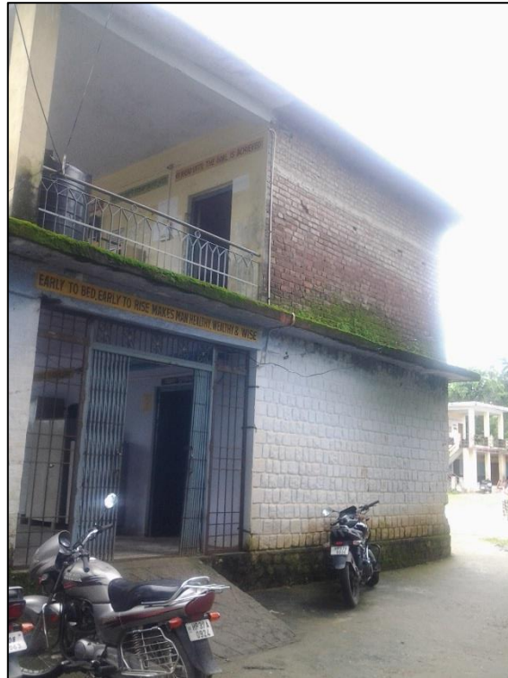
Figure 25: Hybrid Construction (Stone masonry and brick masonry)
