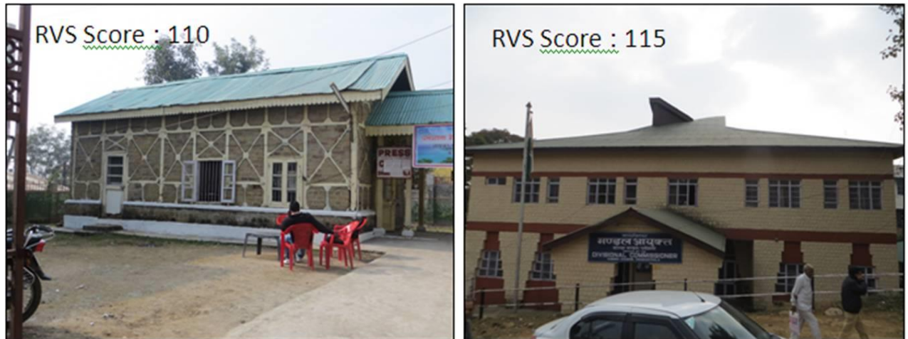
Figure 88: General View of stone masonry Buildings
