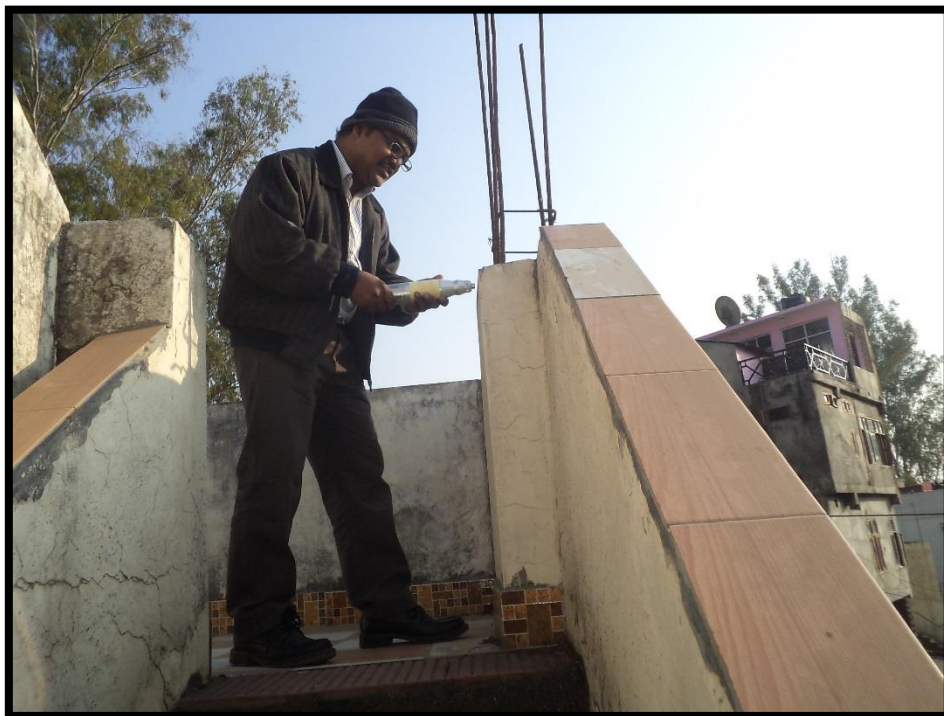
Figure 73: Rebound Hammer Test (Hamirpur, 15th December 2013)
