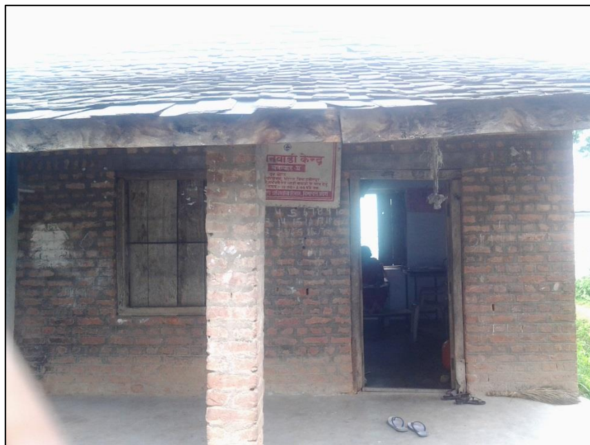
Figure 23: Brick Masonry construction of Anganwadi (Bhoranj, Hamirpur, September 2013)
