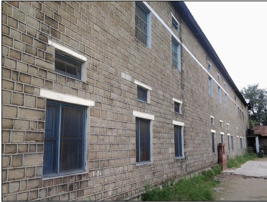
Figure 22: PWD office building in Hamirpur (Hamirpur, 23rd August 2013)
