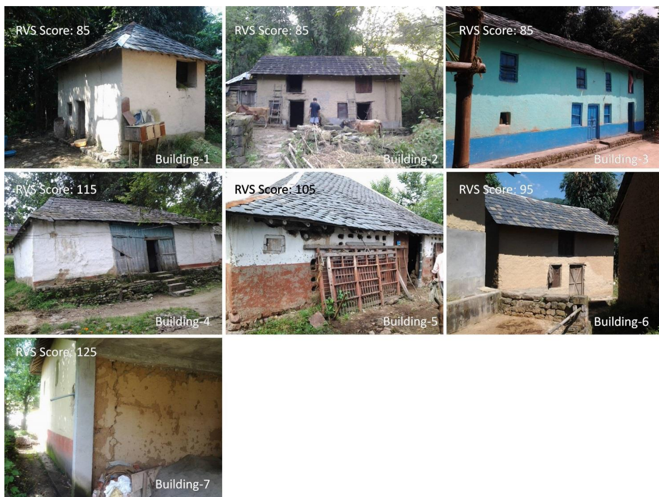
Figure 89: General View of rammed earth Buildings
