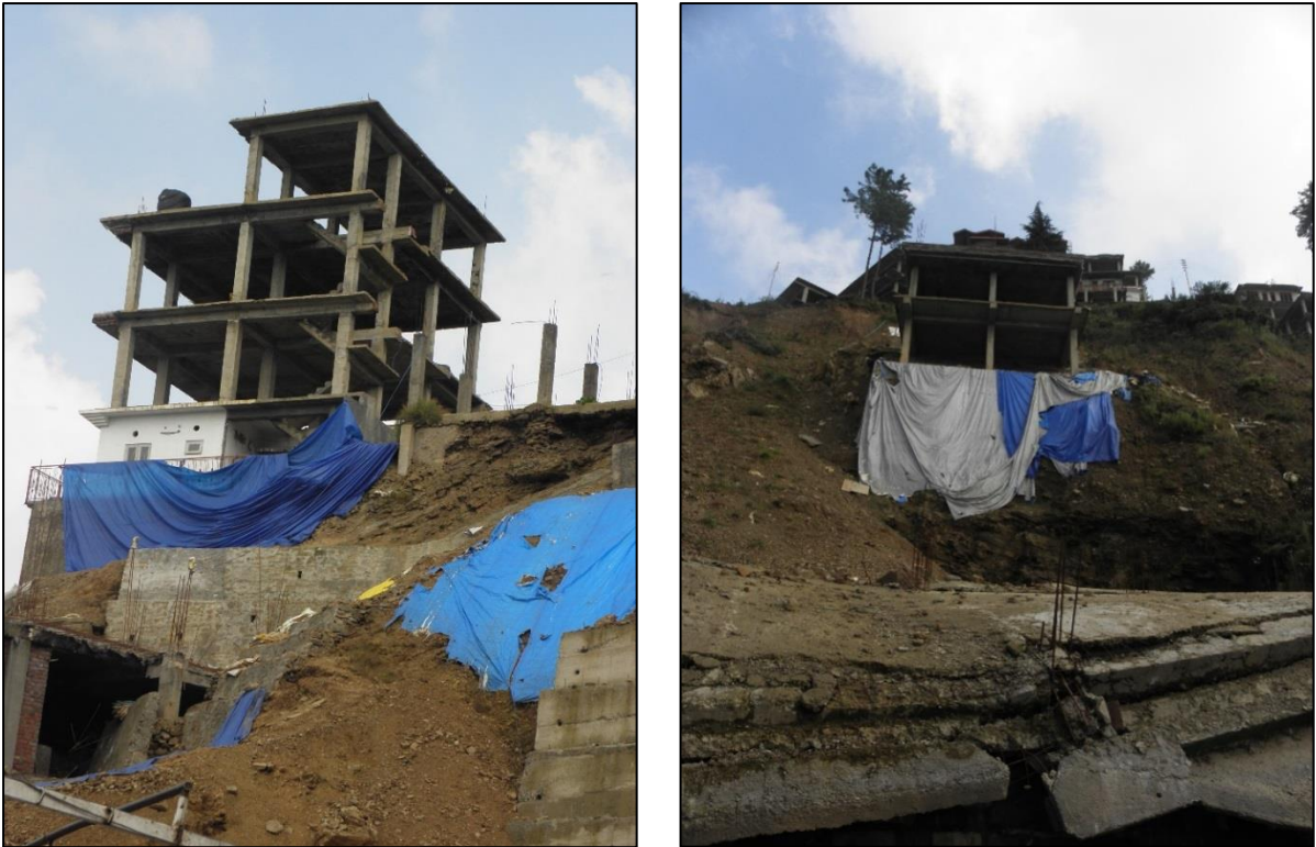
Figure 30: Construction of building on sloping site
