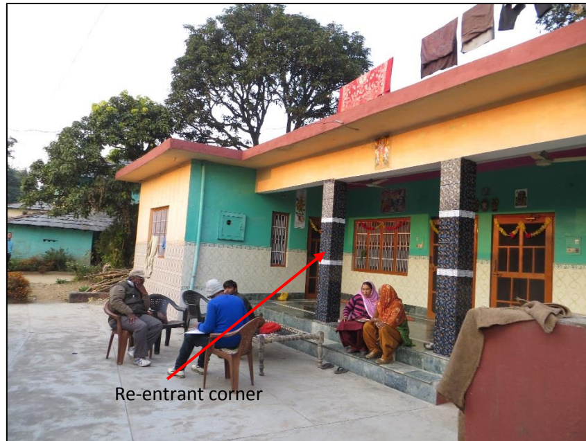
Figure 29: Re-entrant corner in L shape building (Kangra, 17th December 2013)
