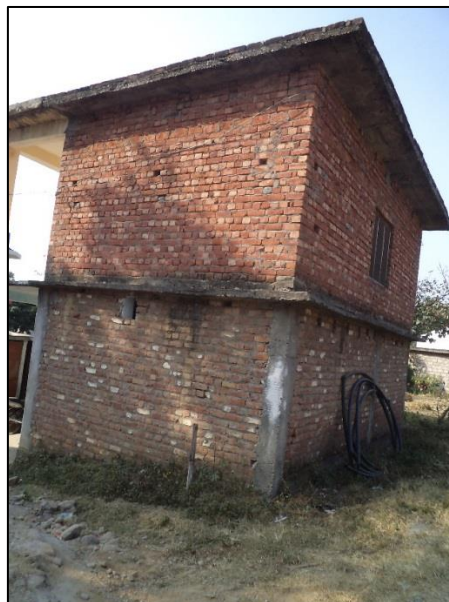
Figure 24: Hybrid Construction (RC Frame and Brick Masonry) in Kangra
