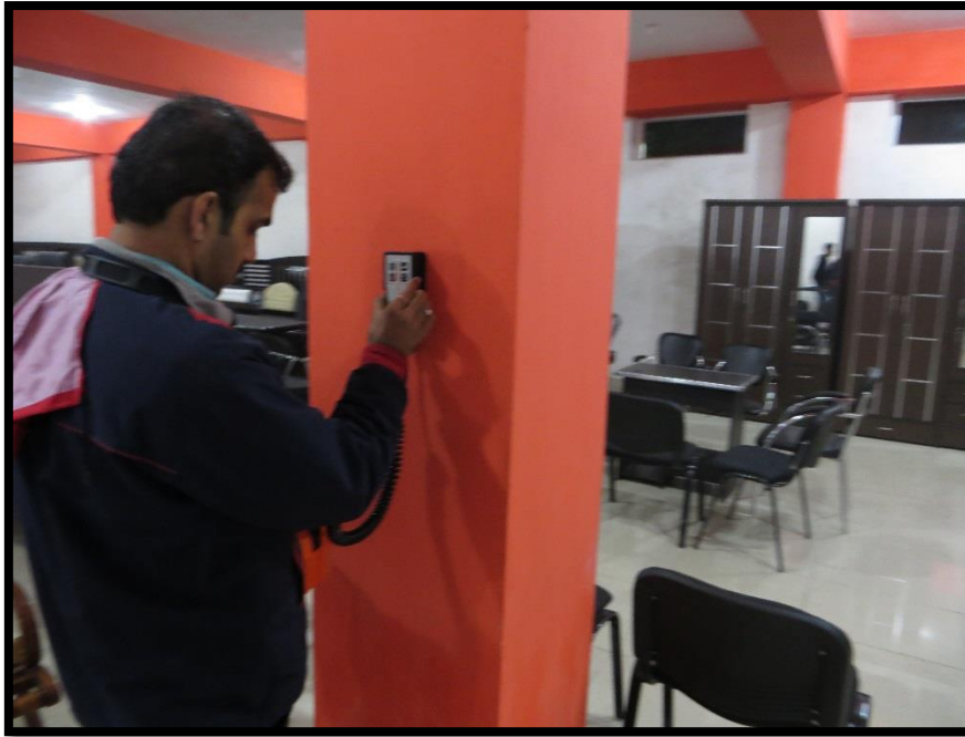
Figure 76: Rebar Locator Test (Kangra, 17th December 2013)
