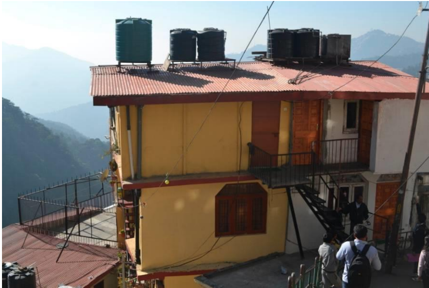
Figure 39: Heavy overhangs are present on the top of structure at Kangra district
