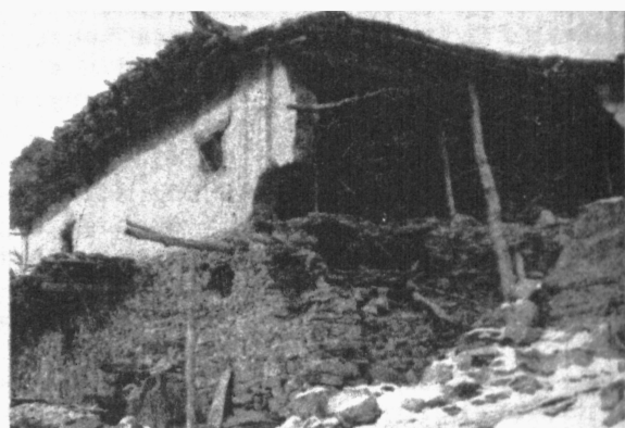
FIG. 2 - COMPLETE COLLAPSE OF SUNDRIED MUD BRICK WALL OF A DOUBLE STOREYED HOUSE AT SHALKAR. THE GROUND FLOOR IS IN RRS IN MUD MORTAR
