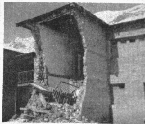
FIG. 5 - COLLAPSE OF STAIRCASE WELL IN A DOUBLE STOREYED HOUSE OF DSM IN MUD MORTAR AT LEO
