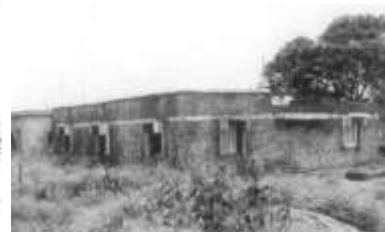
(b) A building with horizontal lintel band in Killari village: no damage
