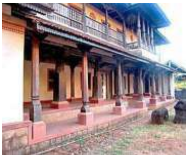
Ashlar Stone Walls with Mangalore tiles gabled roof- Karnataka
