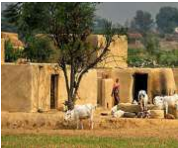
Cob walls with timber and mud flat roof - Haryana
