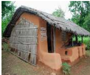
Cob walls with thatch gabled roof - Madhya Pradesh
