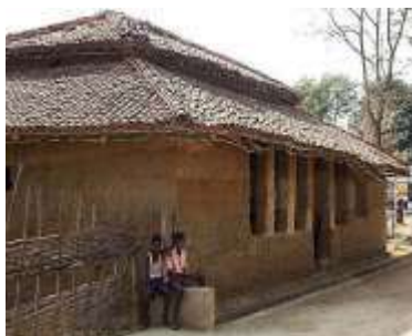
Cob walls with tiled hipped roof - Chhattisgarh
