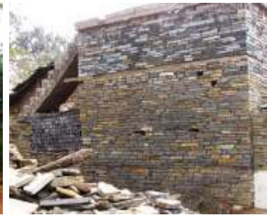
Ashlar Stone Walls with country tiles hipped roof- Chattisgarh
