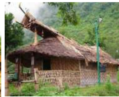
Wattle and daub walls with thatch roof - Nagaland
