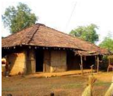
Wattle and daub walls with Mangalore tiles hipped roof - Maharashtra
