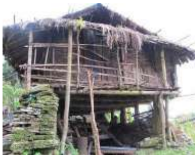
Timber walls with thatch hipped roof- Sikkim
