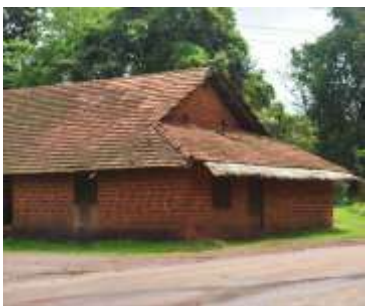
Ashlar Stone Walls with Mangalore tiles hipped roof- Goa
