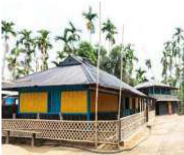
Wattle and daub walls with sheet hipped roof - Kerala
