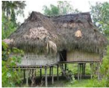
Wattle and daub walls with thatch hipped roof - Arunachal Pradesh
