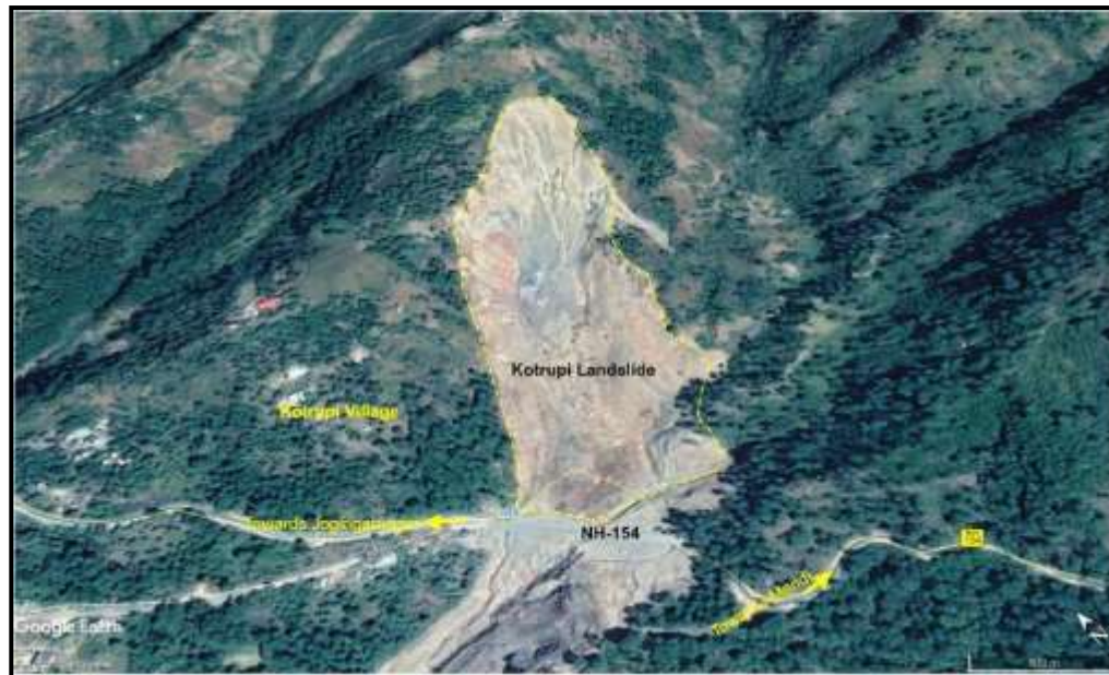
Fig.-3: Updated/ Post-2017 incidence satellite view of Kotrupi Landslide [Part of NH-154 can be seen repaired] [Source: Google Earth].
