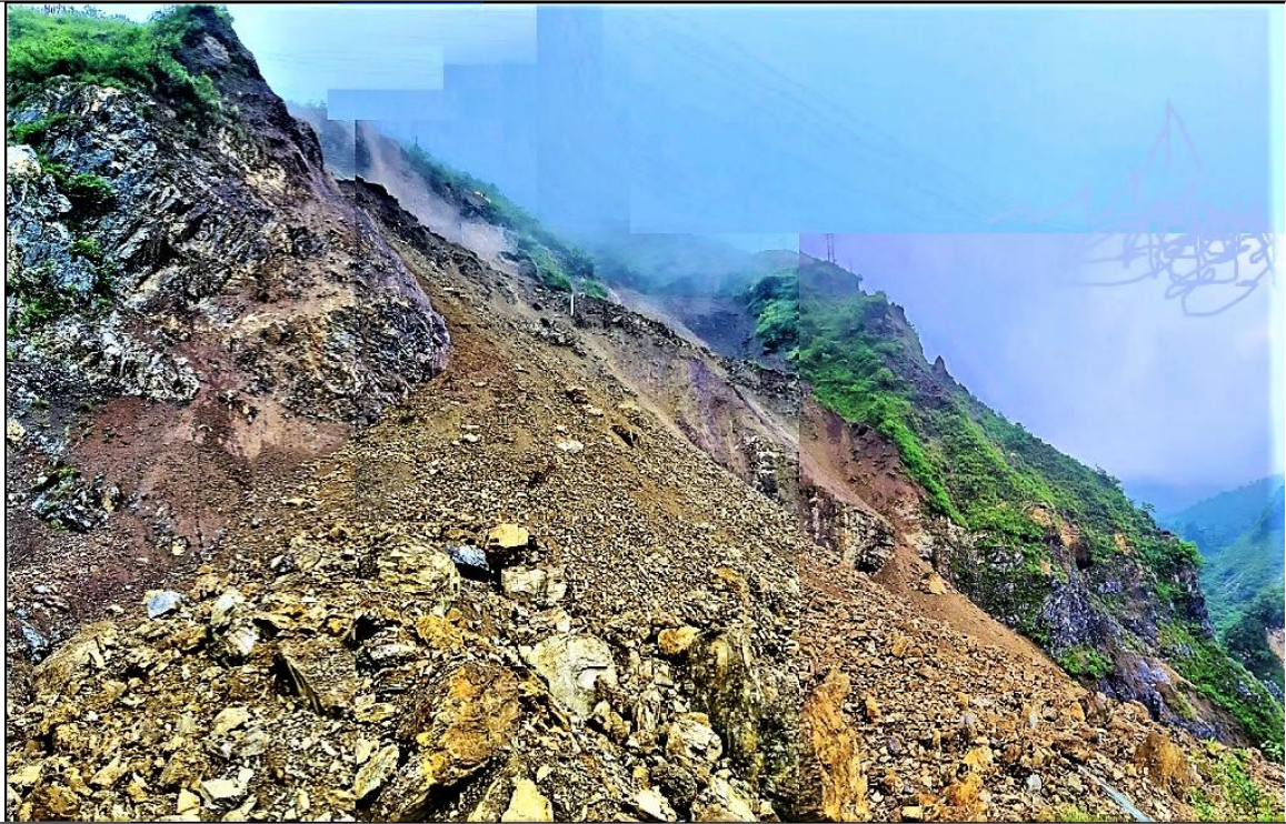
Fig.-7: Uphill view of the landslide shows dislodged large oxidized bed rock blocks possibly derived from the toe part.
