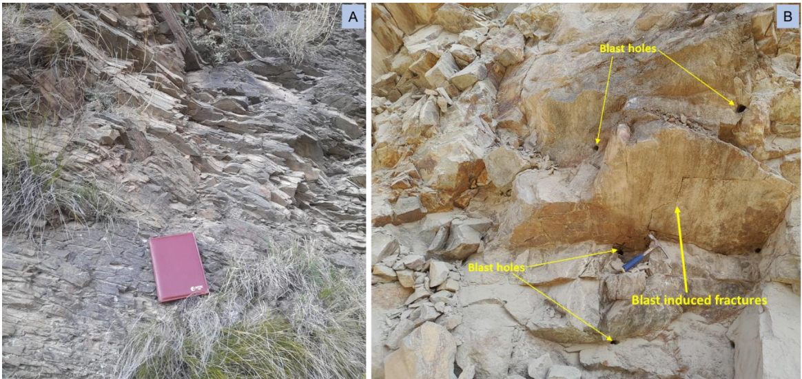
Photo 10. (A) The thinly bedded, lighter colored schistose quartzites seen at the higher slopes, (B) Blast induced fractures in the rock mass.
