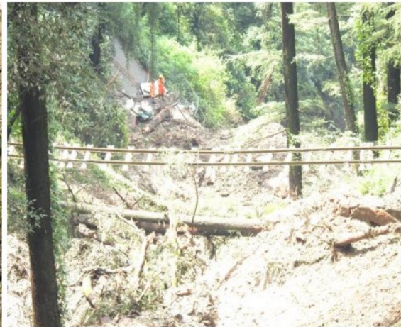
Damaged railway track along the path of slide
