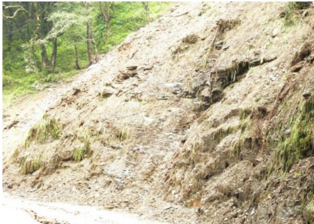
In-situ rock exposed along the road section
