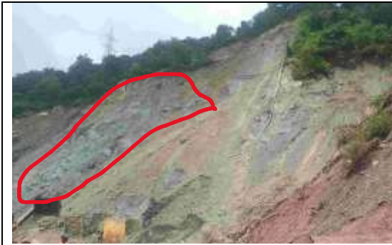
i. Rock mass exposed after the removal of debris cover
