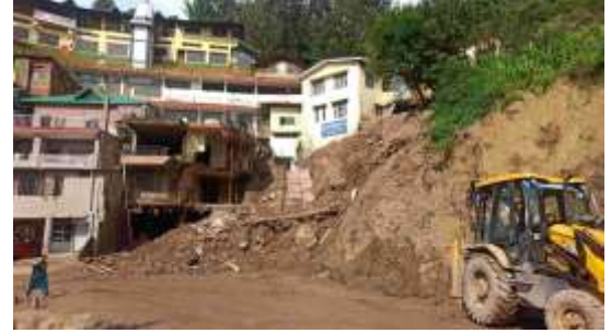
m. Debris slide near BL School
