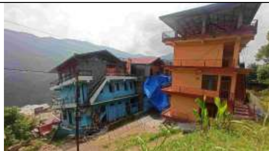
k. Tilted house in Shamti area.
