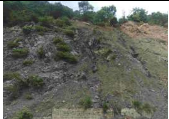
b. The highly jointed rock mass exposed along the road.
