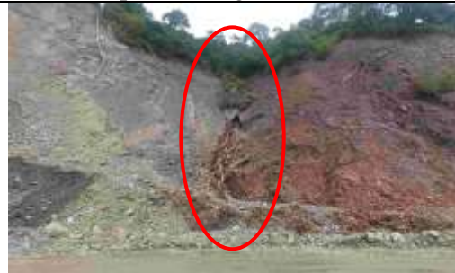
d. Flowing hydrological conditions along the affected slope.
