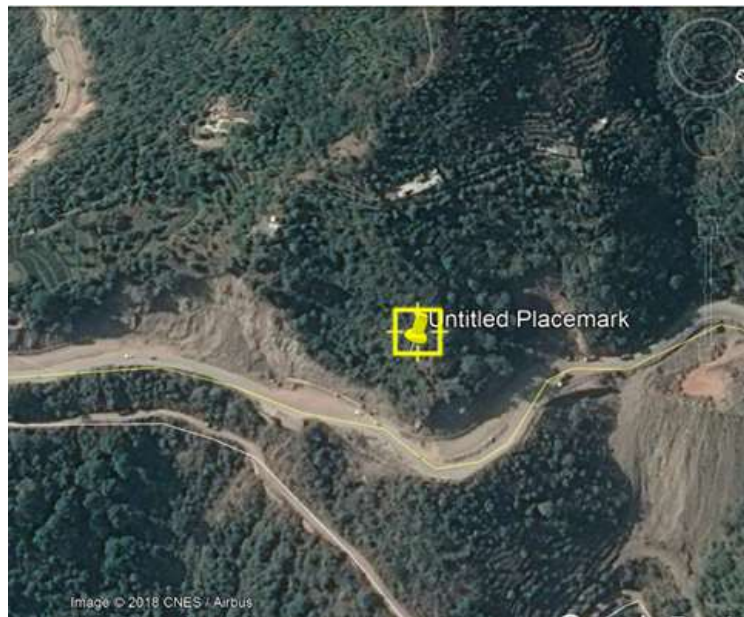
Fig. 13A: Location Map of the Chaki Morh Slide at NH-05/ RD: 87+480, (Source: Google Earth)
