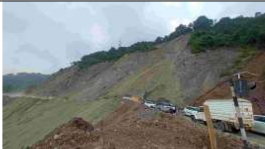
c. Steep cut slope exposed along the NH 05.
