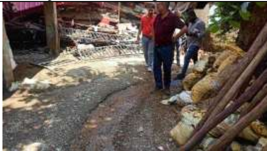
g. Flowing conditions in the vicinity of damaged houses.
