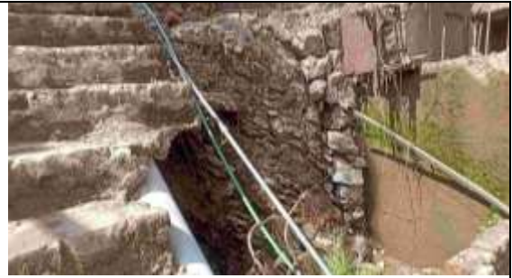
b. Highly disintegrated dolomitic limestone.
