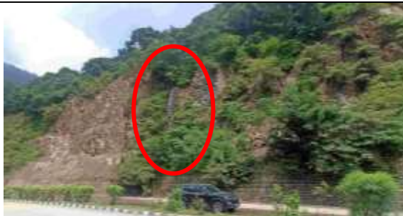
e. Flowing hydrological conditions along the affected road.
