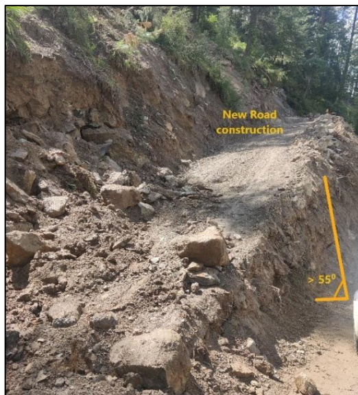
Fig. 33. New Road construction with large slope angle.
