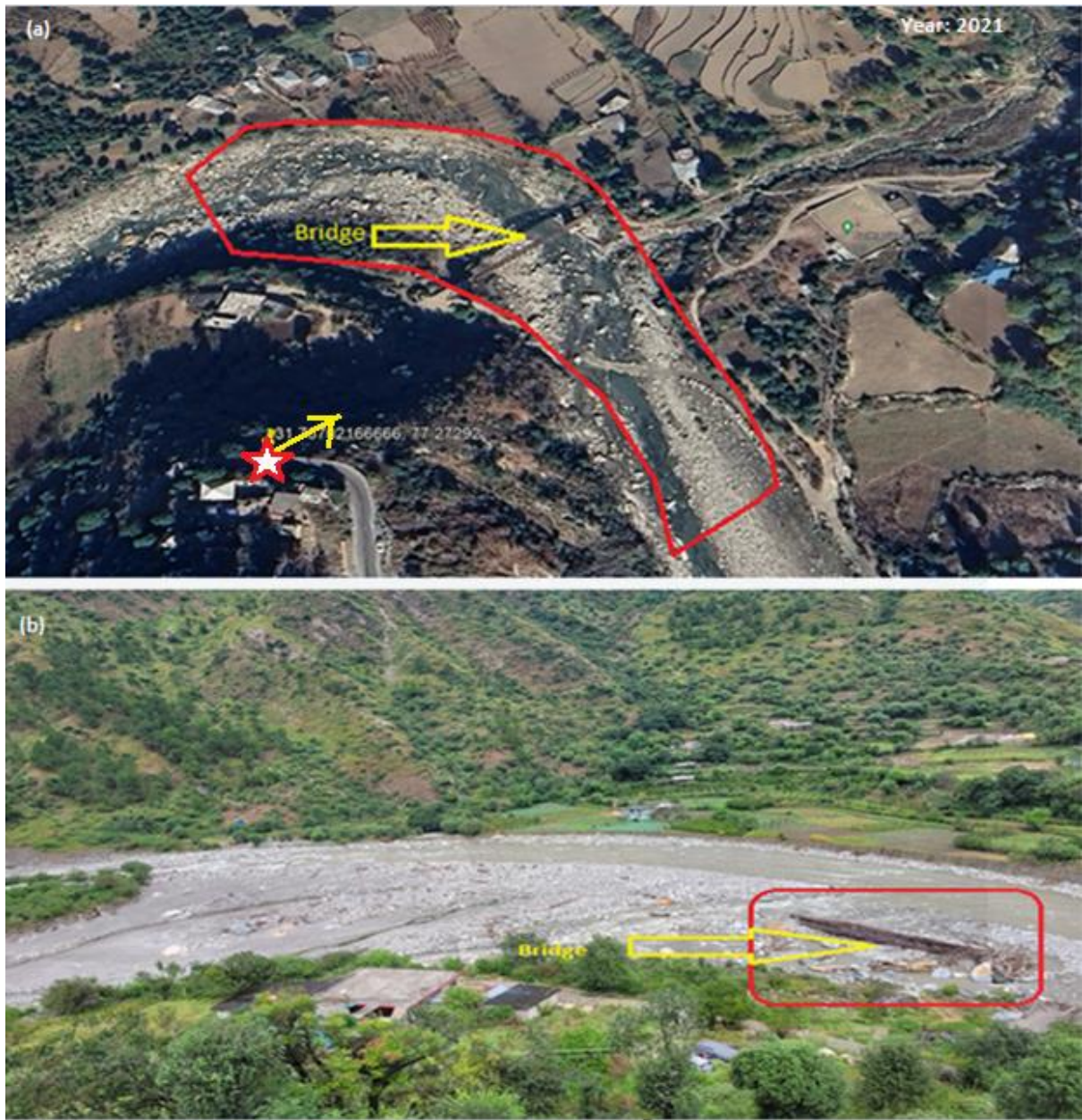
Fig. 14. The main vehicular bridge providing connectivity at Tareda village has been completely washed away by the high-intensity flash flood event. Additionally, 2-3 houses situated precariously along the edges of the river were also swept away.
