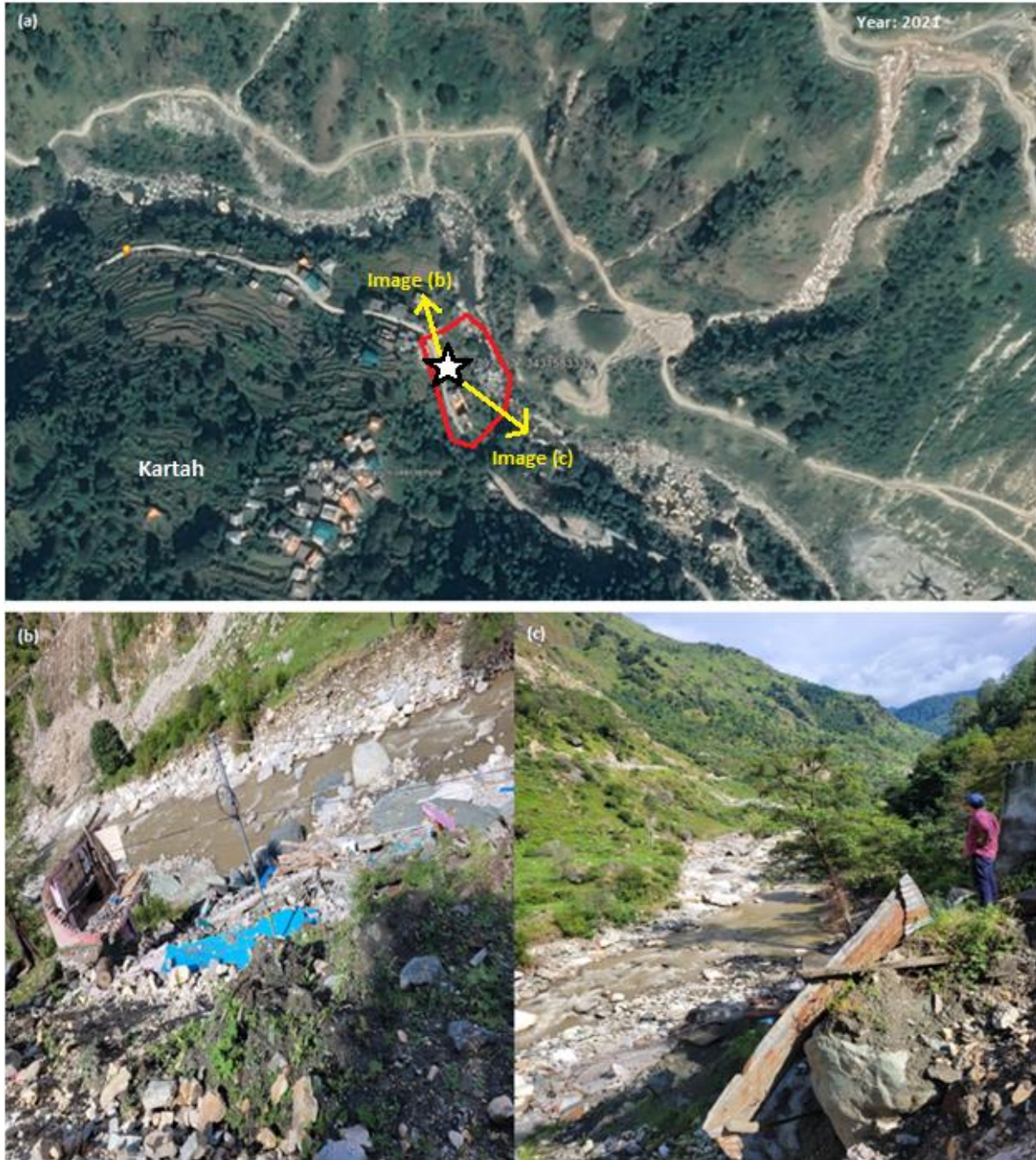
Fig. 20. In Kartoh village, approximately 5 houses constructed at the base of a hill were completely buried under debris due to a major landslide spanning over 150 meters wide. Tension cracks were visible on the slope.
