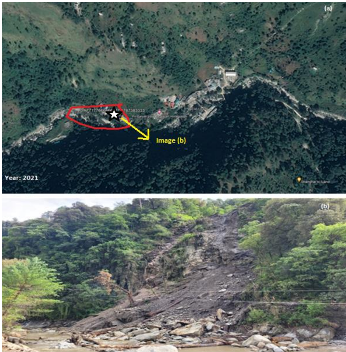
Fig. 21. A massive landslide extending over 40 meters vertically has occurred at Neuli village, fully destroying a connectivity bridge. The landslide has blocked access across 4-5 panchayats, requiring a makeshift crossing.
