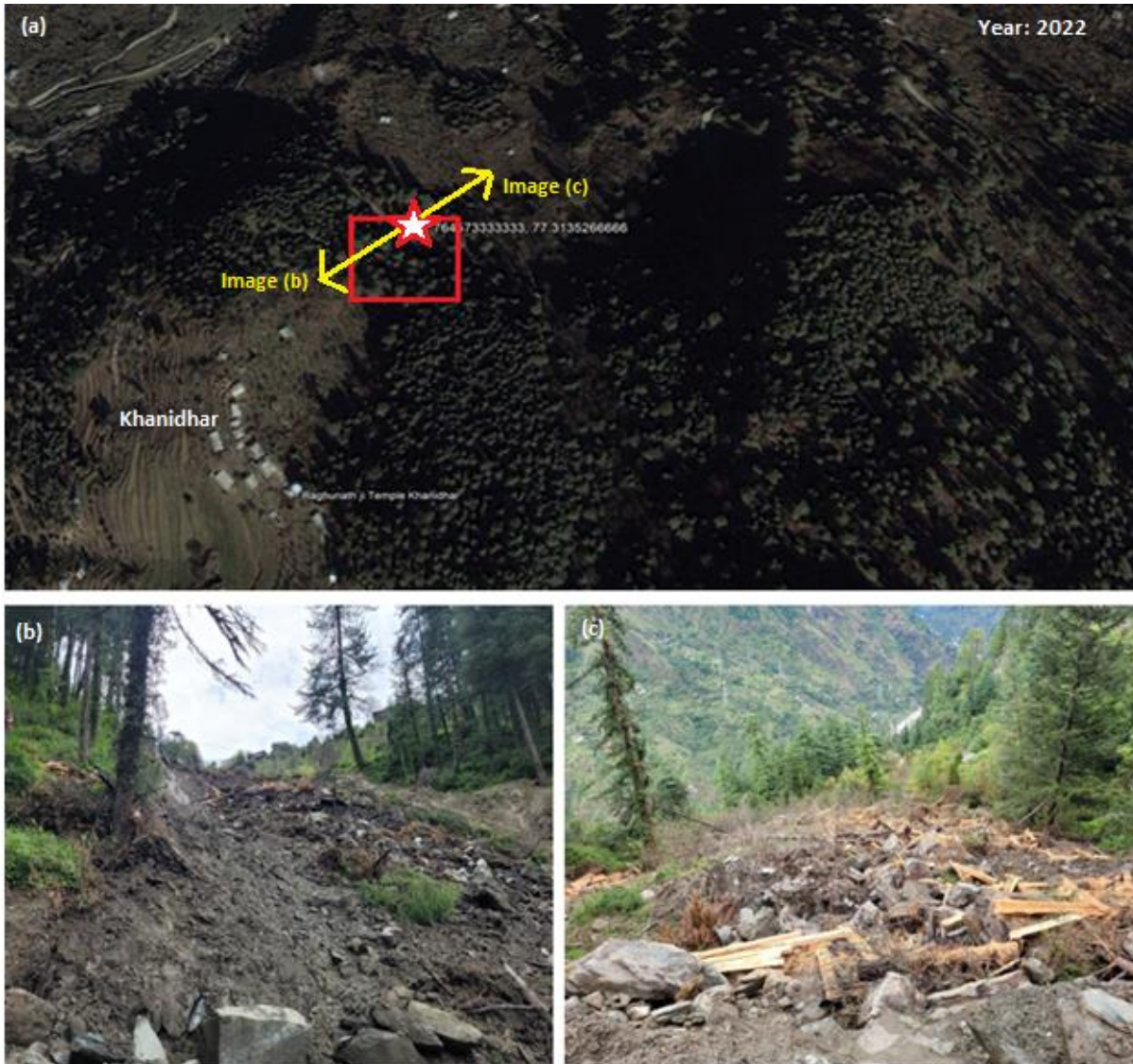
Fig. 16. A major landslide spanning approximately 200 meters wide has occurred at Khanidhar village, leading to destruction of several old growth deodar and apple orchards on the hillside.
