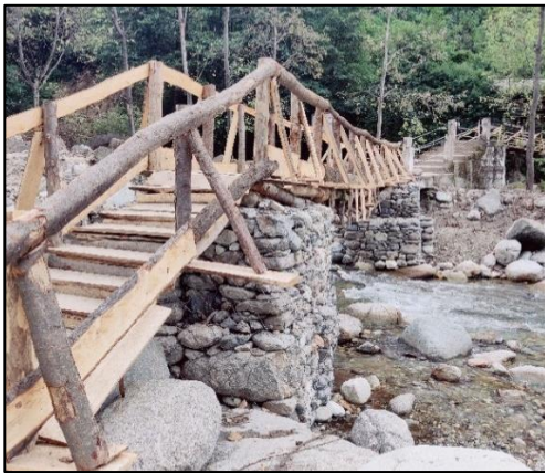
Fig. 35. Temporarily constructed bridge.
