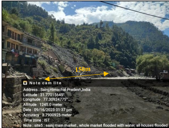
Fig. 44. Sainj main market 150 m damaged stretch.
