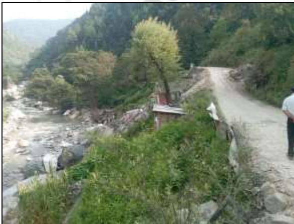
Fig.56; Damaged houses towards the valley side of the slide at Kartah.
