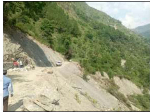
Fig.38; Road subsidence along Machine Nala landslide.
