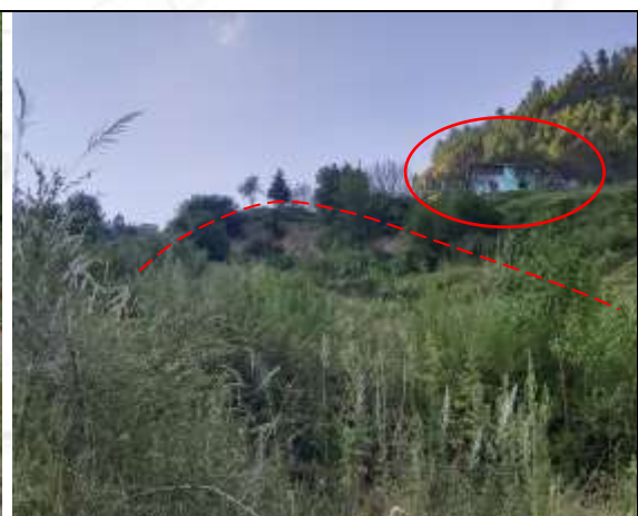
Fig.67. Houses in high risk zone observed on the crown portion.
