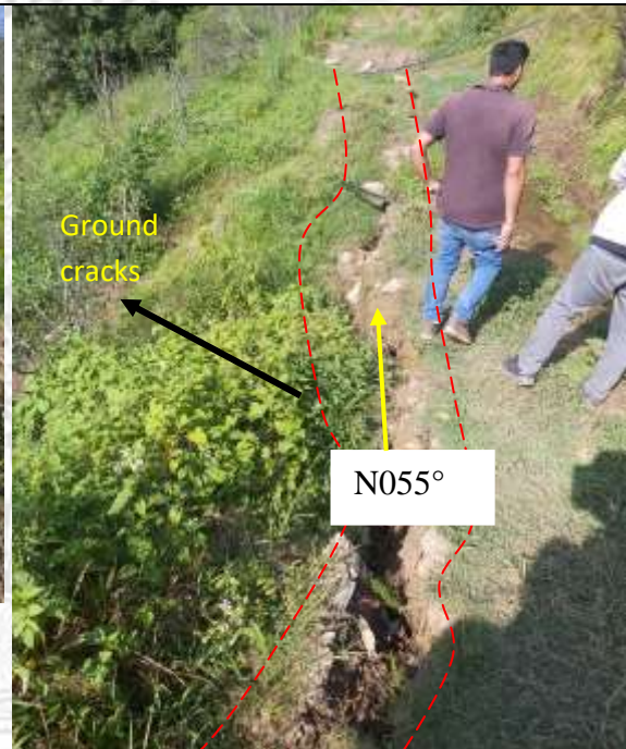
Fig.2. Open ground cracks in Chehava slide
