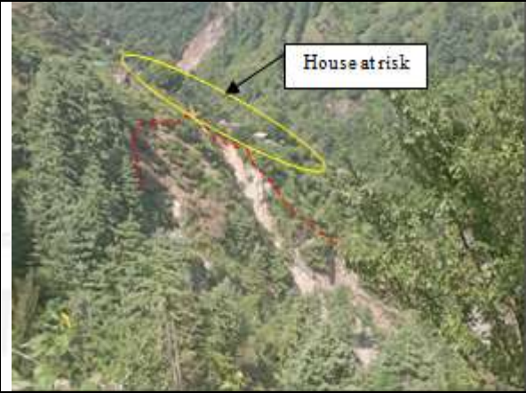
Fig.3. Landslide on right flank of the slope
