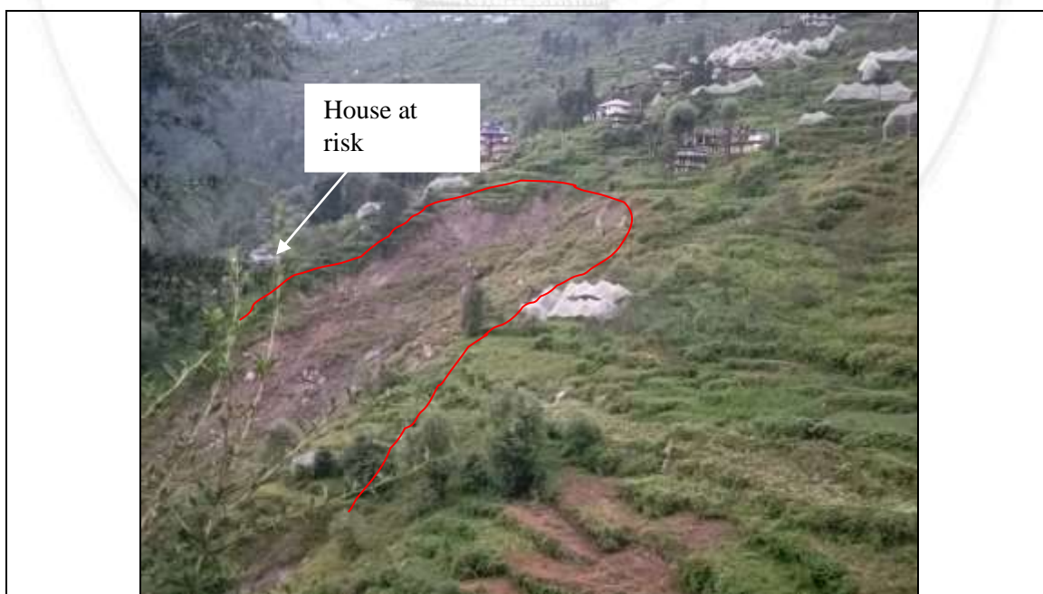
Fig.78.a; Field photograph showing Kot Nala landslide.
