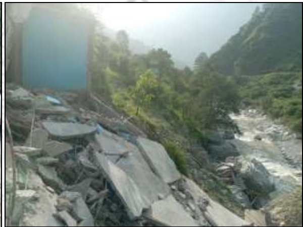
Fig.57; Damaged houses located near the bank of River at Kartah.
