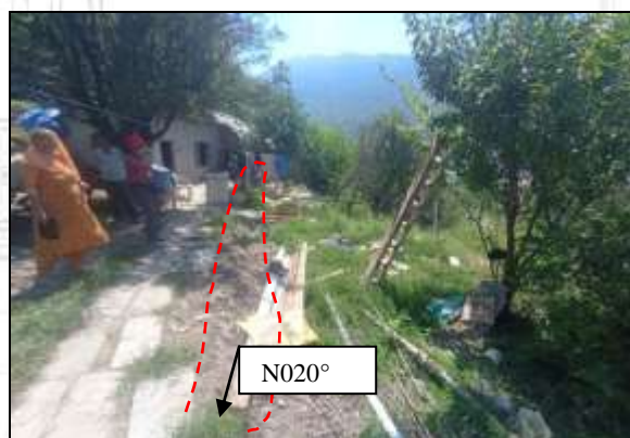
Fig.14; Ground cracks observed at Banontar Kharahal
