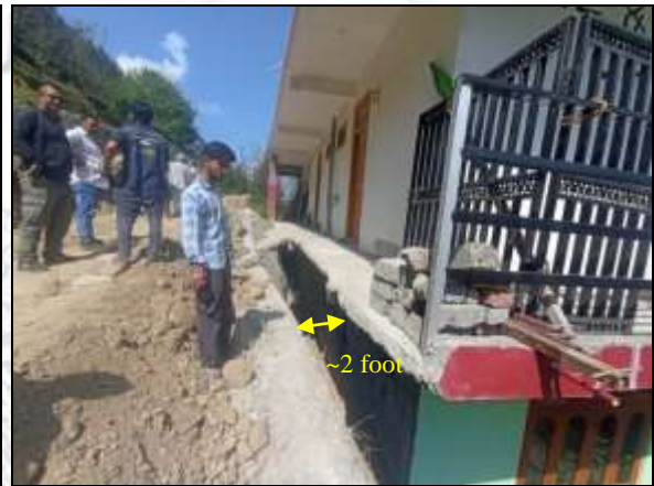
Fig.30 ; Damaged retaining wall towards valley side of lowermost road level.
