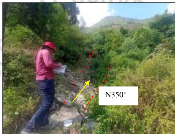
Fig.39; Traverse ground crack on the right flank of landslide.
