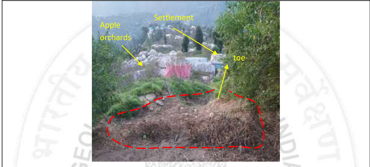
Fig.1. Unstable crown with toe side observed in Leharali slide
