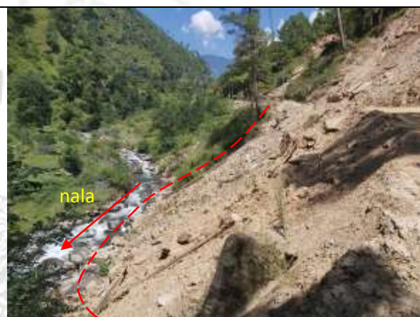
Fig.82. Run off material of slide reaches up to the nala
