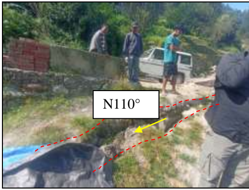
Fig.29; Ground cracks along the lower most road level at Bandal.
