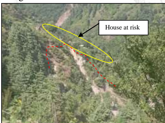
Fig.25; Landslide on right flank slope of the Barauna village.
