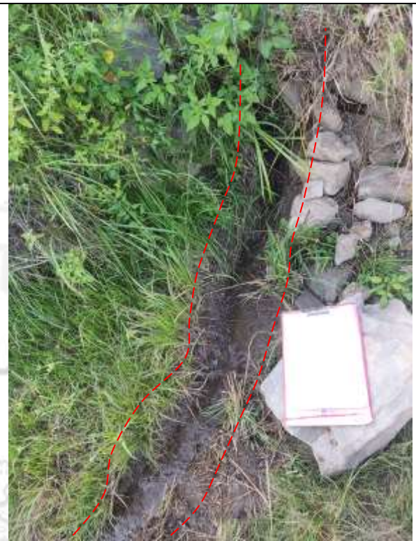
Fig.69. Ground water seepage within the ground crack in the slide area
