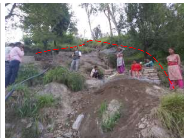
Fig.66. Construction of retaining wall carried out to protect the crown.
