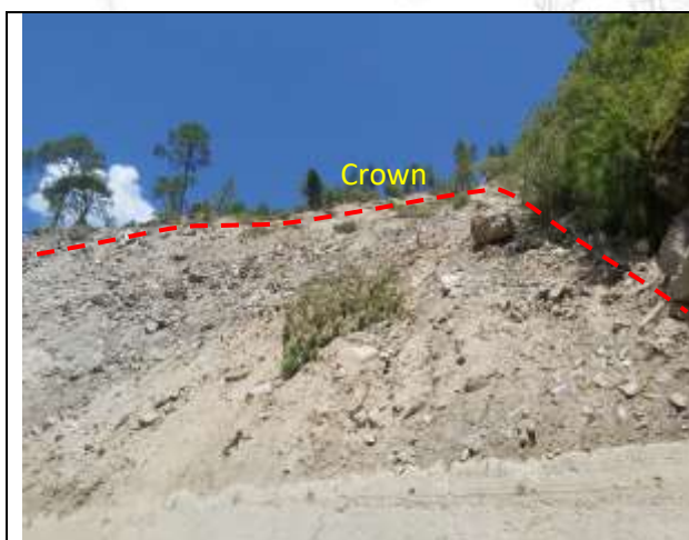
Fig.79. Unstable crown portion of slide
