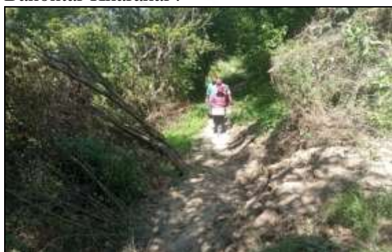
Fig.15; Tilting of trees along the valley side of foot path.
