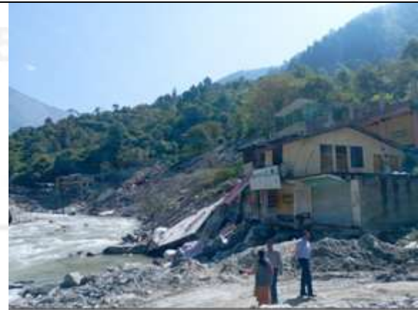
Fig.3. House at risk (left bank of the river)
