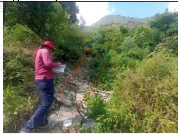
Fig.3. Traverse ground crack on the right flank of landslide.
