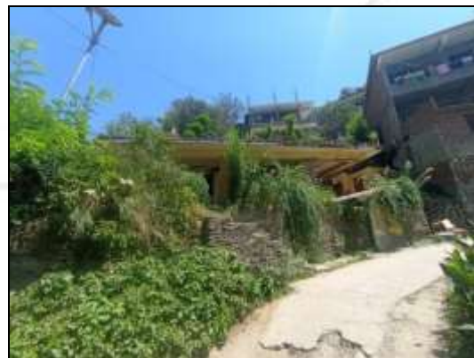
Fig.4; Damaged house at Devdhar village.
