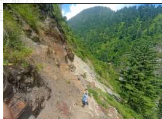
Fig.26 Footpath completely wash out/damaged due to landslide on right flank slope of Barauna village.
