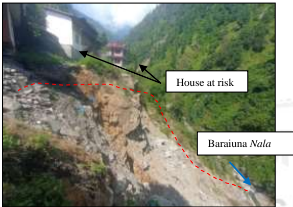
Fig.21; Crown of the slide along steep slope at Barauna village.
