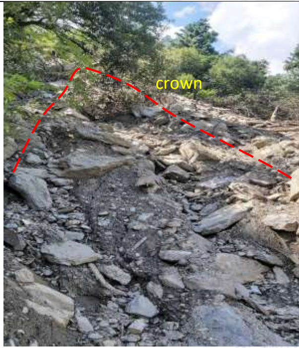
Fig.1. Unstable crown portion of Darsha slide
