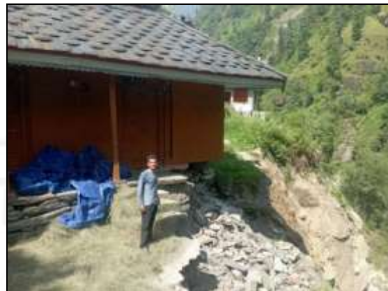
Fig.22; Mandir at risk located on the crown of the slide at Barauna village
