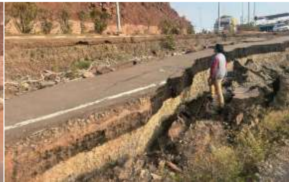
Figure 6 (b) subsidence upto 2 m near Dimple Dhaba.
