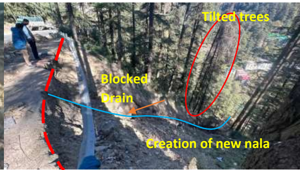
Figure 7 (b) Crown of slide at the road level
