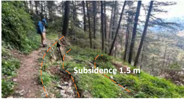
Figure 8 (f) Subsidence at crown by 1.5 m
