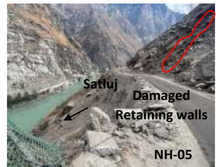
Toe of Nathpa Rock Slide, Kinnaur District, Himachal Pradesh
