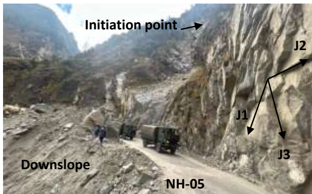
Figure 24(b) Three set of joints of Panvi Bridge Rock Fall, Kinnaur District, Himachal Pradesh
