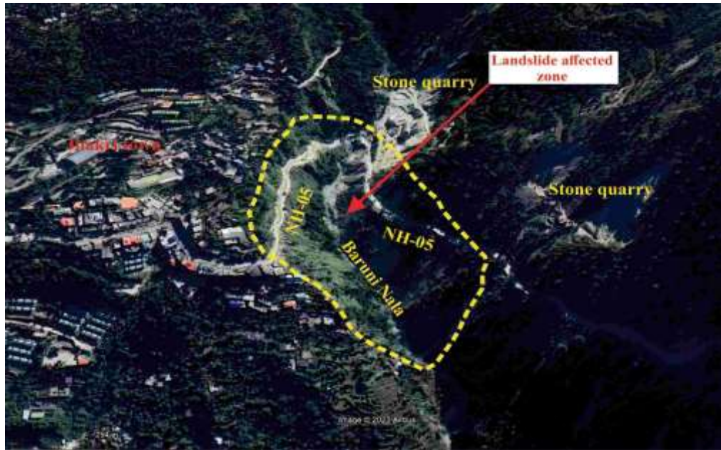
Fig. 21 (i) Google Earth Imagery depicting the location of Barauni Nala Slide Zone
