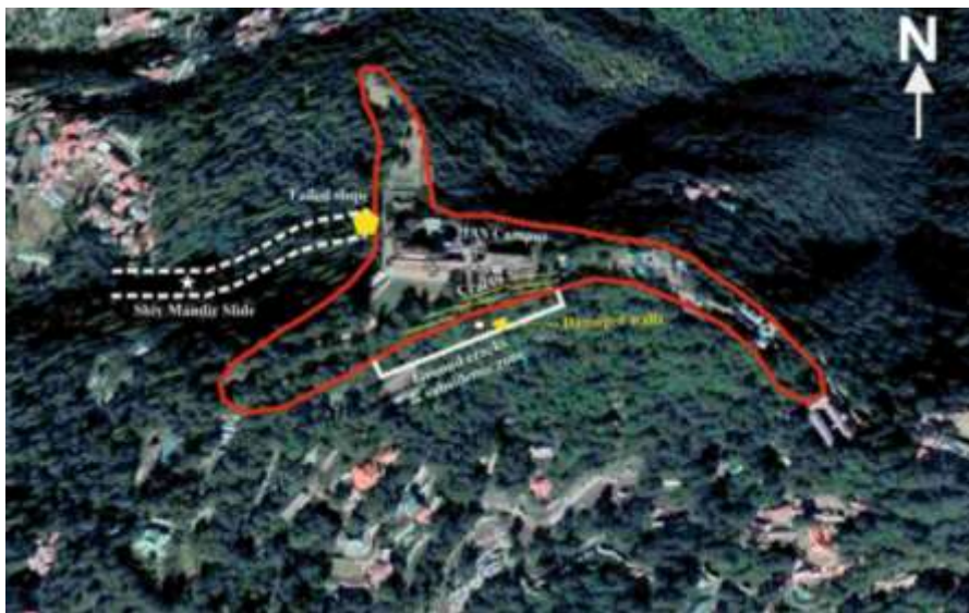
Fig. 10a Google Earth Imagery representing the affected slopes around the IIAS Campus.
