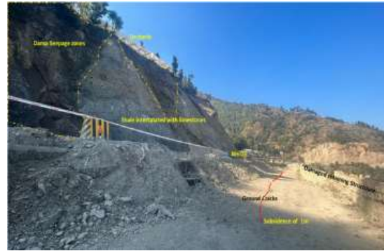
Figure 13 (f) Damp zones and orchards on upslope of Mansar slide
