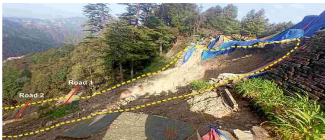
Fig. 10 (g) Slope failure at the western flank of IIAS below which the Shiv Madir Slide had occurred in the month of August 2023.
