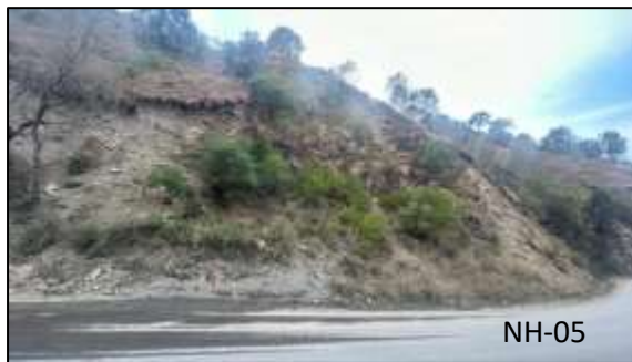
Figure 18 (c) Highly weathered slates of Khamrada Formation of Kullu Group.
