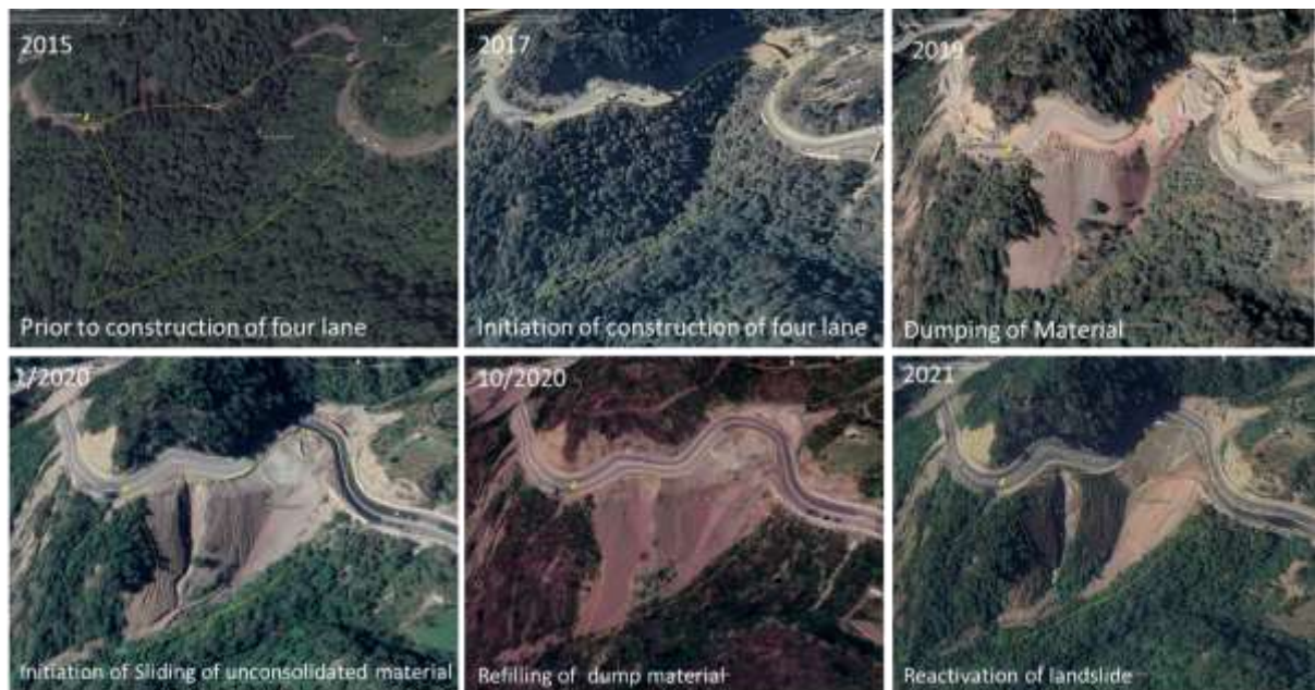
Figure 5 (e) Satellite imagery showing development of the slide by creation of dumping zone along road during construction of the four lane National Highway from 2015 to 2021
