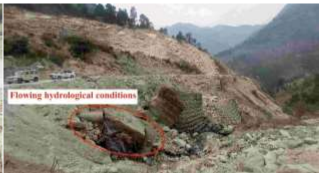
h) Perennial flowing nala across the NH-05
