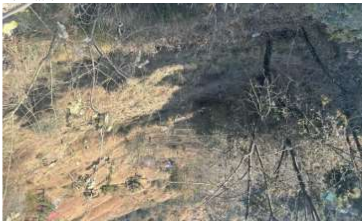
Gentle downslope of slide area having seepage zones.
