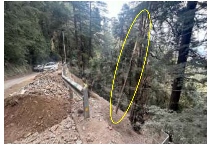
Figure 11(d) Subsidence and tilting of trees observed along road section
