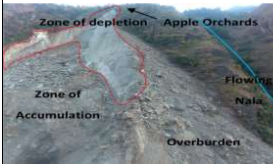
Crown of Nathpa Rock Slide, Kinnaur District, Himachal Pradesh
