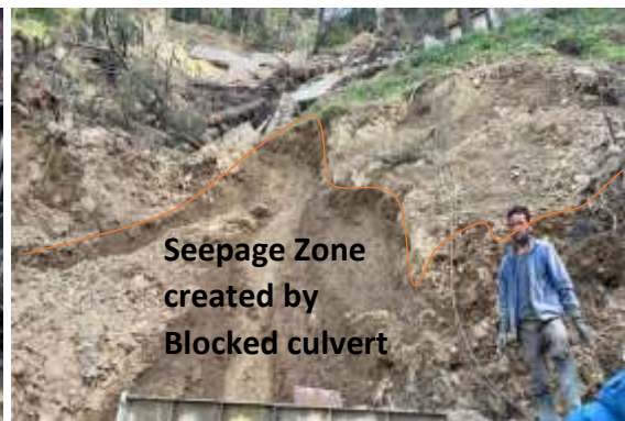
Figure 8 (c) Seepage zones created at sites where culverts have been blocked
