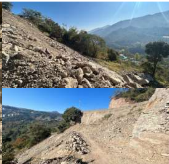
Figure 12 (e) Creeping of trees and bulging of retaining structures
