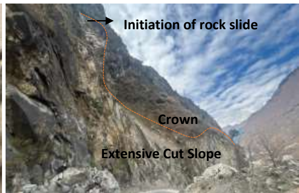
Figure 24(c) ECS at Panvi Bridge Rock Fall, Kinnaur District, Himachal Pradesh
