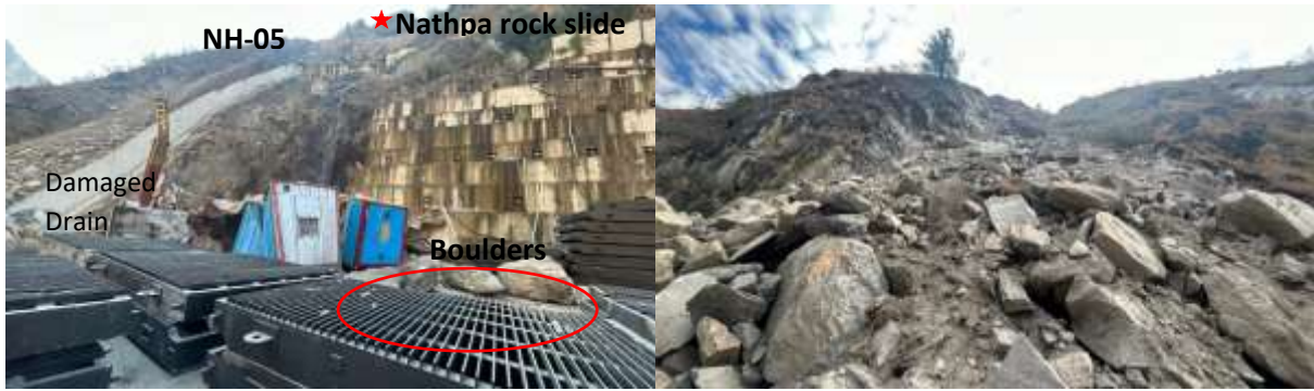
Figure 25(f) Damage to SJVNL dam
