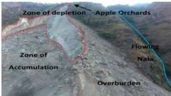
Figure 25(b) Crown of Nathpa Rock Slide, Kinnaur District, Himachal Pradesh
