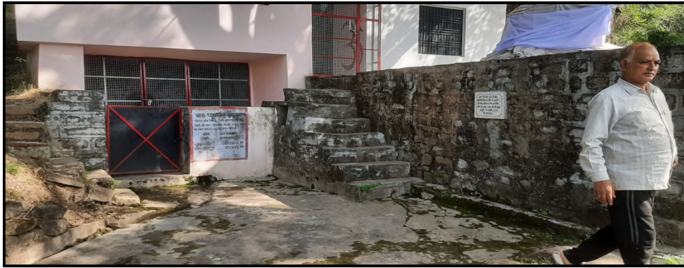
Fig. 26: A natural spring renovated with construction of civil structure/shade around it. Reported minor subsidence within/immediate next to spring premises.
