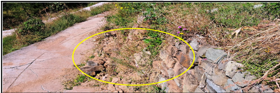
Fig. 18: A minor bund failure in bund wall of agriculture terraces at some distance away from Mahila Mandal Complex (Note the yellow oval).
