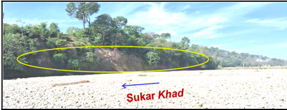
Fig. 10: Weathered and jointed rock mass outcrop exposed towards u/s end of the major gully, as observed along right bank of Sukar Khad (Note the Yellow oval).
