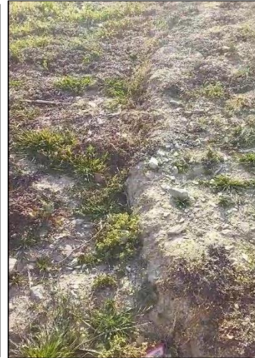
Cracks developed due to settlement in field.
