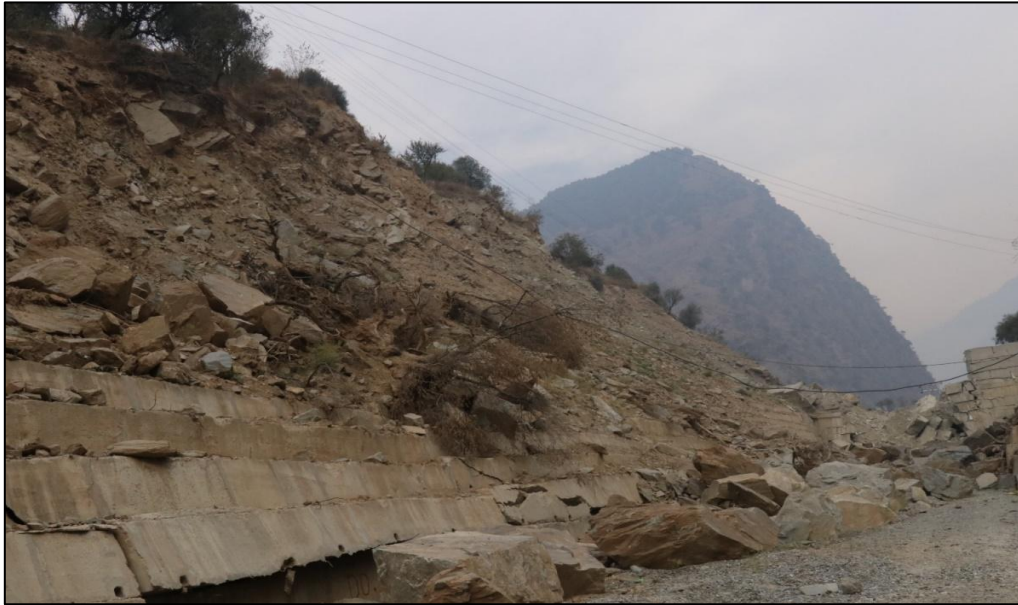
Landslide at site 2 (left view).
