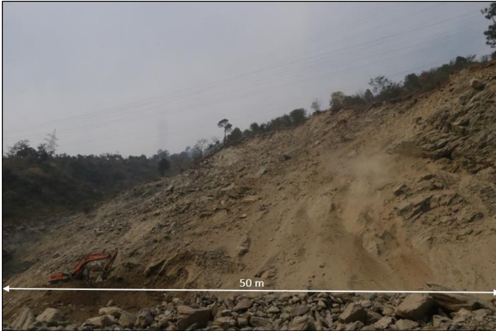
Landslide at Site 1.
