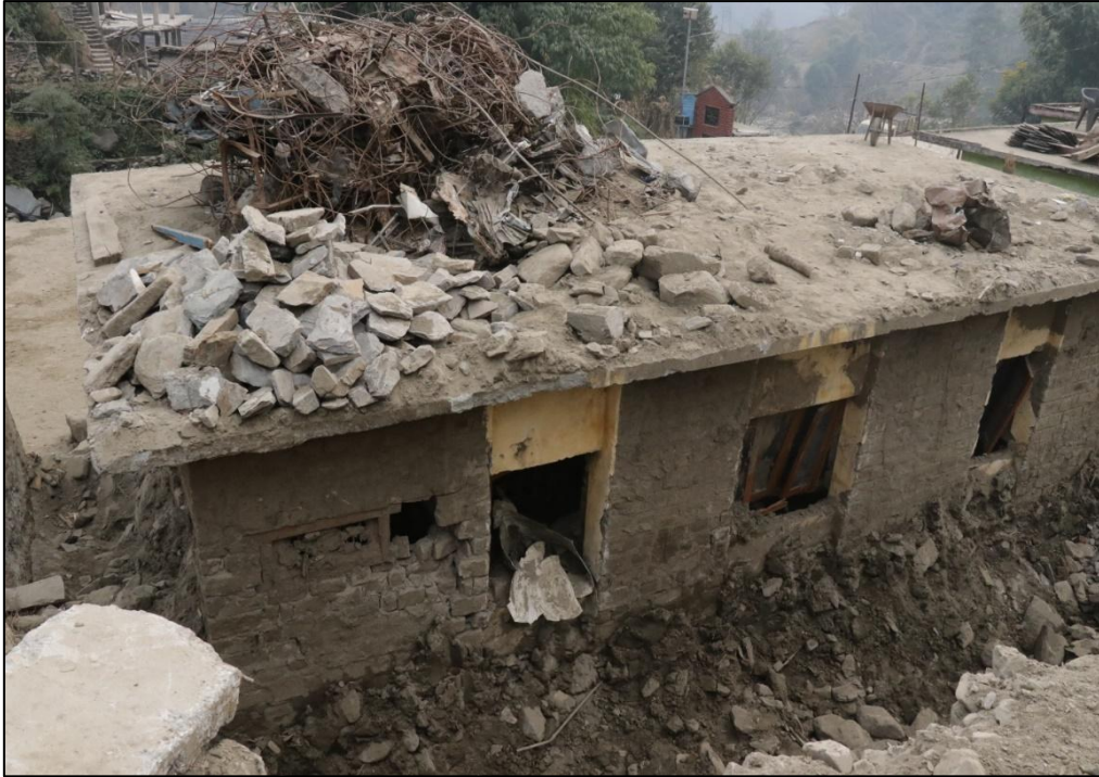
Damaged residential building.
