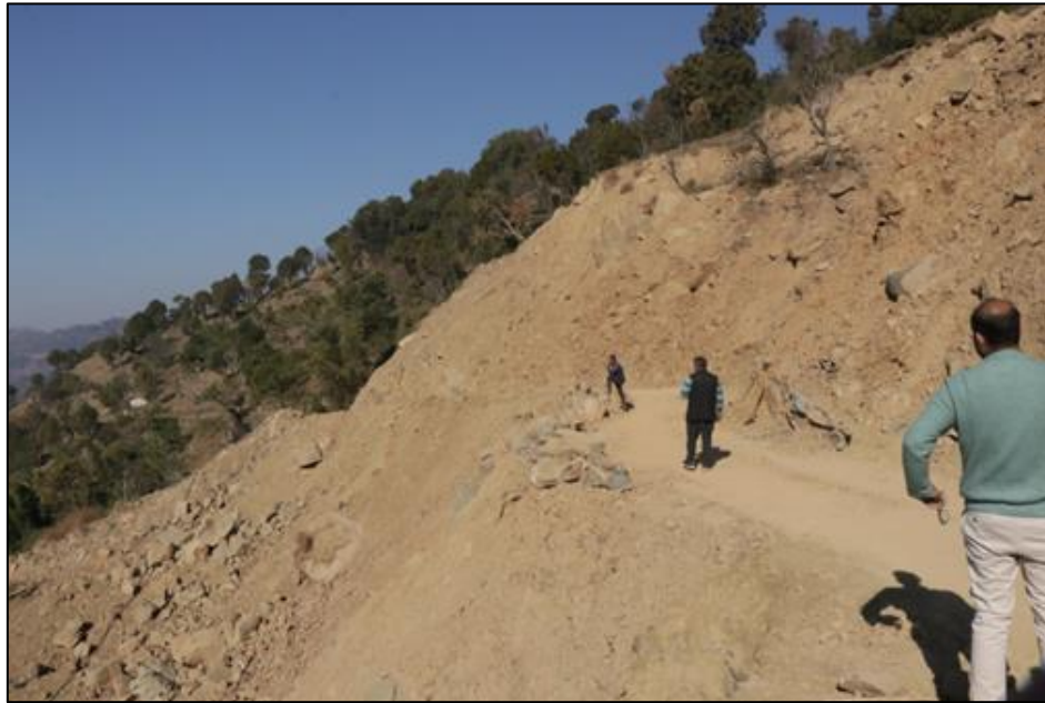
The temporary road restored in December 2023.
