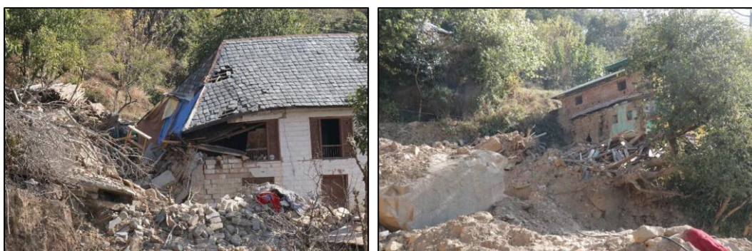
Completely damaged households.
