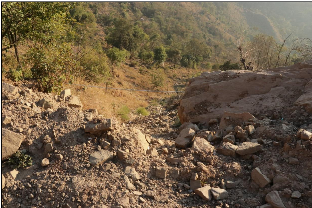
Landslide site below road.
