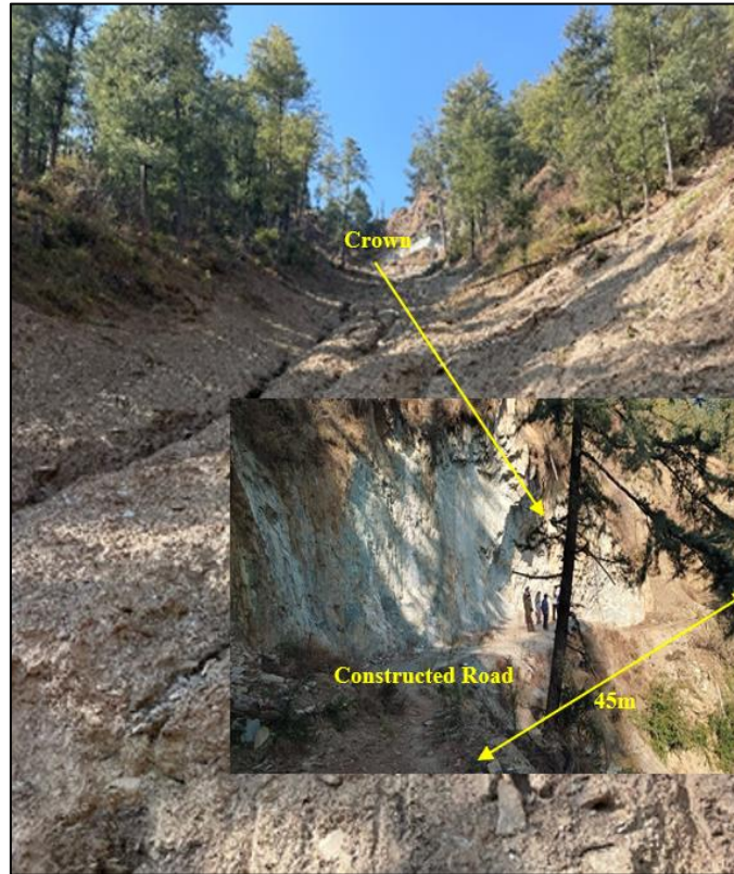
Crown of landslide.
