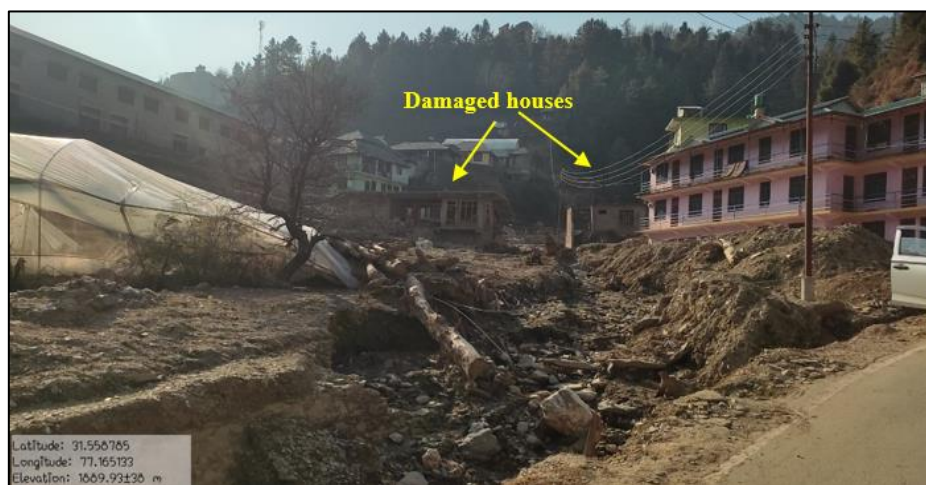
Damages houses in the main market due to debris flow.
