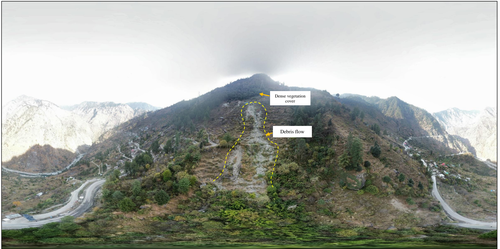
Fig. 21 A panoramic view of Shilani landslide, Nathpa, Kinnaur district, HP
