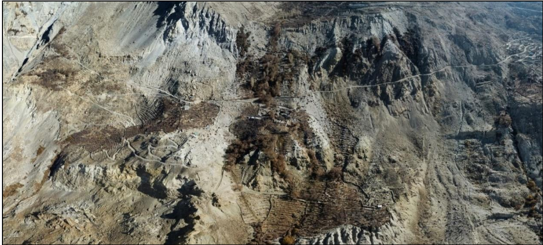
Fig. 6 Field photograph of Yangthang landslide, Kinnaur District, HP
