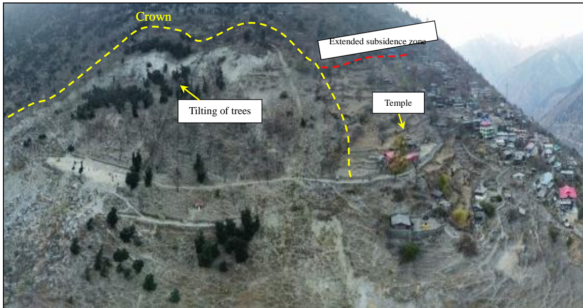
Fig. 12 Field photograph of the Brua landslide using UAV survey.
