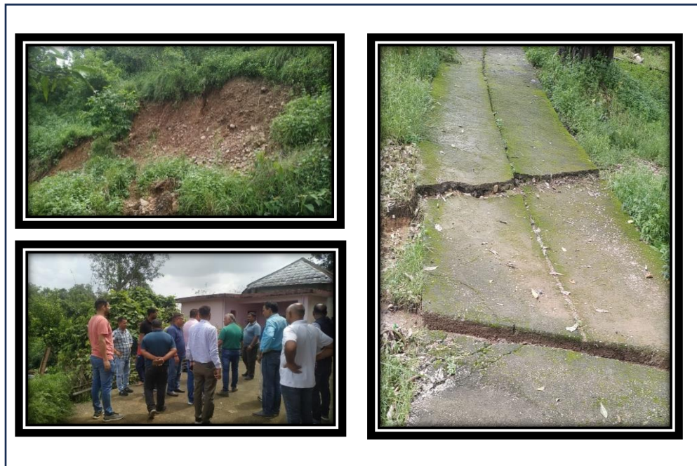
Fig. 7 Shows the scarp in the second slide zones and house with in the slide zone.
