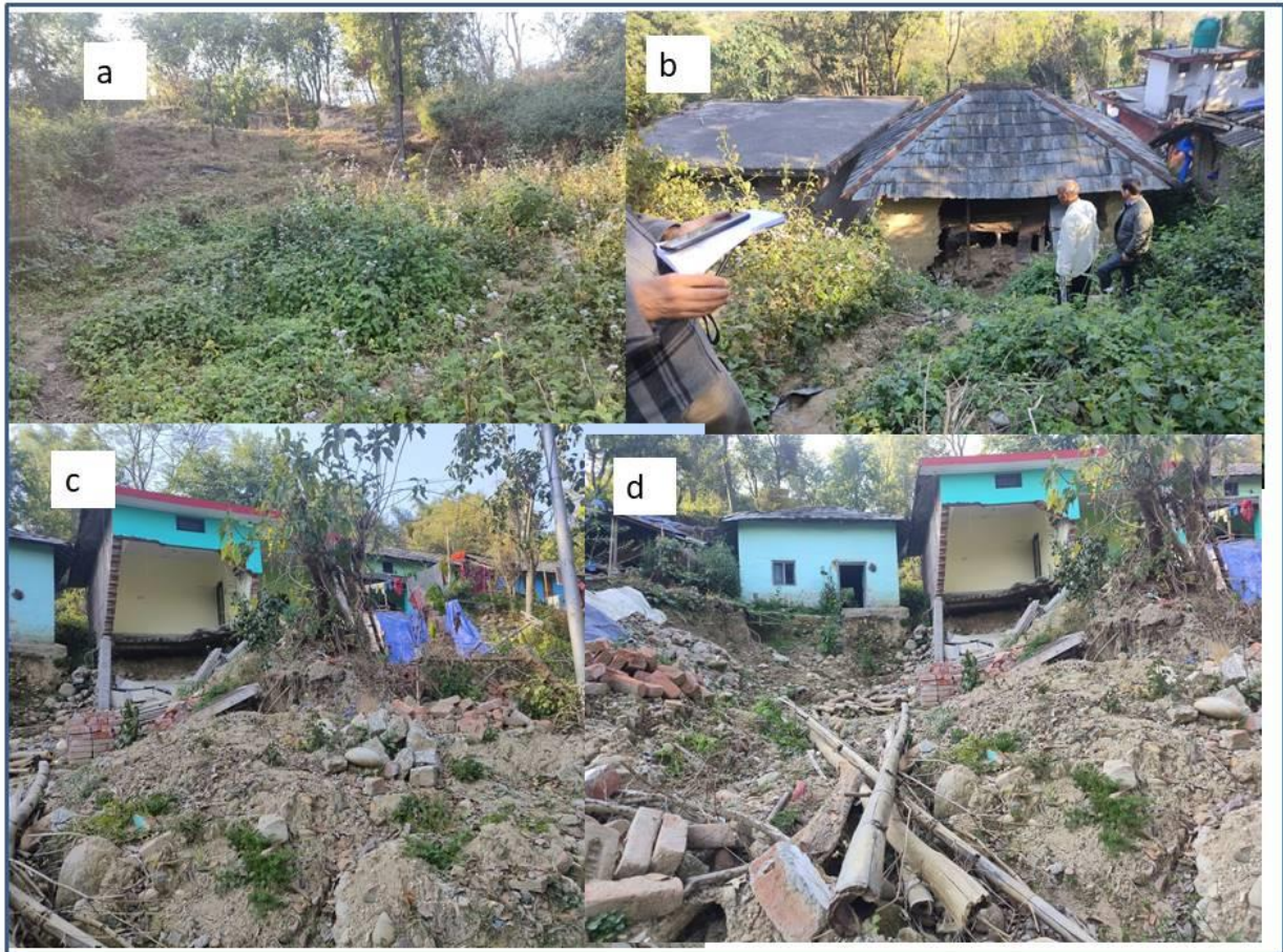
Fig. 12 Shows the damage cause to the houses in Gurthali village a) shows the slope angle and ridge from where water came after heavy rain fall b) the back side of the houses where water was blocked, the mud houses could sustain the pressure but concrete houses could not sustain the water pressure due to soft storey at the bottom c and d) damage cause especially removal of lower portion of concrete house and havoc caused by blocked water in the down side agricultural land in front of the houses.
