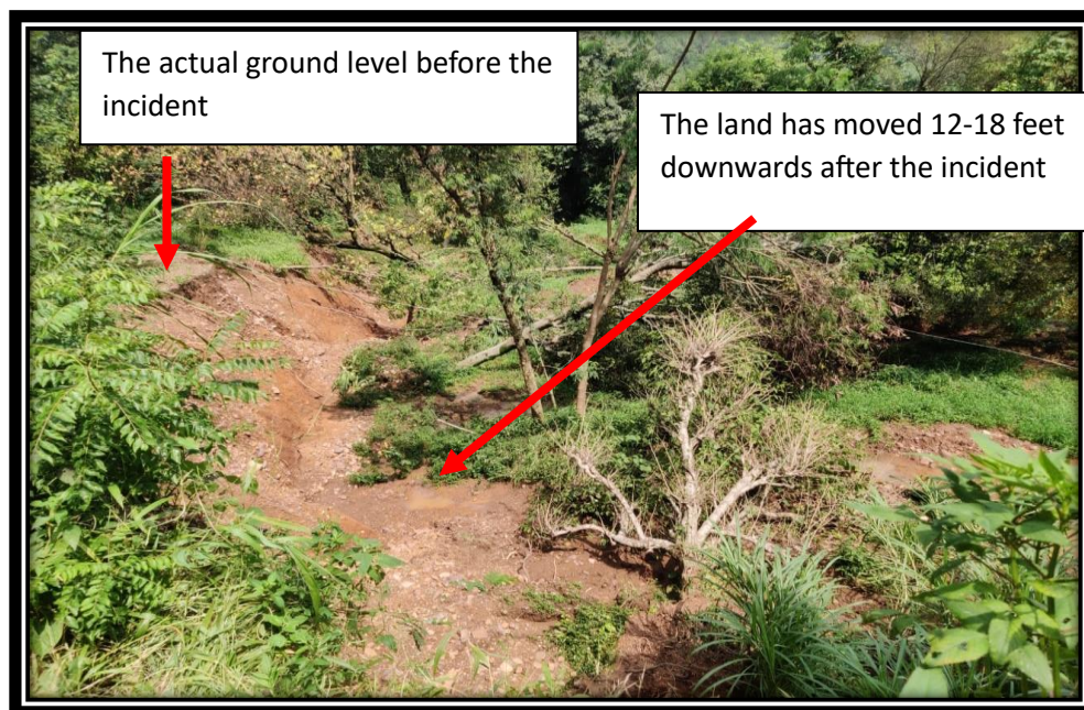
Fig. 10. Showing development of wide fissures in the agricultural land with titling of trees indicating deeper slip surface.
