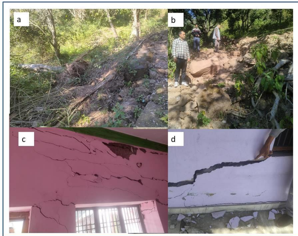
Fig.14 Uprooting of trees and displacements of roads and it's downwards movement suggesting deeper slip surface b) Development of cracks in walls suggesting movement direction
