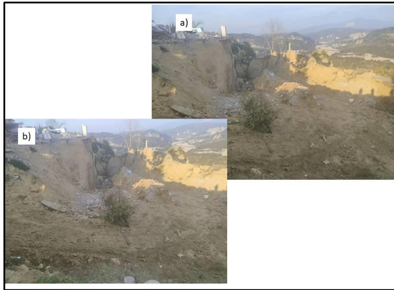
Fig. 15 Sandstone rocks get displaced along the fissure and caused disastrous impact in the village. All houses located on this portion of the sheet like rock also displaced.
