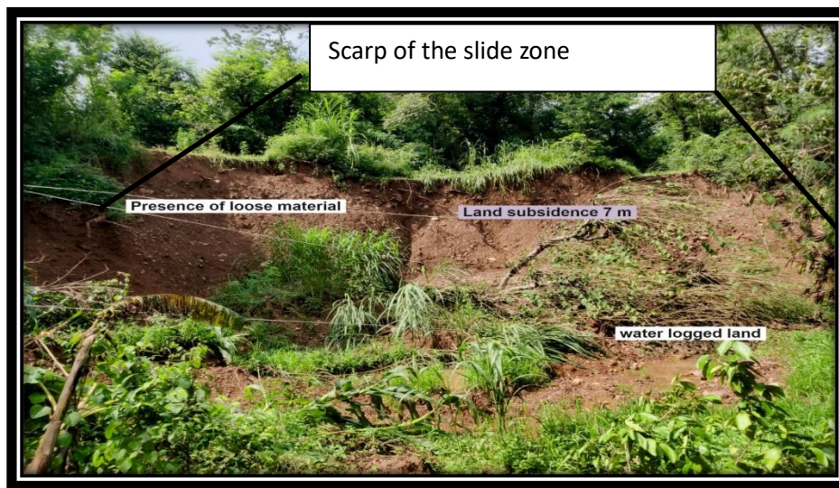
Fig 9 showing full panoramic view of landslide event and subsequent land subsidence at site no 3
