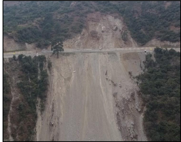
Fig. 14. Loose debris slide material
