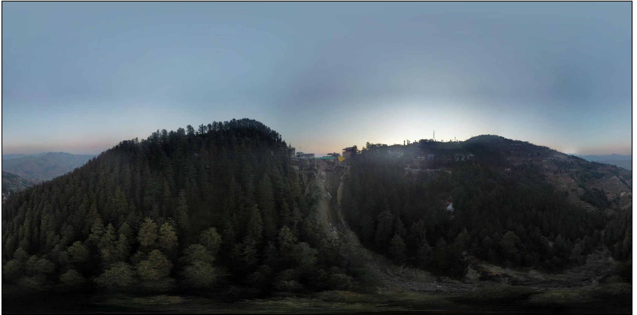
Fig. 51 A panoramic view of Rahighat Kyartu Link Road, Theog landslide site, Shimla district
