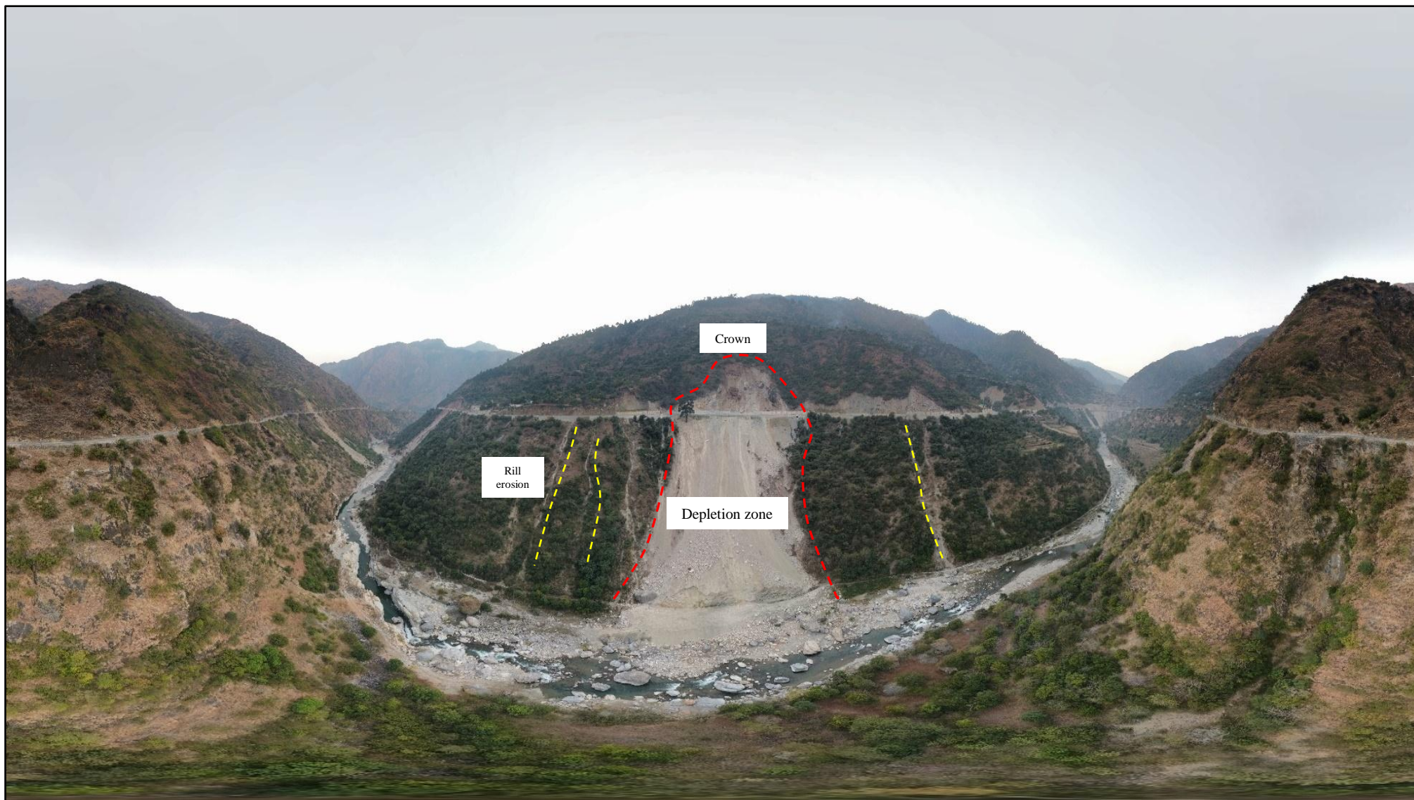
Fig. 10 A panoramic view of NH-707B landslide site near Fedzipul, Chopal, Shimla district
