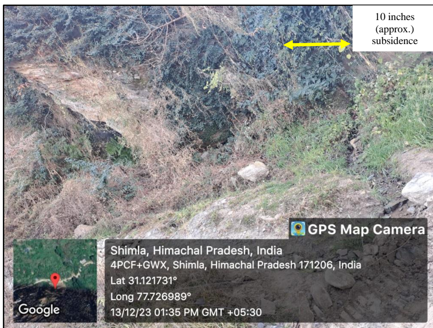
Fig. 39. Cracks in Apple Orchards Caused by Land Subsidence
