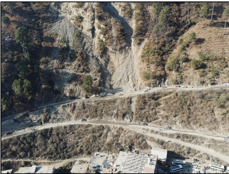
Fig. 25. Structures likely to be affected by Landslide
