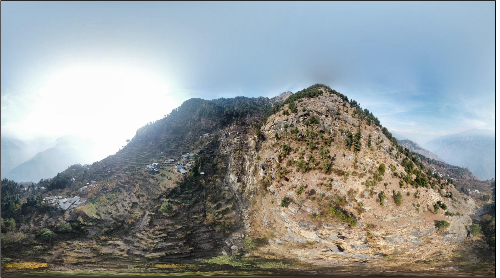
Fig. 71. A panoramic view of Kot, Rampur landslide site, Shimla district
