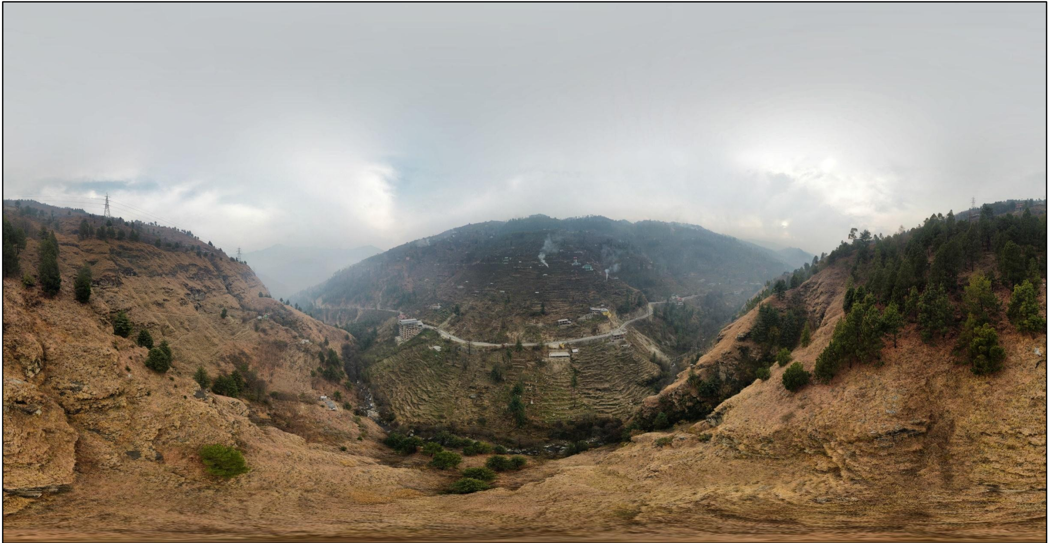
Fig. 35. A panoramic view of Ploutidhar, Jubbal landslide site, Shimla district
