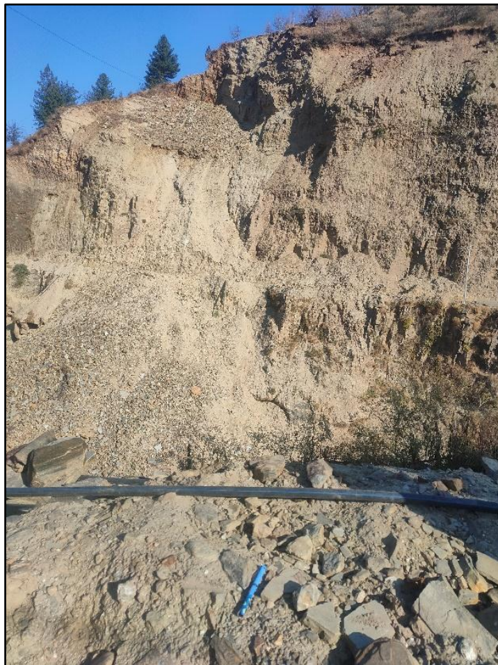
Fig. 48. Titrikyar landslide depicting the loose debris slide
