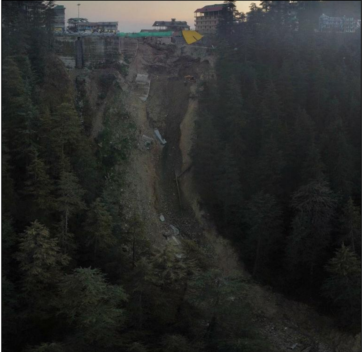
Fig. 52. Field photograph of Rahighat Kyartu Link Road, Theog landslide site, Shimla
