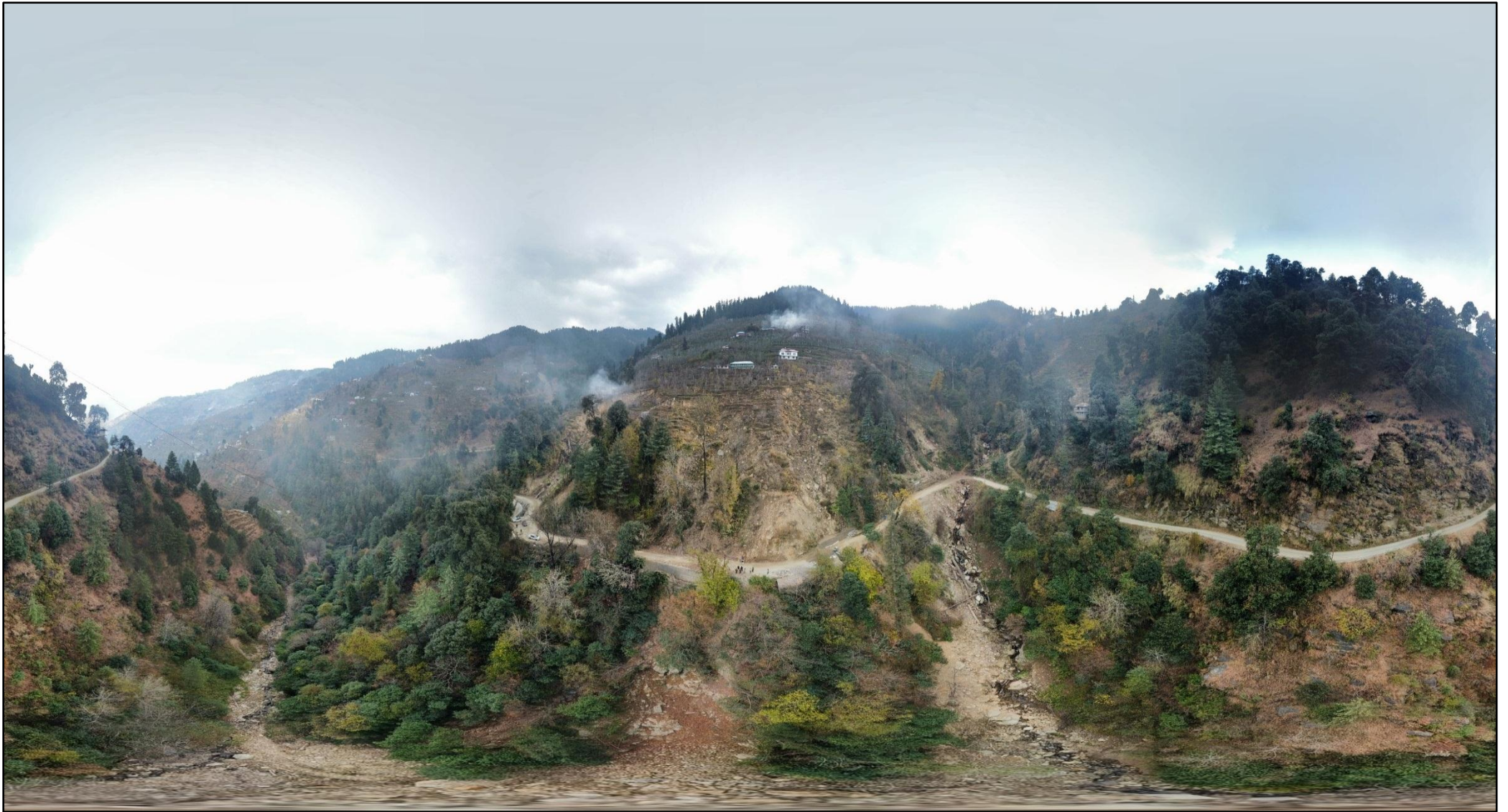
Fig. 55. A panoramic view of Marni-Kanhar, Kumarsain landslide site, Shimla district
