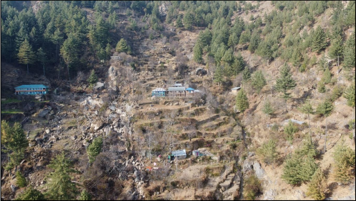
Fig. 72. Field photograph showing sinking area and houses at risk
