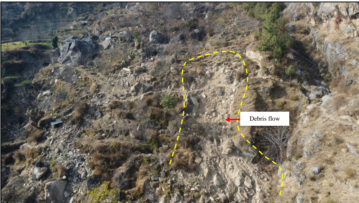
Fig. 73. Debris runout material illustrates the extent of the landslide's impact
