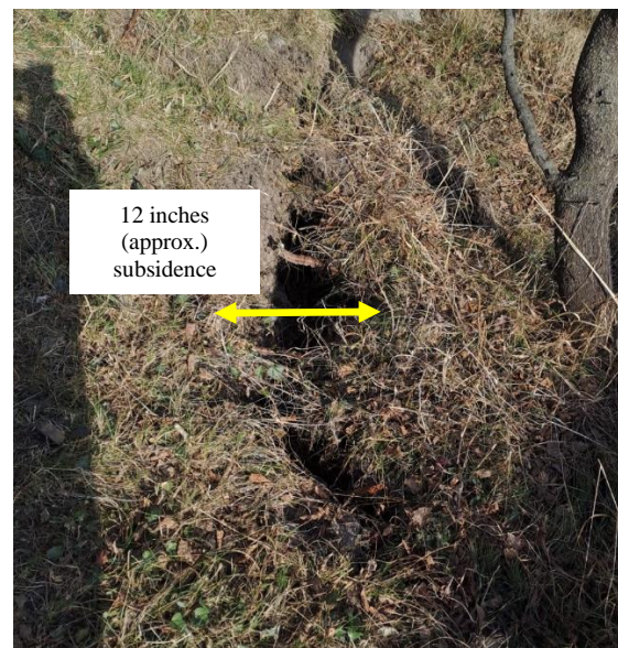
Fig. 75. Cracks in apple orchards due to subsidence
