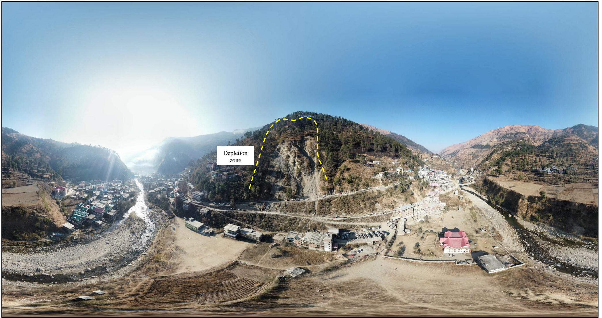
Fig. 23 A panoramic view of PWD rest house, Nerwa landslide site, Shimla district
