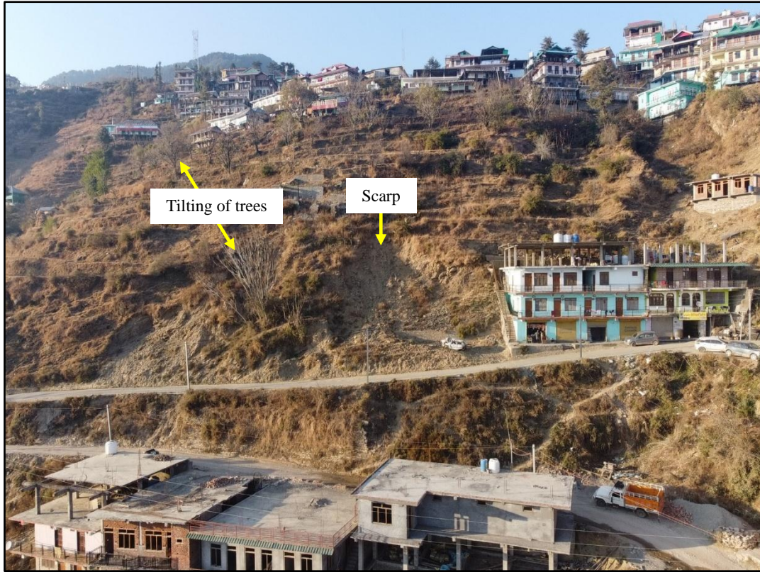
Fig. 29. Structures and agricultural land affected due to landslide
