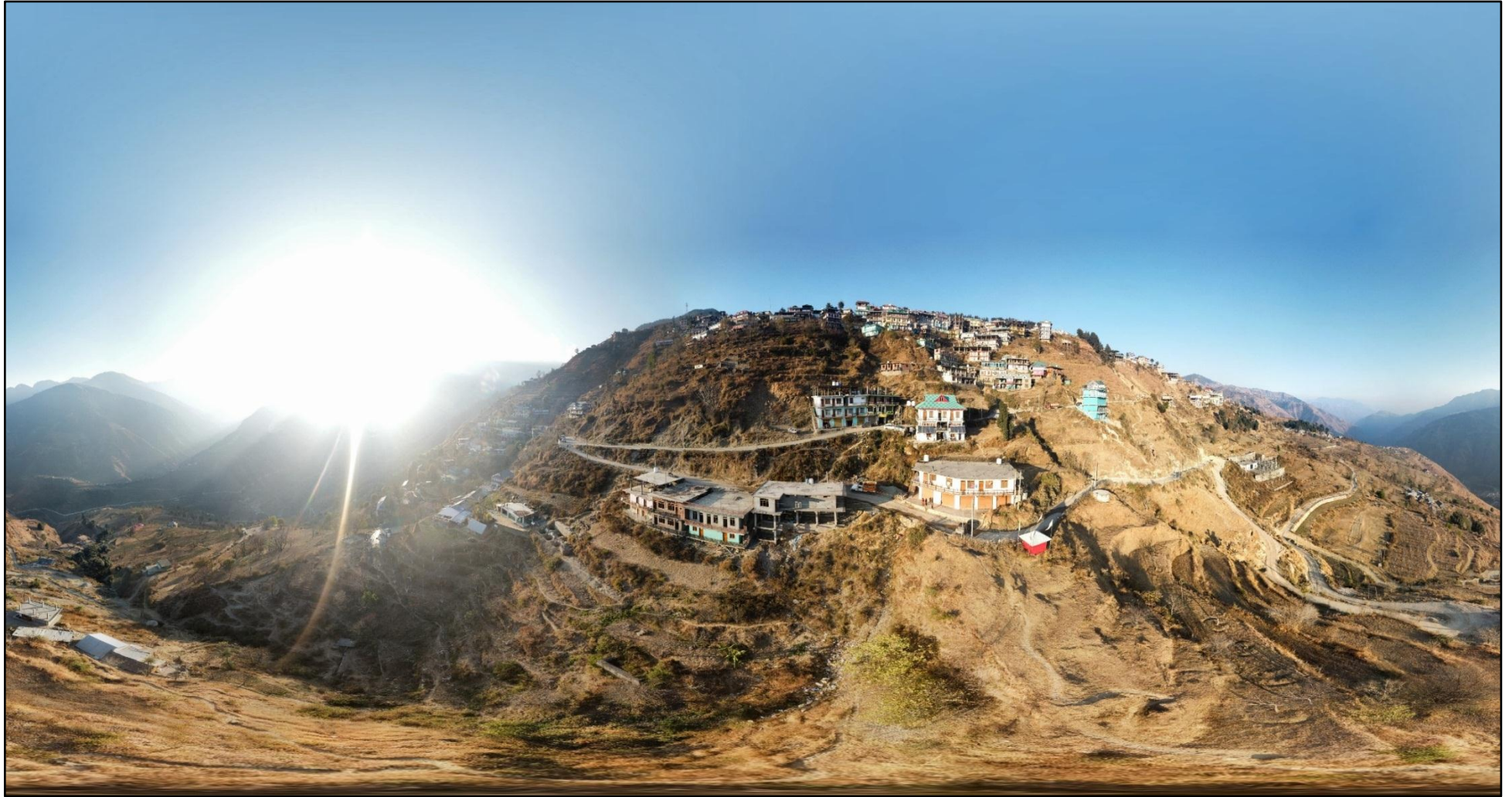
Fig. 28. A panoramic view of Near Police Station, Kupvi landslide site, Shimla district
