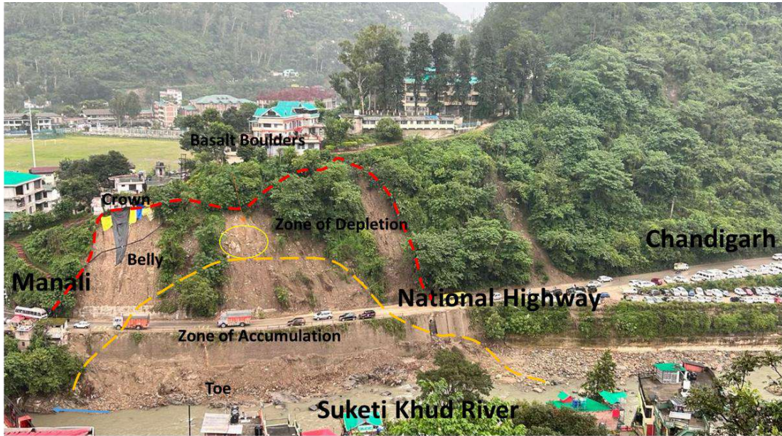
Figure 5.1 Morphometry of the Kanganidhar Landslide.
