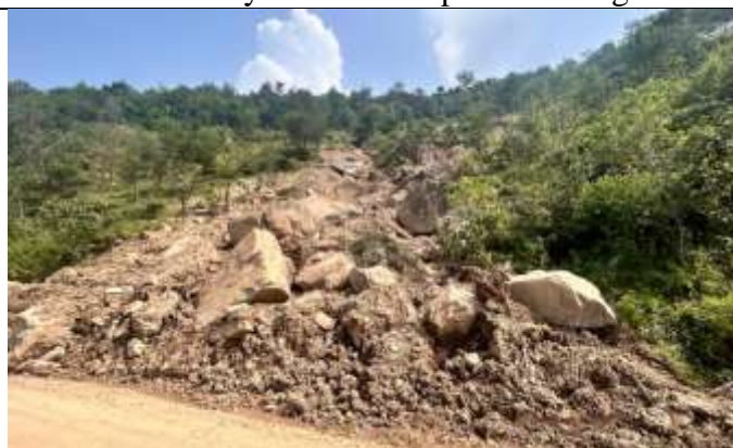
Figure 10 (e) Landslide at Badiyar village, Dharampur, Mandi charged with heavy boulders
