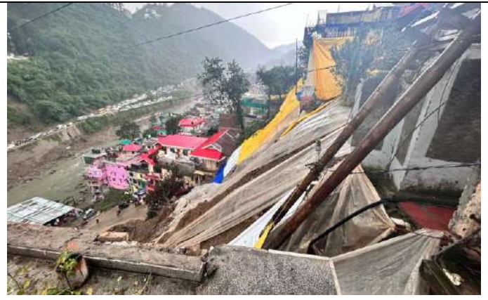
Figure 4.4 Uprooted electric poles and trees due to slide
