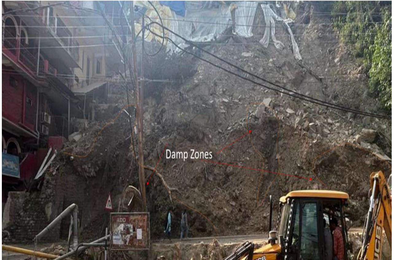
Figure 4.22 Damp Zones at the toe portion of the slide
