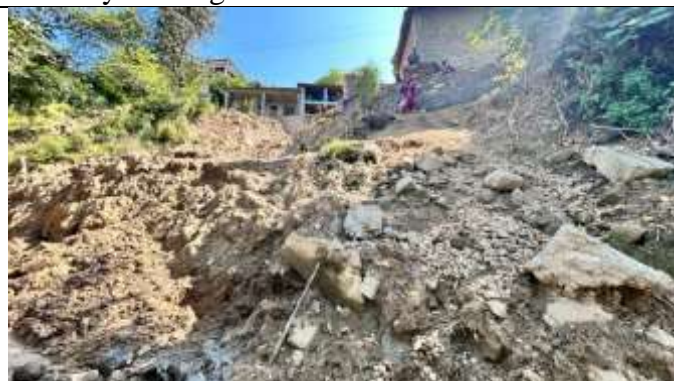
Figure 10 (t) Debris slide observed at Baral village, Mandi district, HP
