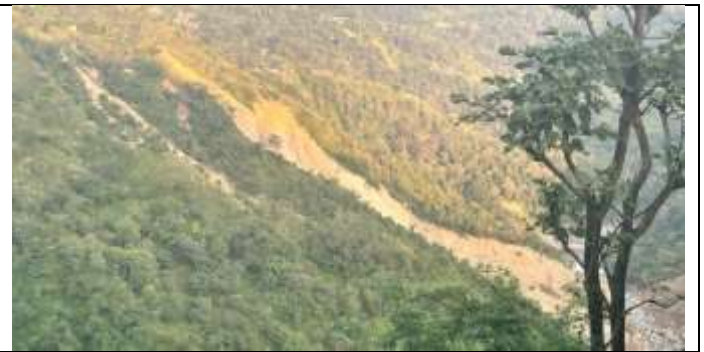
Figure 10 (b) Prospective view of Mandap landslide, Dharampur, Mandi
