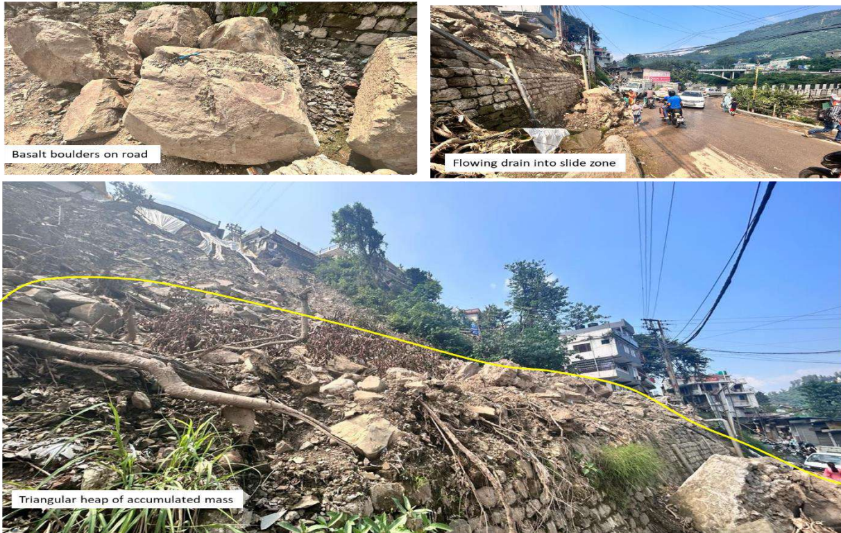
Figure 4.18 a) Basalt boulders along the Mangwai road at Toe b) Flowing drain into the slided zone c) Accumulated material at the toe of Tarna hill slide
