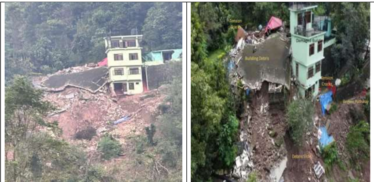
Figure 6: (b) Prospective view of the slide near Circuit house, Mandi District, Himachal Pradesh
