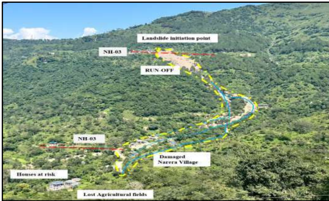
Figure 9 (a) Prospective view of the Cloud burst triggered debris slide, Narera Village, Dharampur, Mandi District, Himachal Pradesh.
