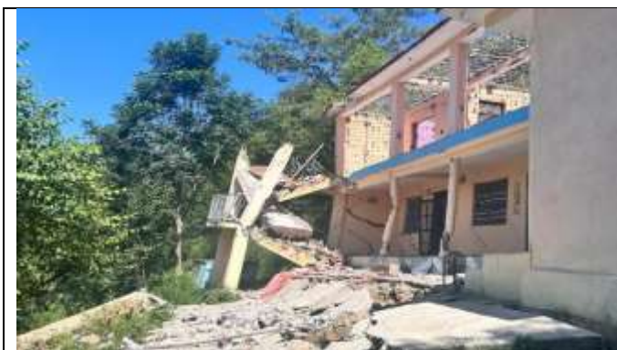
Figure 10 (w) Collapsed house at Barouti Village, Mandi district, HP
