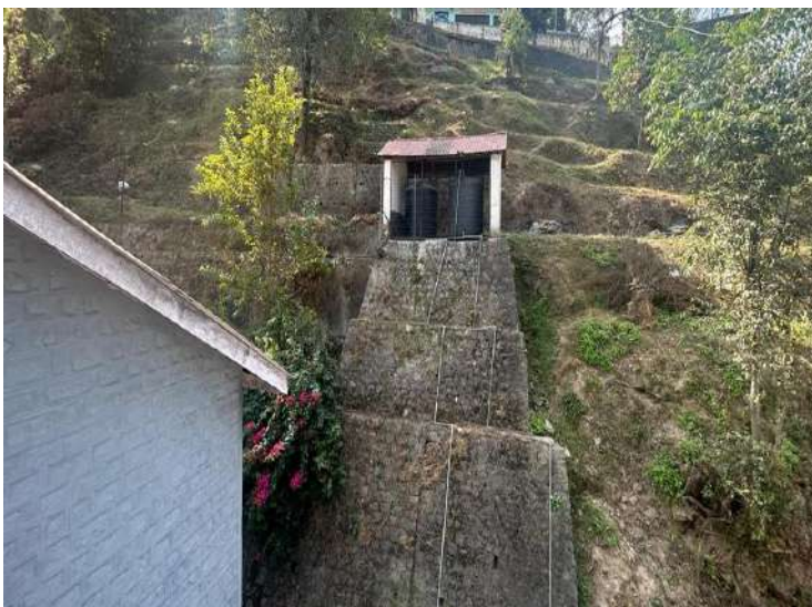
Figure 4.15 The terraced land situated above crown serving for cultivation and settlement purposes
