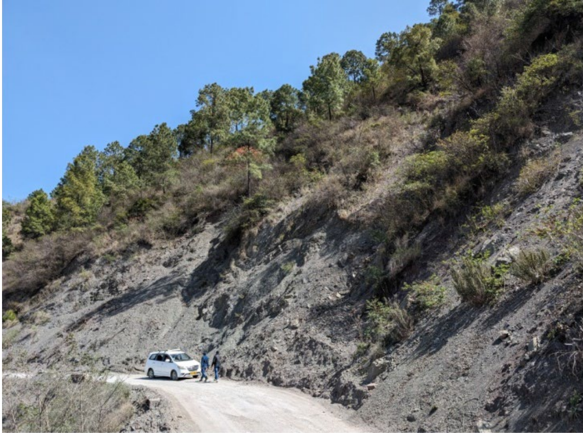
Fig. 2 Debris slide near Chakki Mod, where the damage to the road was marked.
