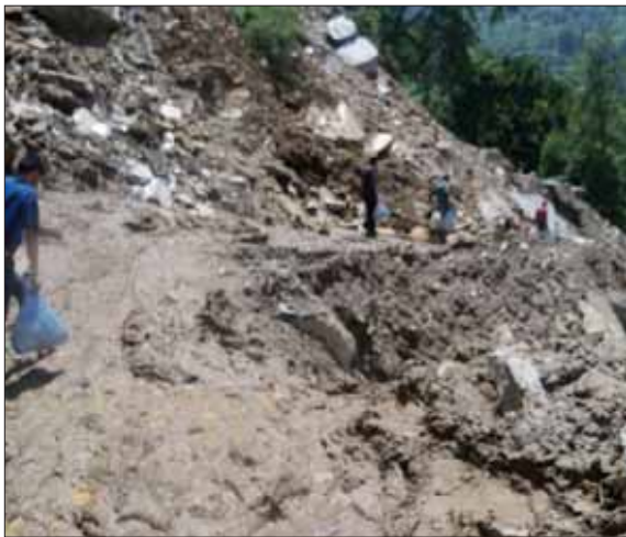
Composite Landslide at Phata, 6 km for Guptkashi
