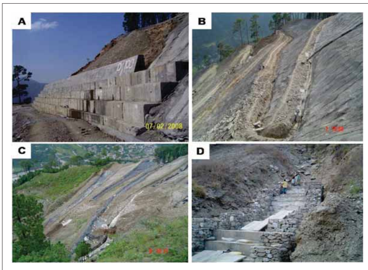
Fig. 3.26 Slope stabilisation measures used in Varunavat Parwat landslides: (A) stabilisation of failed slope by Concrete Cladding; (B) stabilisation of rocky slopes; (C) stabilisation of overburden mass by geo-net below El. 1640 m; and (D) channelisation of chute.
