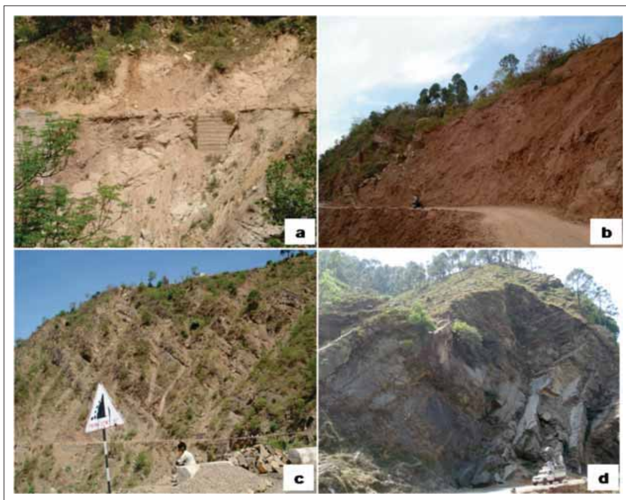
Fig. 4.5. Major landslide along Kangra- Dharmshala-Sihunta-Dalhousie road: (a) debris slide near Sihunta, (b) debris slide zone at 6 km Kakira, (c) rock fall zone near Bakloh junction and (d) wedge failure before Banikhet bridge.
