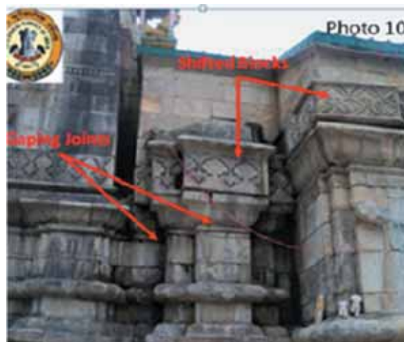
Shifting of blocks of pillars
