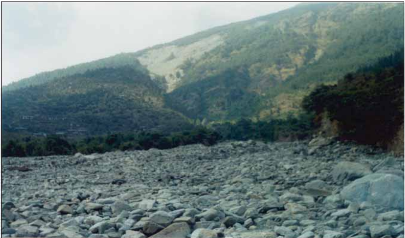
Fig. 3.4. Major rock slide and resulted debris fan on left bank of Badiyar gad (slide no. 14, Table 3.2).
