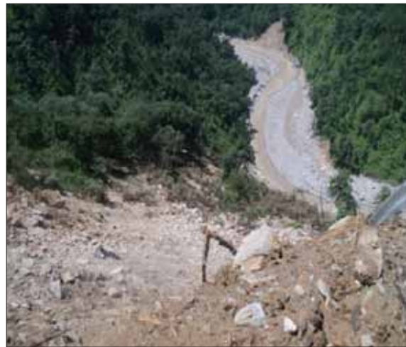
Too Erosion by Mandakini, Phata Landslide
