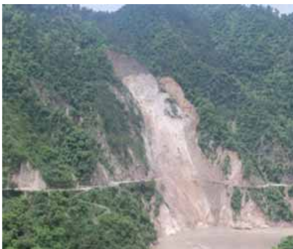
Sirohbagar (Kaliyasaur) Landslide near Srinagar (Pauri Garhwal)
