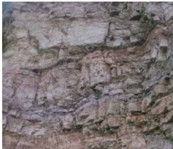
Quartzites of Garhwal Group at Sirohbagar (Kaliyasaur) Landslide
