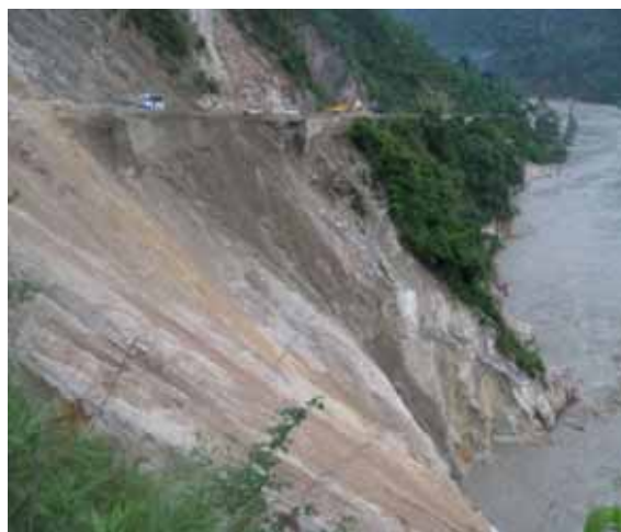
Lower part of Sirohbagar (Kaliyasaur) Landslide near Srinagar (Pauri Garhwal)
