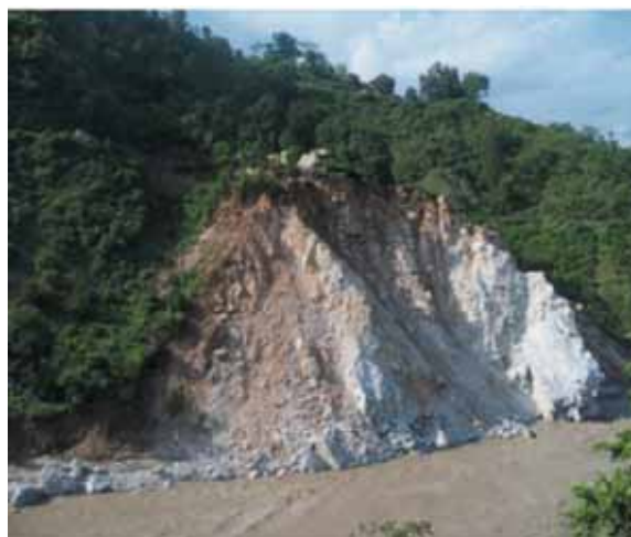
Failure by toe erosion in Terrace involving River Borne Material (RBM)
