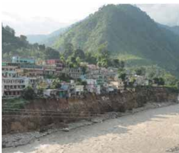
Toe erosion by Mandakini on the right bank below Sumari - Bharsaar village
