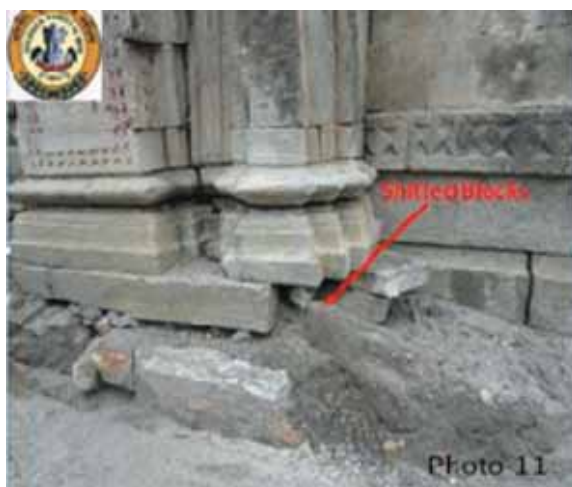
Dislodgement of blocks from the basal part of the temple
