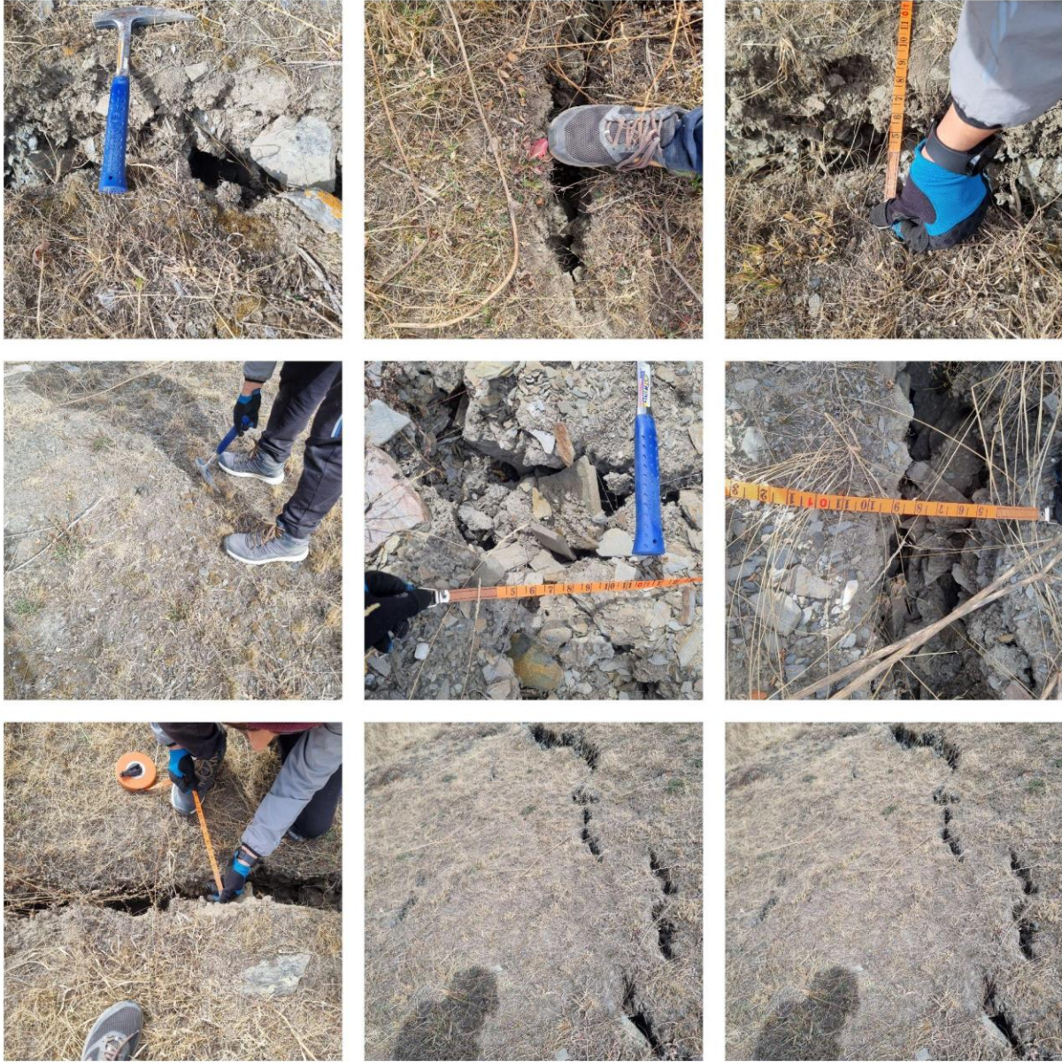
Figure 6: Field Photograph of the cracks observed in the agricultural field
