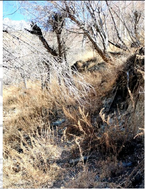
Fig. 23: Ground subsidence together with tilting of trees observed above the crown portion of active slide 1.
