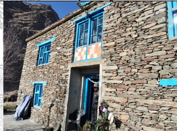
Fig. 13: Two storeyed house made up of local rocks and mud as cementing materials.
