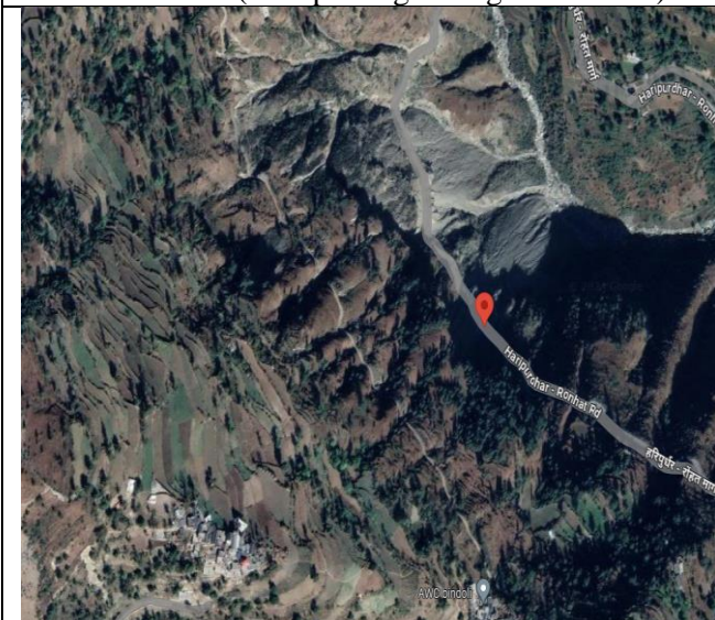
Bindoli site, Ajroli Panchayat, Shillai Subdivision (road section passing through slide & habitation)
