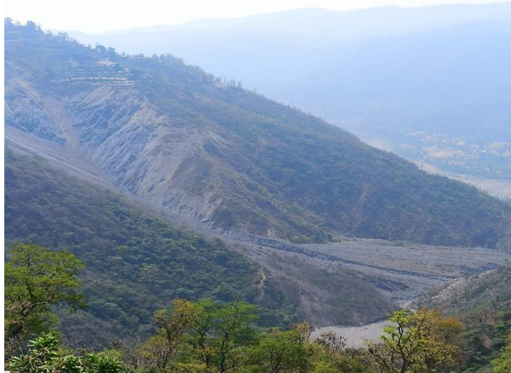
Fig. 6 Large volume of debris material may cause blocking and damming of water below the hill and may contribute to debris flow
