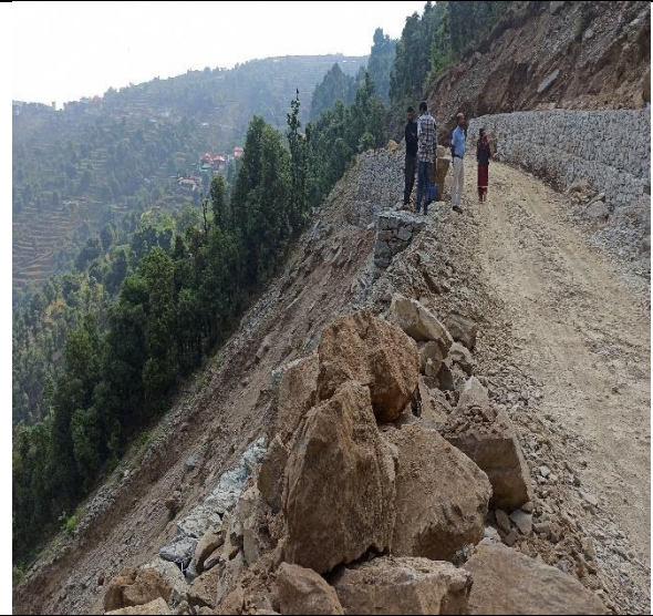
Fig. 2 Debris material and loose boulders indicate debris flow and rock fall potential
