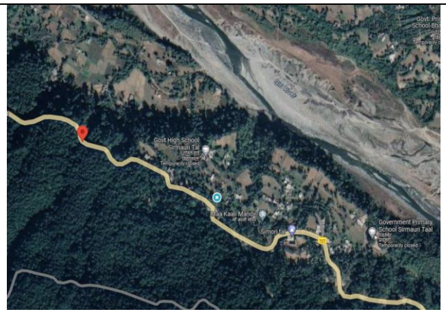
Katchi Dhang NH-707 site, Village Sirmauri Tal, Paonta Sahib Subdivision (Chainage km 14+165), instability in major road passing through slide
