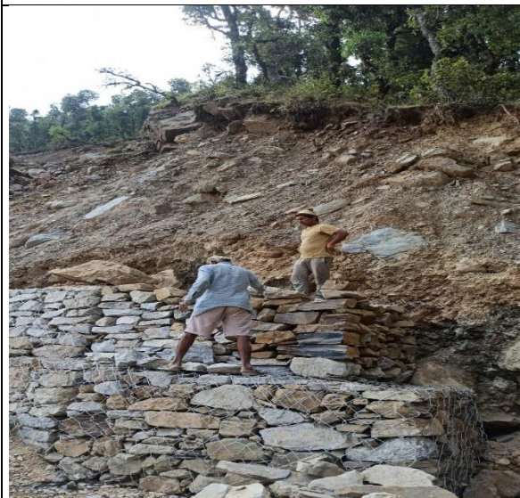
Fig. 3 Strata consists of debris material underlain by disintegrated rock mass
