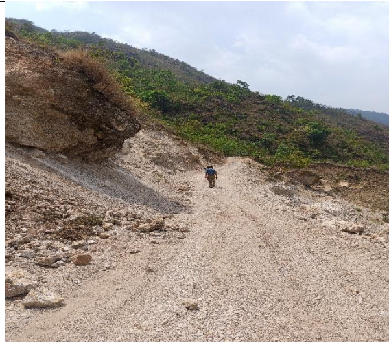
Fig. 4 Slide obstructing major district road
