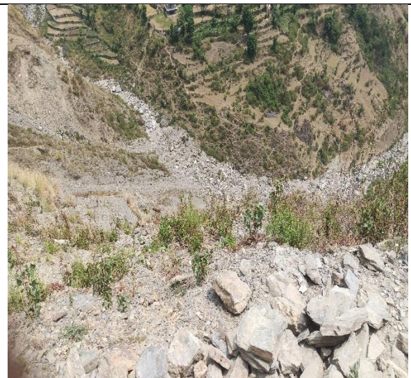
Fig. 2 Debris material visible on valley side slope along with seasonal stream
