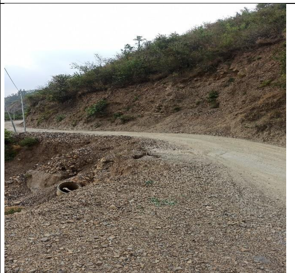
Fig. 2 Debris material on slope and inclined tower indicating ground movement
