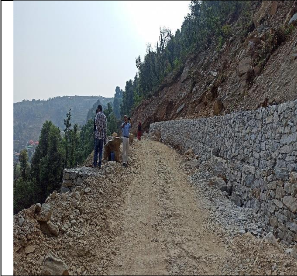
Fig. 1 District road passing through the slide zone
