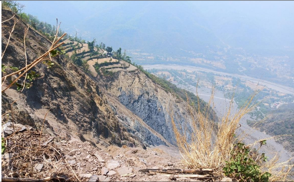
Fig. 1 Residential buildings and agriculture on the top of landslide
