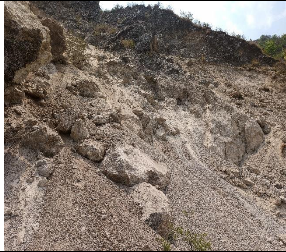
Fig. 2 Significant rock fall potential on hill side slope
