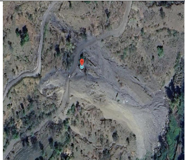
Harlog site, Bhujond panchayat, Sangrah Subdivision (road section passing through slide)
