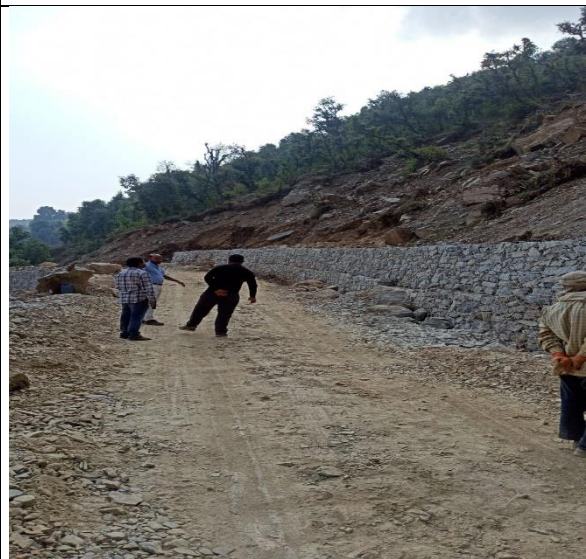
Fig. 4 Ongoing slope mitigation work
