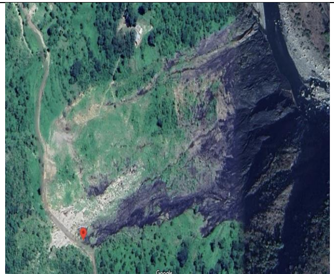
Lana Rauna site, Neri Nawar Panchayat, Pachhad Subdivision (road passing through slide zone)
