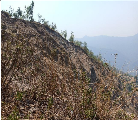
Fig. 2 Disintegrated rock mass and soil fines with boulders in strata
