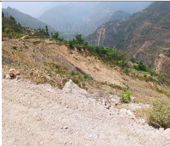
Fig. 6 Instability on valley side affecting infrastructure
