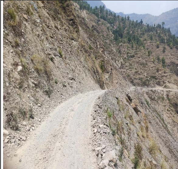
Fig. 3 Debris material underlain with highly disintegrated rock mass
