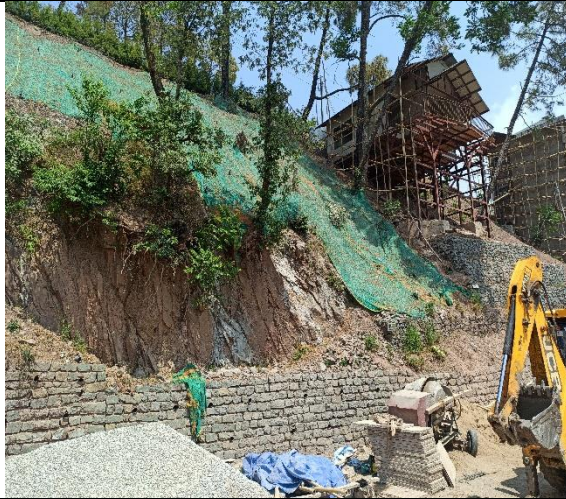
Fig. 1 Mitigation work on hill side slope of the property
