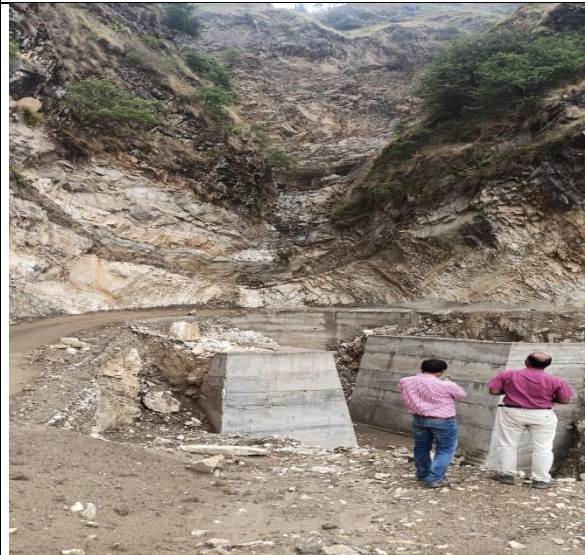
Fig. 4 Bridge bypass under construction at site
