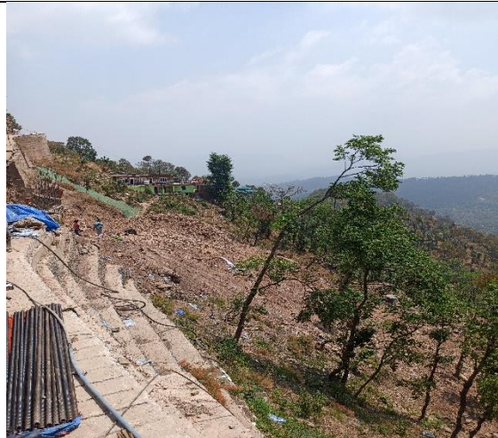
Fig. 3 Buildings present on fringes of slope
