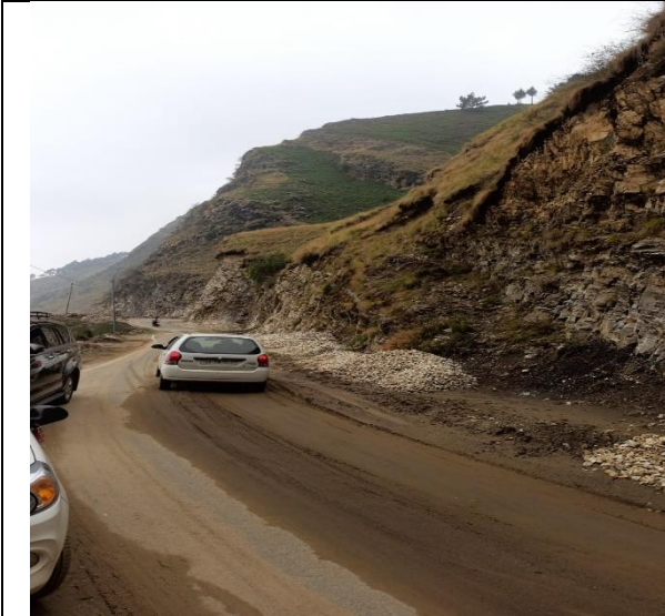
Fig. 1 Major road passing through the slide zone
