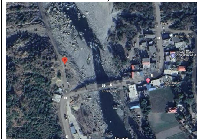
Chunnar site, Neri Nawar panchayat, Pachhad subdivision (road passing through slide zone)
