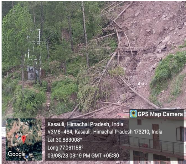
Figure 6 Location before disaster and after restoration
