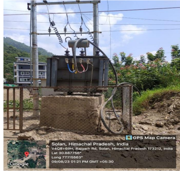
Figure3 Location after restoration
