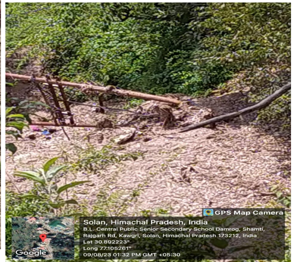
Figure 5 Fully washed out and found nearby place
