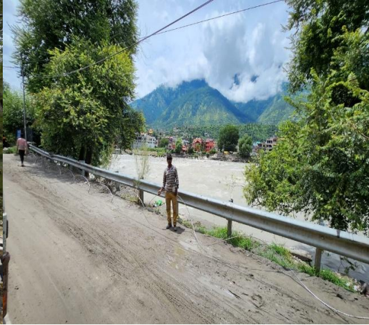
Figure 13 Restoration Work In Progress
