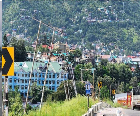
Figure 10. Poles Deformity of Structures Due to
