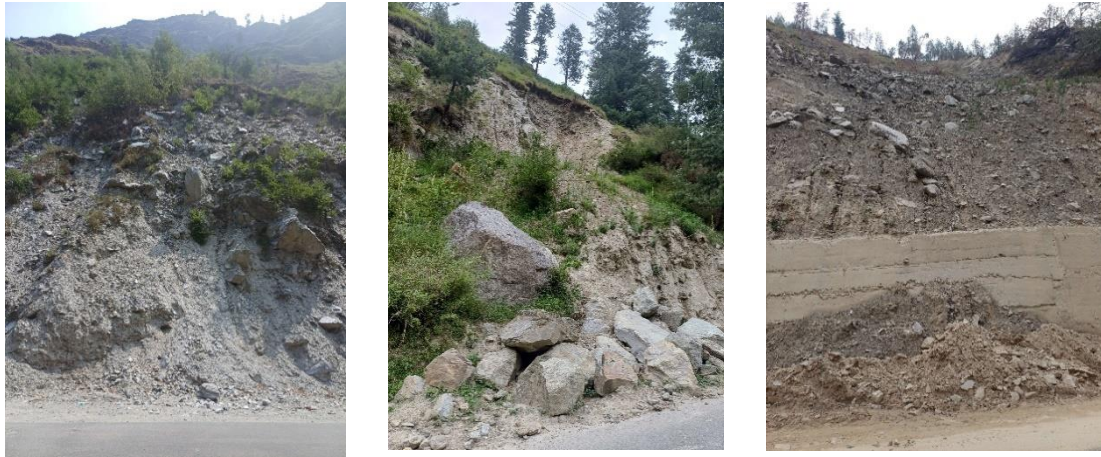
Figure 17: Landslides in Kullu district
