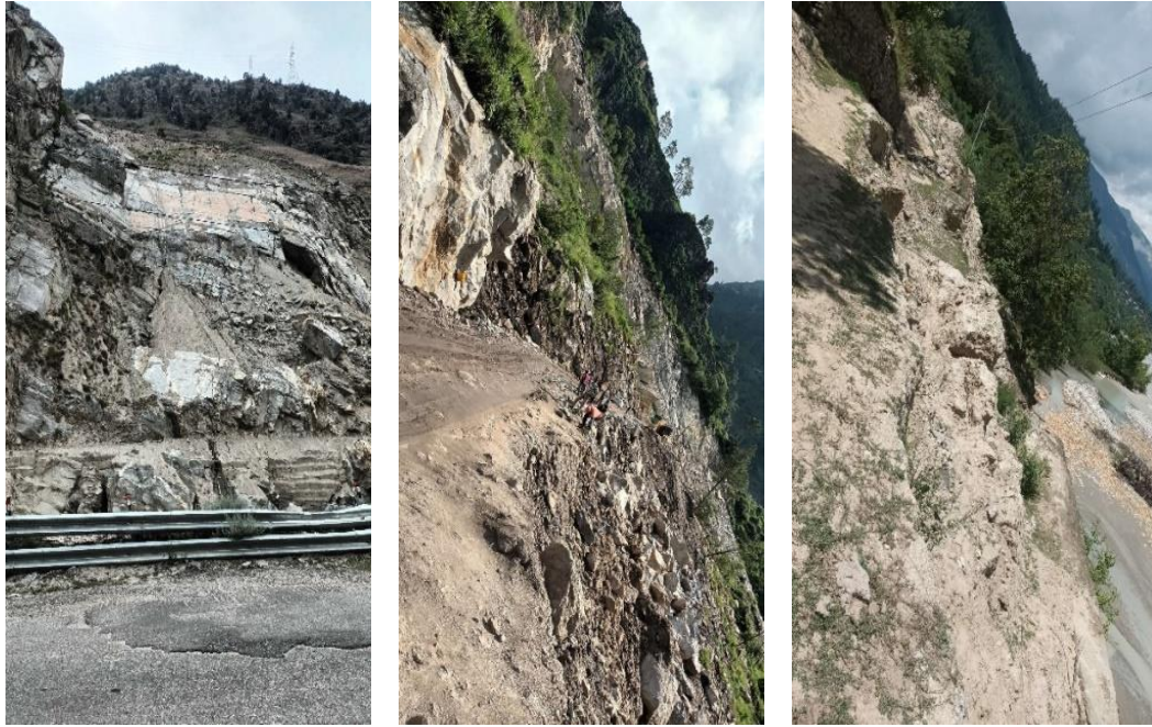
Figure 21: Landslides in Kinnaur district
