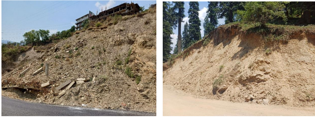
Figure 20: Landslides in Shimla district
