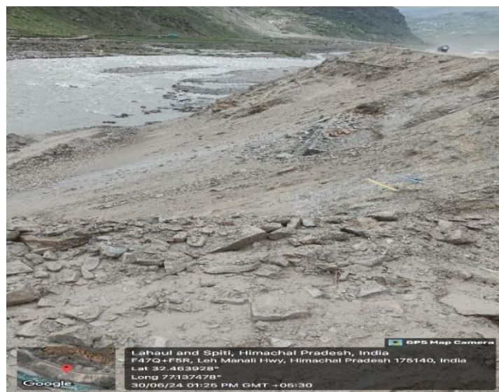
Figure 1 A Landslide damaged the NH-3 near Sissu, Lahaul & Spiti district
