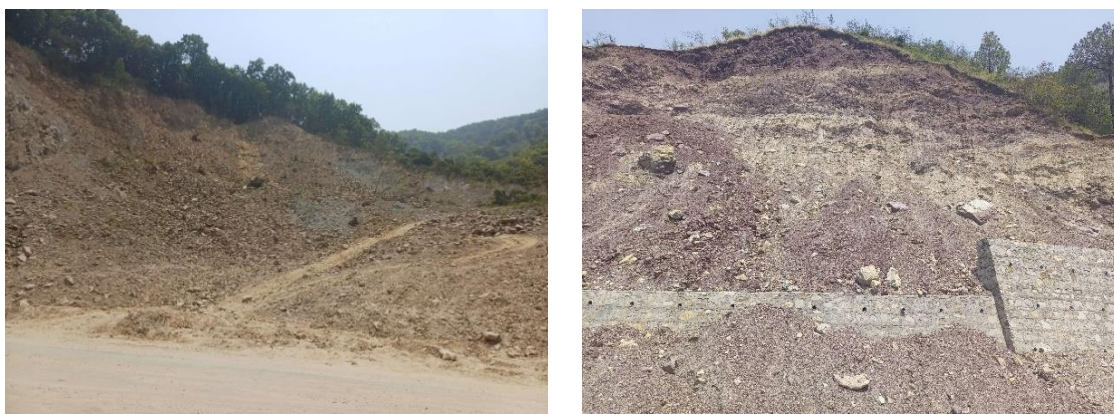
Figure 16: Landslides in Sirmour district
