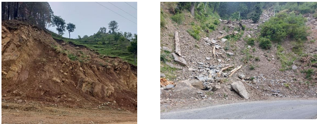
Figure 18: Landslides in Mandi district
