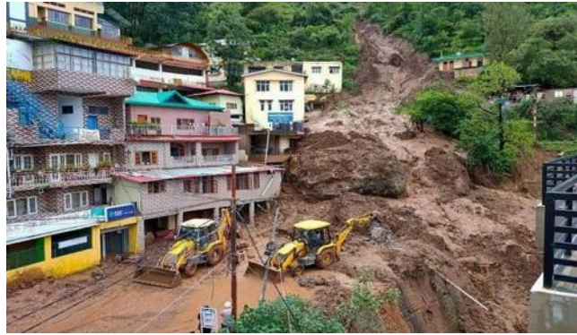
Figure 5: Landslide in Shamti in Solan district
