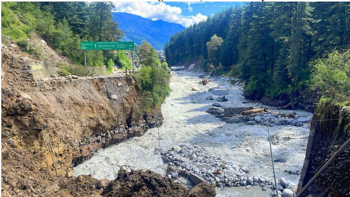
NH damaged in District Kullu
