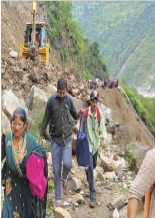
Pilgrims cross a damaged road stretch in Bharmour. PHOTO: MANI VERMA
