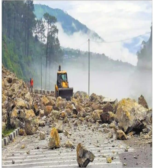
Restoration work underway on the Manal-Chandi highway in Mandi on Thursday. Natural disasters triggered by heavy rain in Himachal Pradesh have led to a loss of over ₹1,600 crore to the state.
