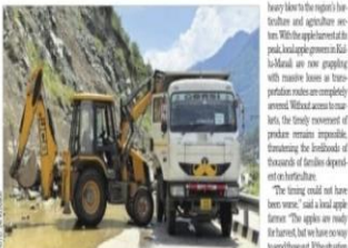
Restoration work underway on the Kirtarpur-Manali highway near Pang Deh in Mandi on Wednesday.
