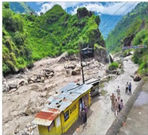
Flashfloods damaged a bridge and other infrastructure at Ganvi in Rampur of Shimla district.
