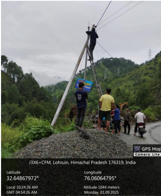
Electricity Supply being restored by HPSEBL
