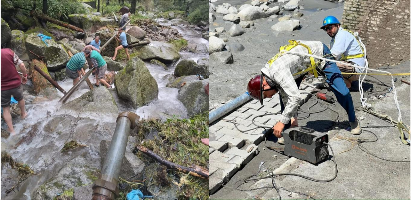
Restoration Work of WSS Schemes
