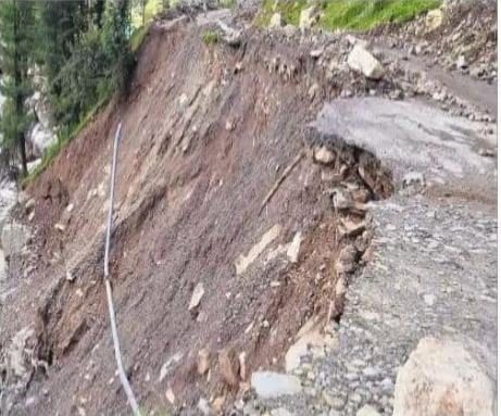
A road damaged due to a cloudburst in the Seraj valley of Mandi. PHOTO: JAI KUMAR
