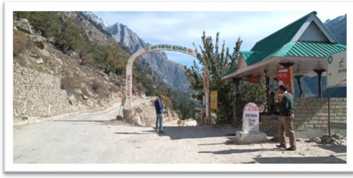
Visit to the Land Slide Site and Early Warning Gazette installation site at Batseri Village, Kinnaur on 4 th November
