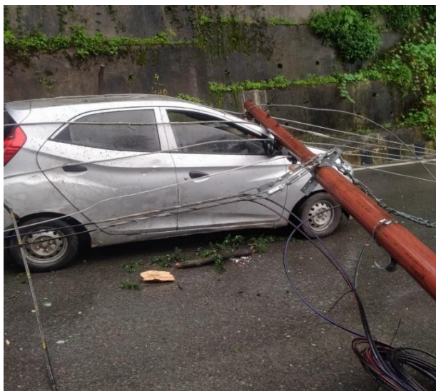
Figure 12 HT pole fallen on car due to heavy rainfall
