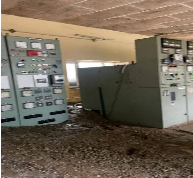
Figure 8 Mucked up deposition inside substation figure 7 Structural damage because of debris flow
