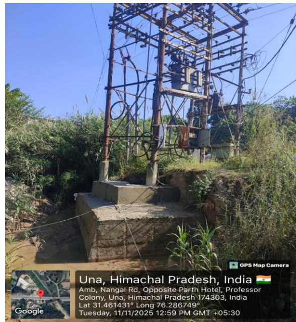
Figure 9 Post restoration work
