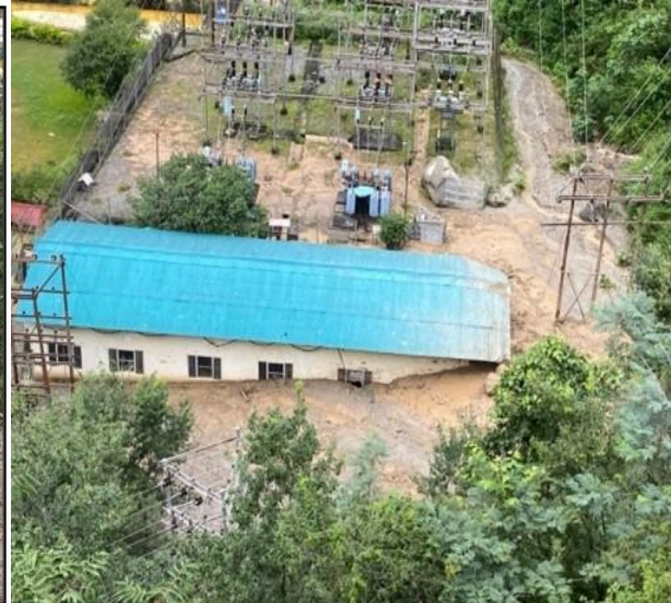
Figure 6 Muck Deposited in Substation
