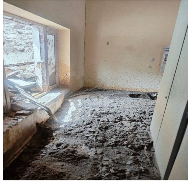
Figure 8 Mucked up deposition inside substation figure 7 Structural damage because of debris flow
