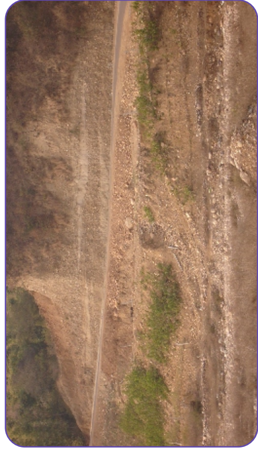
(Hedge Brush Layer : Bhawarna-Jaisinghpur Road, Chainage 25+600)
