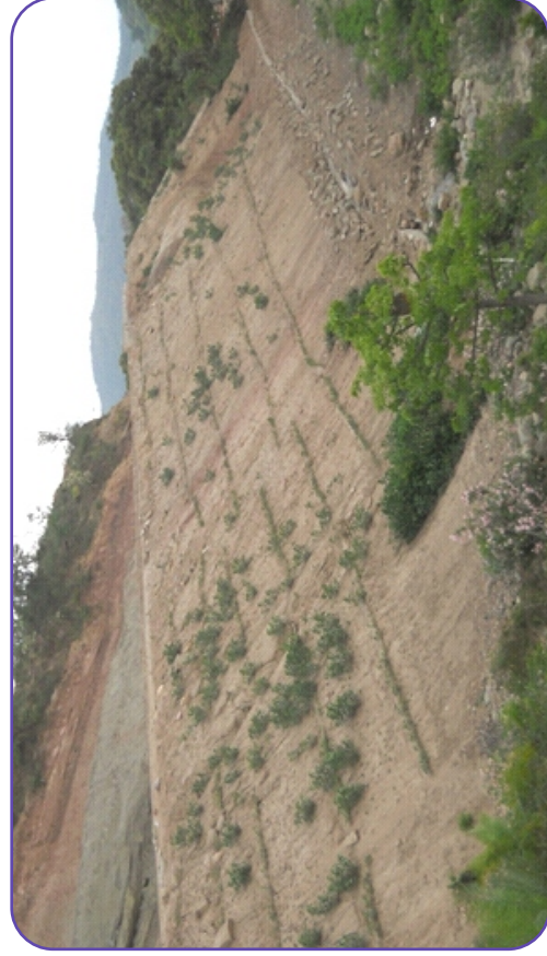
(Bamboo Crib Wall Formation : Barsar-Jahu Road, Chainage 67+200)
