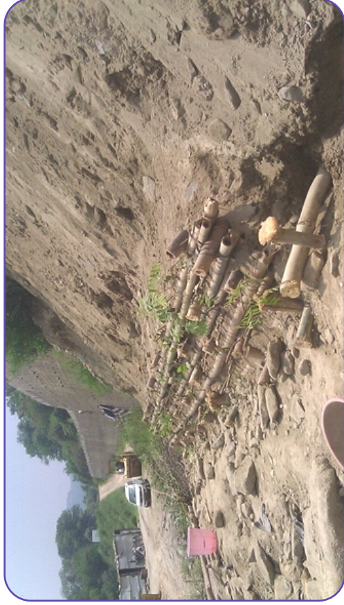
(Bamboo Crib Wall Formation : Barsar-Jahu Road, Chainage 67+200)
