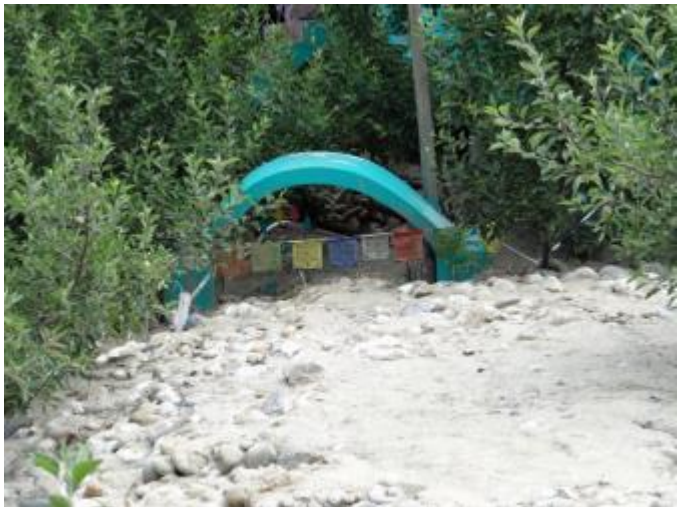
The entrance of a house completely blocked by mud and debris.
