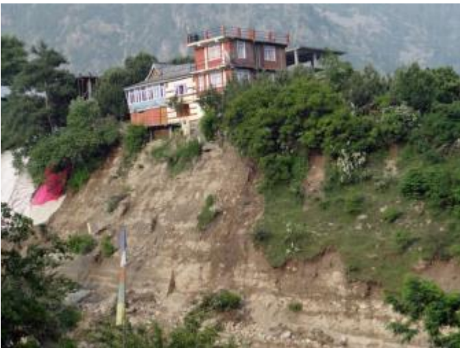
Some houses are on the verge of collapsing.
