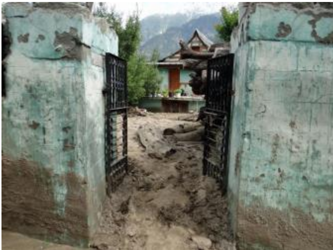
A glimpse of what flash flood and mud flow did to houses and property in Sangla valley.
