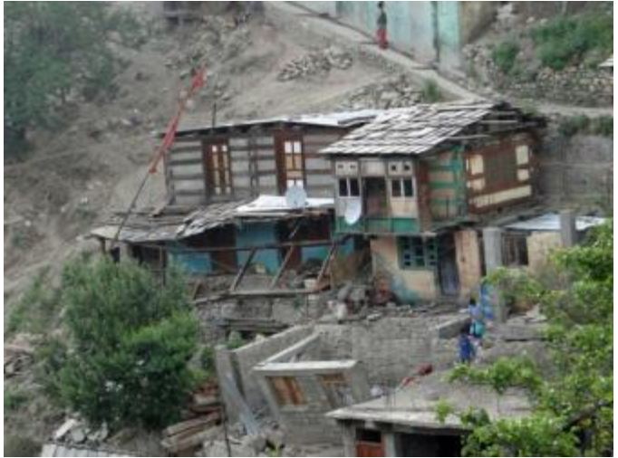
Sinking land also destroyed some houses in Sangla village.
