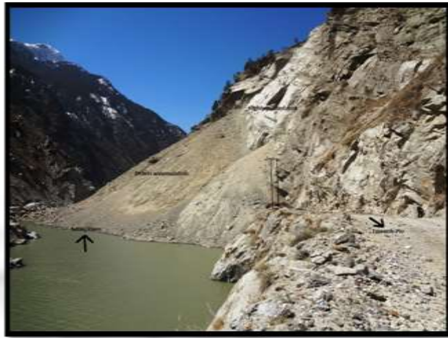
Fig 6 Debris accumulation on NH-22 and part of river Sutlej forming a landslide lake
