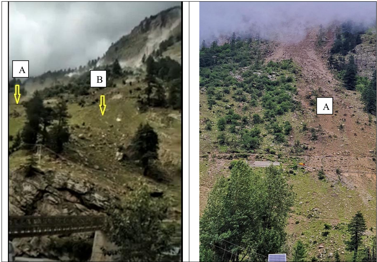
Fig.-7: The perspective view of trajectory of the rock fall before and after rock fall. The zone is with near absence of any vegetation, indicative of active natural processes along the slope
