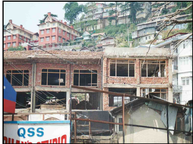
Common Structures .in Himachal Pradesh
