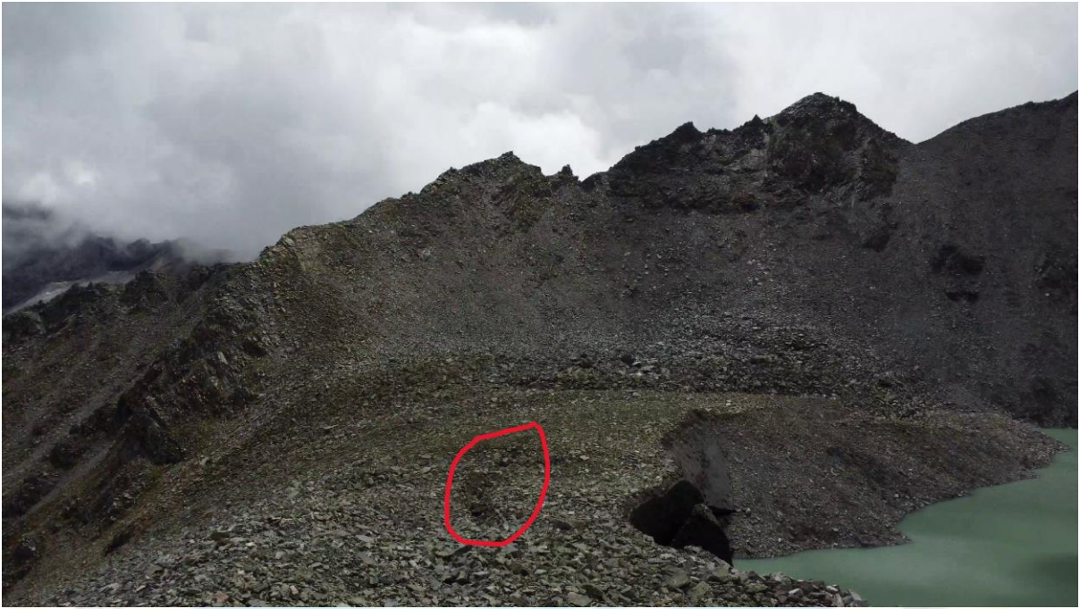
Fig 1: Crack seen on the moraine wall (Photo captured using drone)
